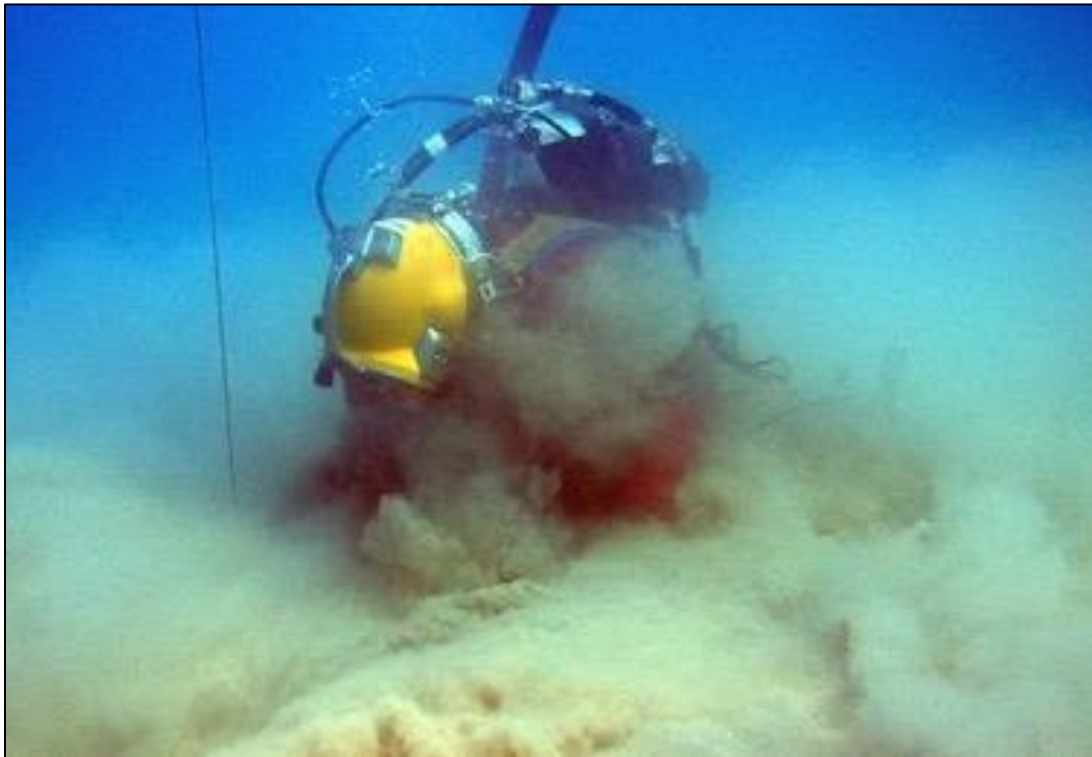
Figure 5-11 Surface supplied air (SSA) diver using a diver-operated dredge
