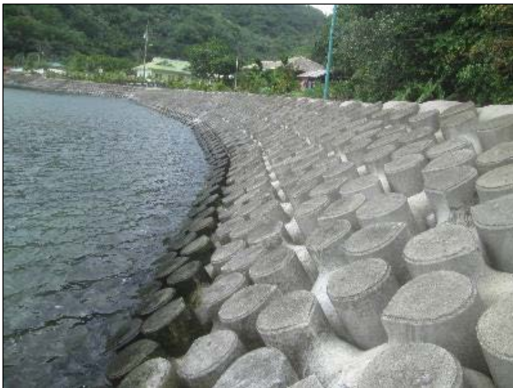
Figure 5-14 Tribar concrete armor units in American Samoa
