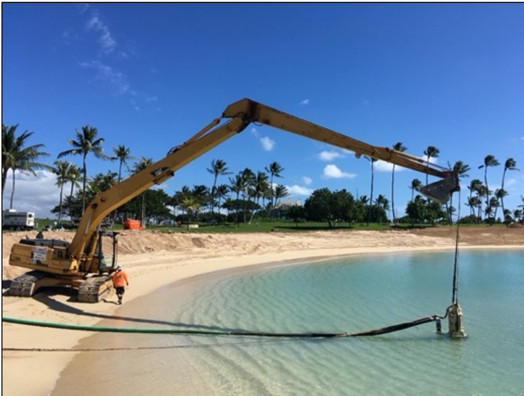
Figure 3-2 Sand pumping at Koʻolina, Oʻahu (2017)
