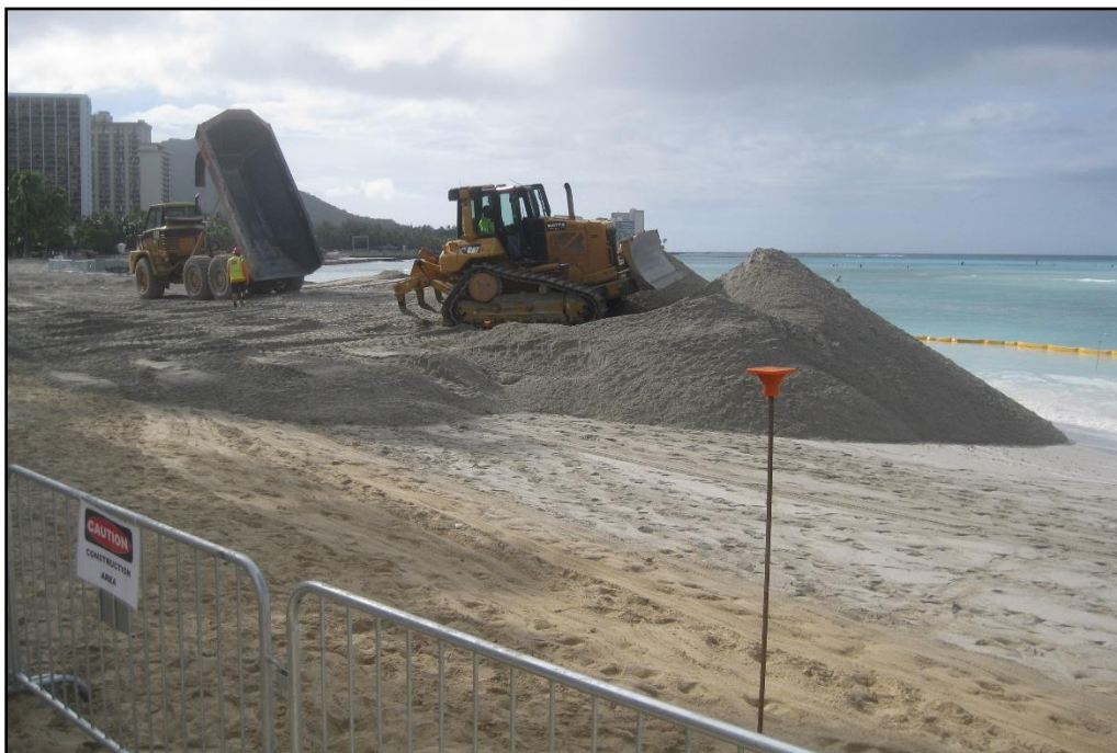
Figure 5-16 Sand placement, 2012 Waikiki Beach Maintenance Project.
