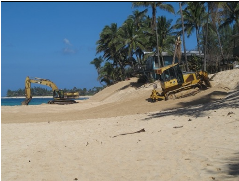
Figure 3-1 Sand pushing at Sunset Beach, O‘ahu (2014)
