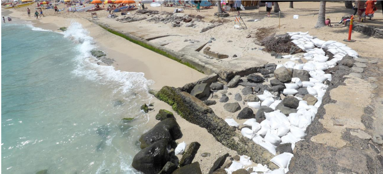
Photo 4. Concrete foundation exposed by erosion at the Diamond Head end of the Royal Hawaiian sector, May 17, 2017. Photo courtesy of Matt Bell.
