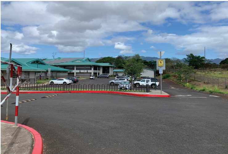
3. View of Waikele Elementary School from the vehicle entrance on Kukula Street, looking west toward the Project Site.
