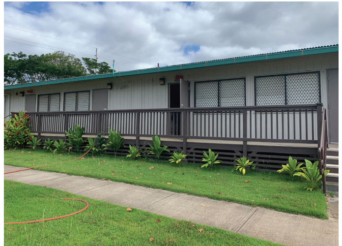
4. View of a portable classroom building on the Project Site, looking northwest.
