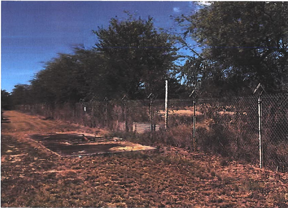
Photo 1: Original 'Ewa Field base fence, north of Roosevelt Avenue.
