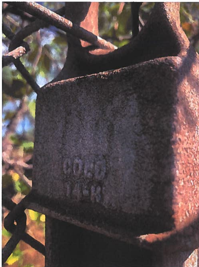
Photo 5. Identifier "COLO 14-H" on fence topper likely denotes the Colorado Chain Link Fence Company as the manufacturer, with the "H" referring to the post type.
