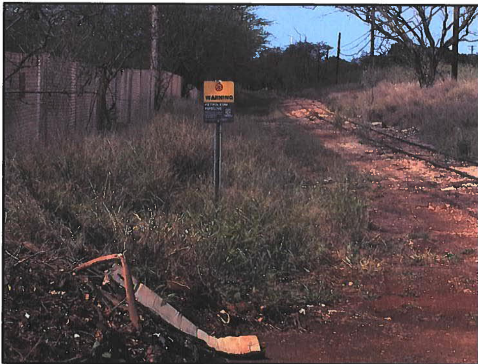
Photograph 8. Railroad Crossing #2, view of OR&L ROW looking west from Malio Street.
