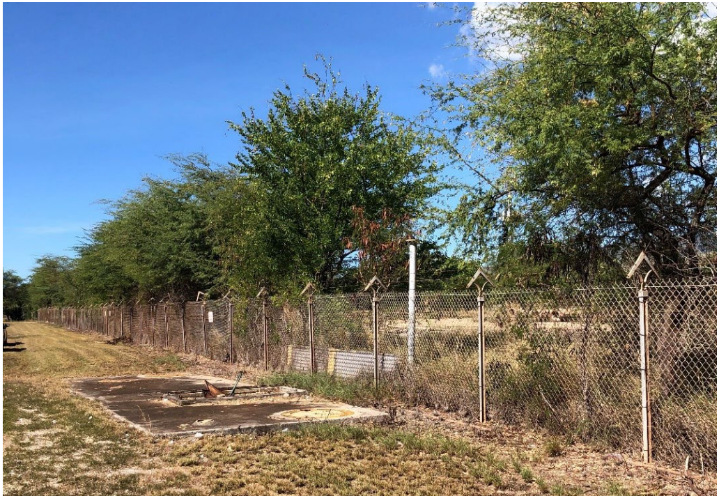
Figure 2-9. 'Ewa Field Base Fence, North of Roosevelt Avenue
