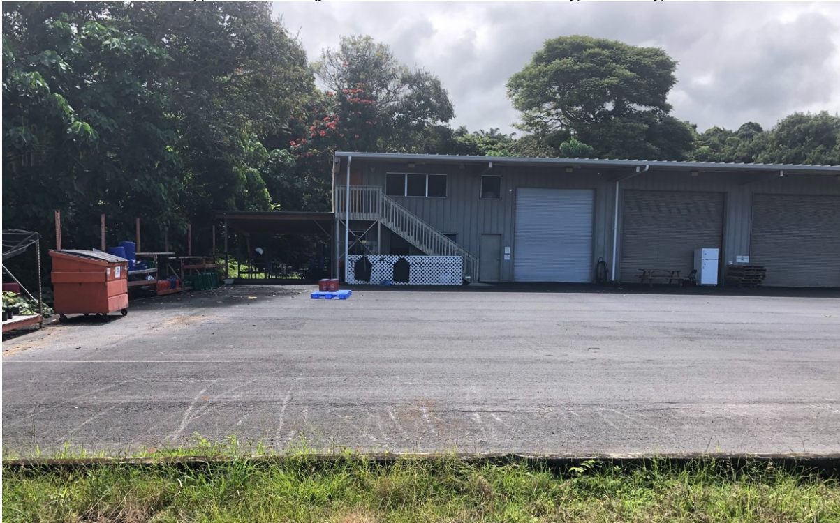
Figure 2. Project Site Photos. a. Existing Building
