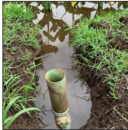
Above: Closed outflow connecting lo'i and 'auwai. Source: Hui, 2020
