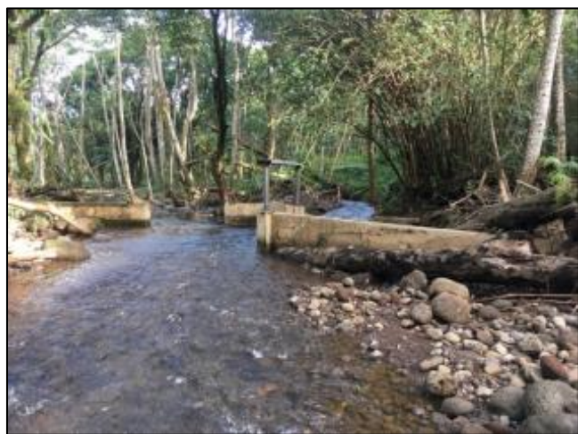
Po‘owai “Lower” Diversion – Upstream view of “lower” diversion on tributary of stream.
