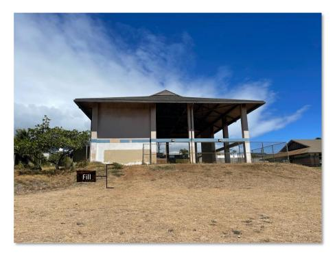
Figure 2-5. Overall view of play court structure showing the pad of fill underlying the play court foundation view to northwest.
