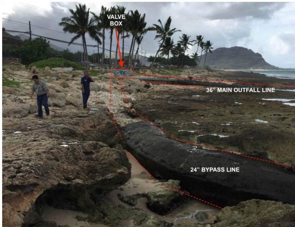
Figure 1-2. Outfall bypass line and junction/valve box.
