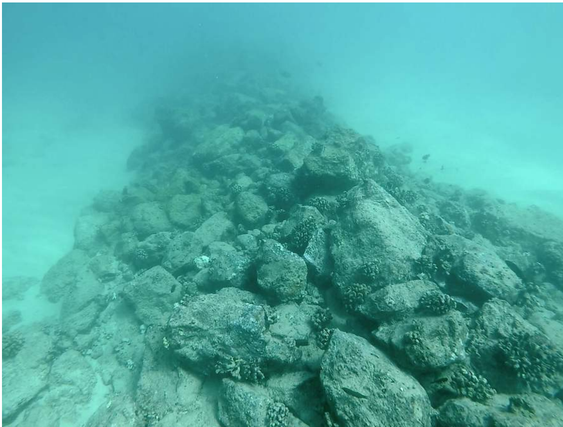
Figure 4-27. Typical ballast pile condition, near station 10+00
