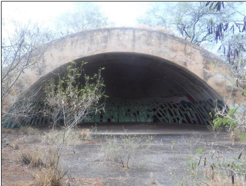
Figure 48. SIHP 50-80-12-XXXXX (T-02), Feature 46 revetment (view to southeast).
