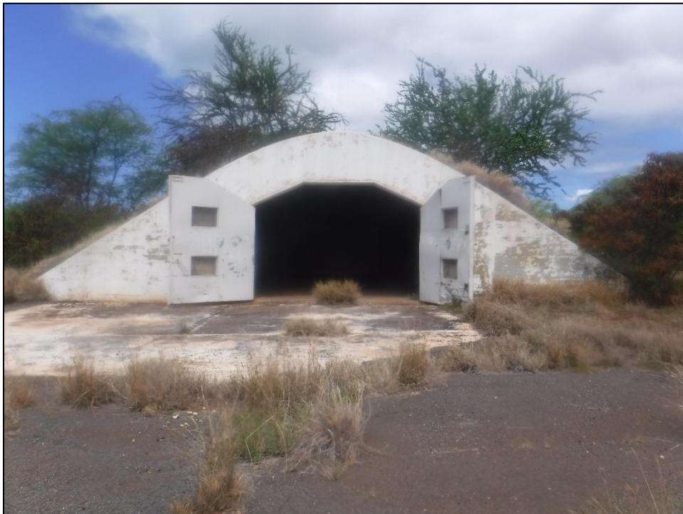
Figure 11. SIHP 50-80-12-XXXXX (T-01), east side of Feature 6 magazine (view to west).
