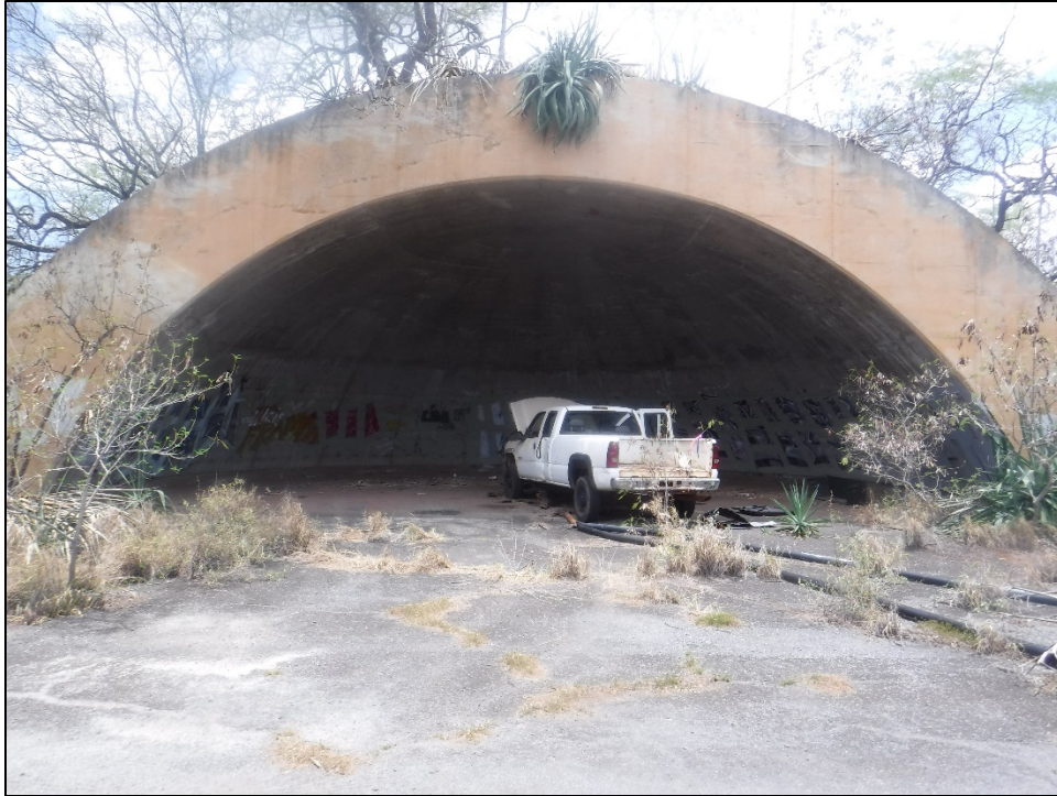
Figure 21. SIHP 50-80-12-XXXXX (T-02), Feature 9 revetment (view to west).
