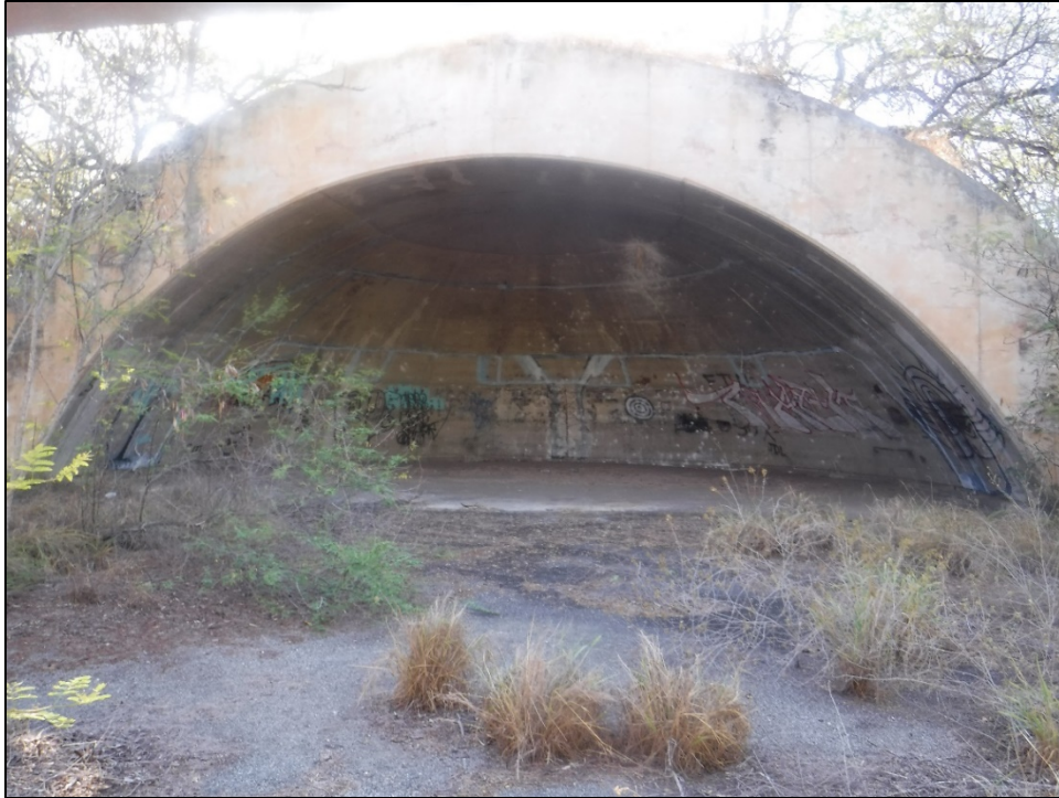
Figure 45. SIHP 50-80-12-XXXXX (T-02), Feature 43 revetment (view to east).
