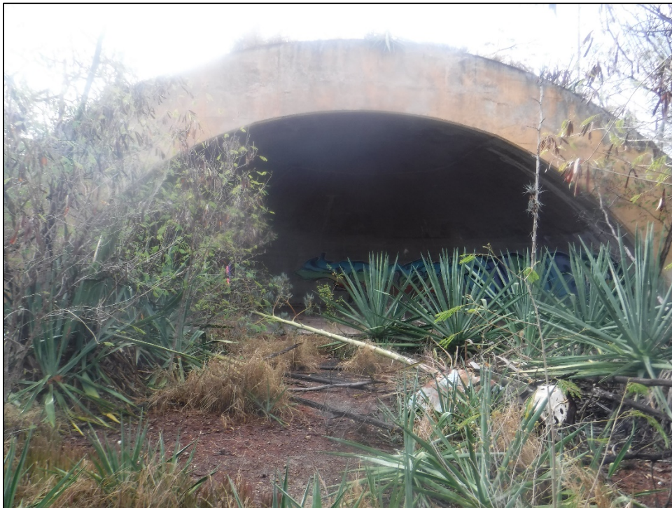
Figure 20. SIHP 50-80-12-XXXXX (T-02), Feature 7 revetment (view to east).
