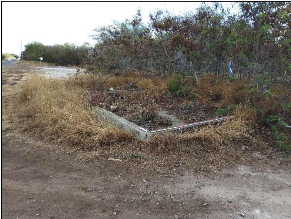
Figure 263. SIHP 50-80-12-XXXXX (T-09) Feature 6 concrete building foundation (view to northeast).
