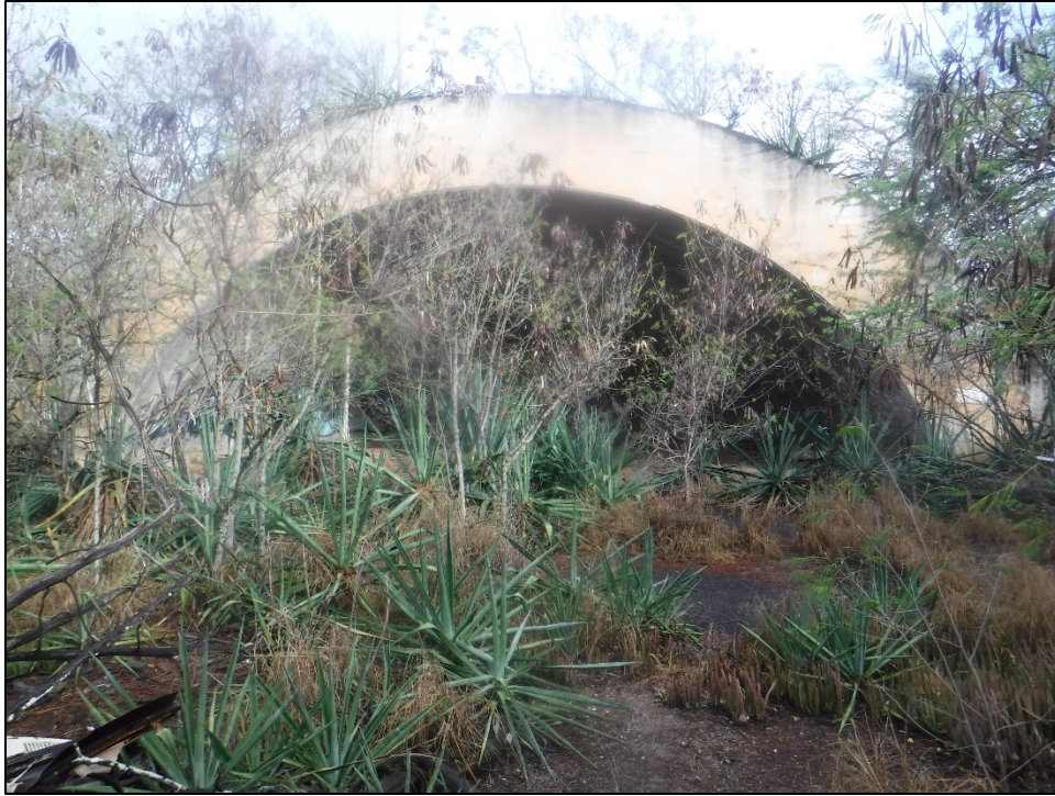
Figure 19. SIHP 50-80-12-XXXXX (T-02), Feature 6 revetment (view to west).
