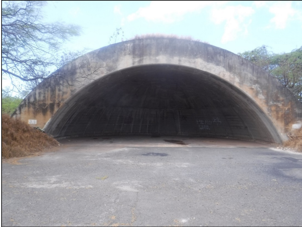
Figure 31. SIHP 50-80-12-XXXXX (T-02), Feature 25 revetment (view to south).
