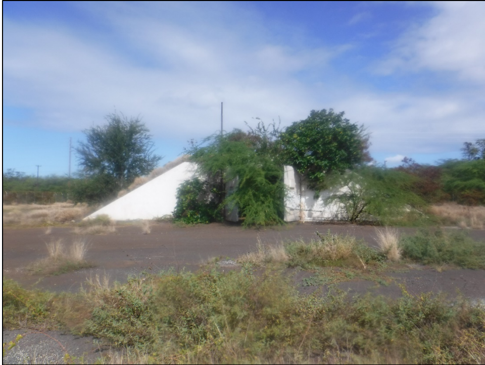
Figure 8. SIHP 50-80-12-XXXXXX (T-01), east side of Feature 4 magazine (view to west).
