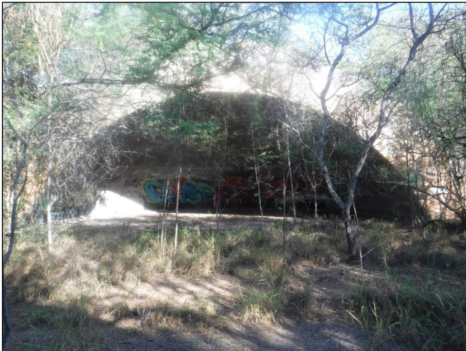
Figure 50. SIHP 50-80-12-XXXXX (T-02), Feature 50 revetment (view to west).
