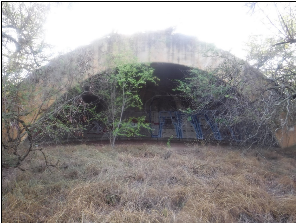
Figure 38. SIHP 50-80-12-XXXXX (T-02), Feature 32 revetment (view to east).
