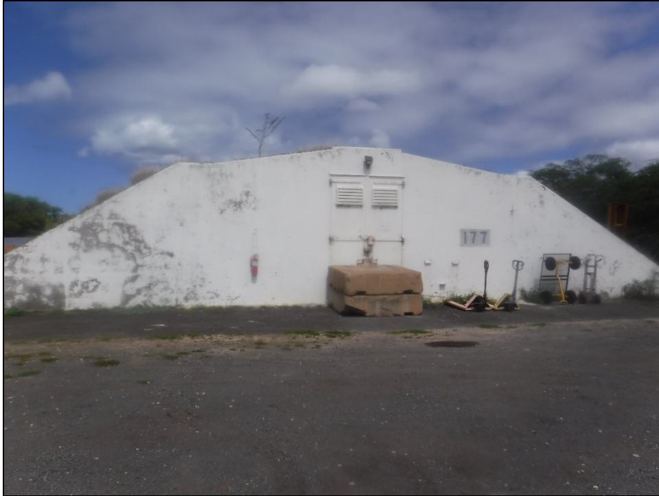
Figure 4. SIHP 50-80-12-XXXXX (T-01), east side of Feature 2 magazine (view to west).
