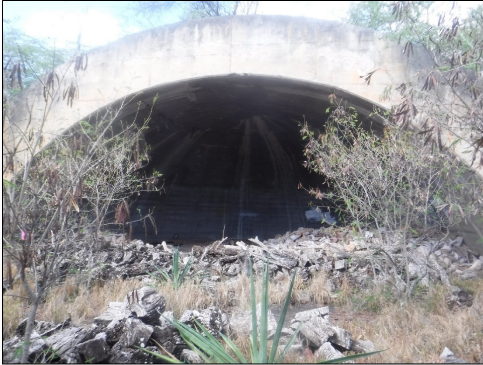
Figure 37. SIHP 50-80-12-XXXXX (T-02), Feature 31 revetment (view to southwest).
