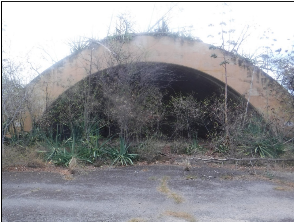
Figure 22. SIHP 50-80-12-XXXXX (T-02), Feature 10 revetment (view to east).
