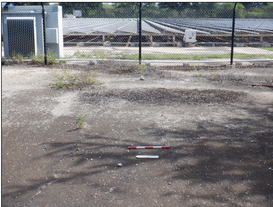
Figure 250. Site 50-80-12-XXXXX (T-08), Feature 1, showing portion of 1942 apron on eastern boundary of project area with the Kalaeloa Renewable Energy Park (KREP) facility in background (view to east).
