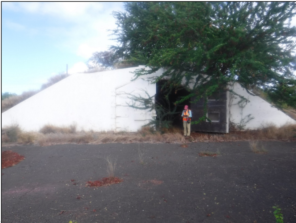
Figure 9. SIHP 50-80-12-XXXXXX (T-01), east side of Feature 5 magazine (view to west).
