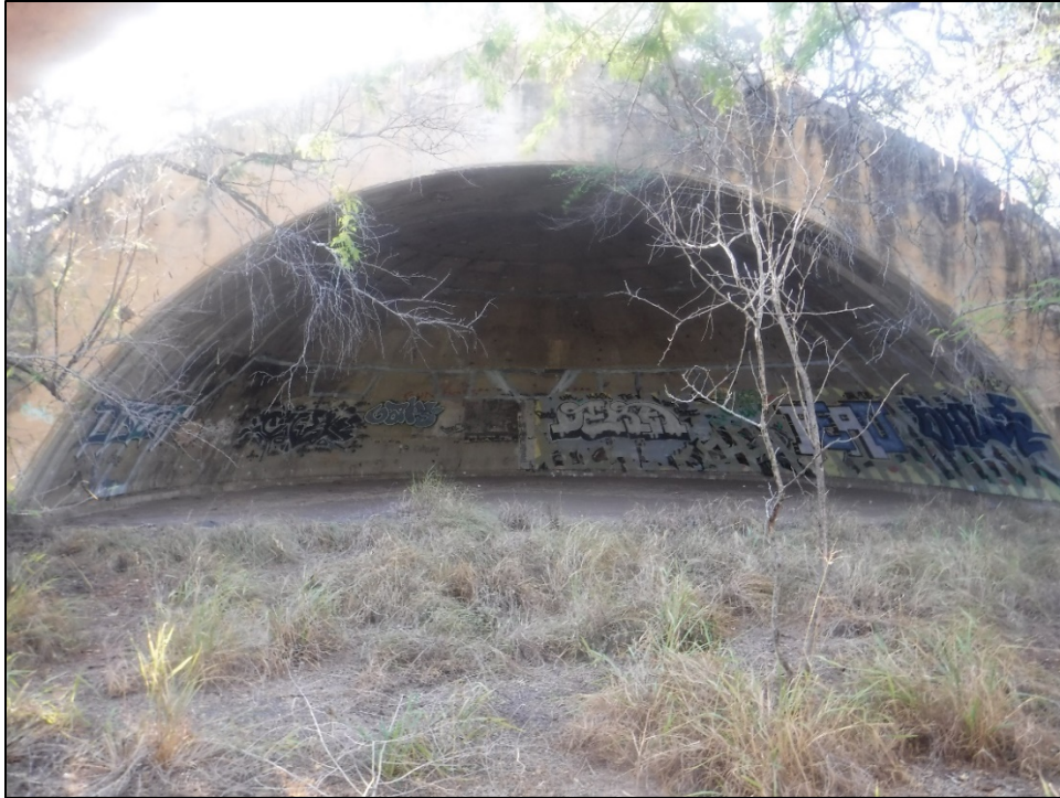
Figure 51. SIHP 50-80-12-XXXXX (T-02), Feature 51 revetment (view to east).
