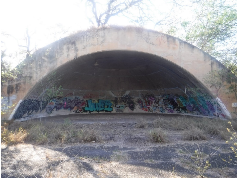
Figure 43. SIHP 50-80-12-XXXXX (T-02), Feature 41 revetment (view to east).
