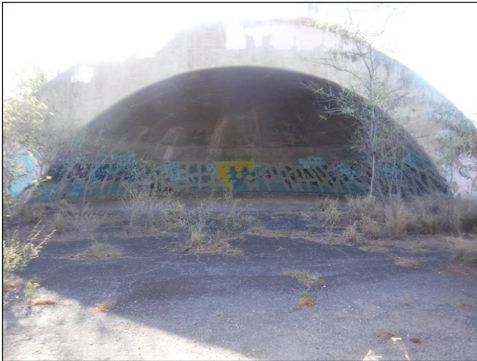
Figure 18. SIHP 50-80-12-XXXXX (T-02), Feature 4 revetment (view to east).
