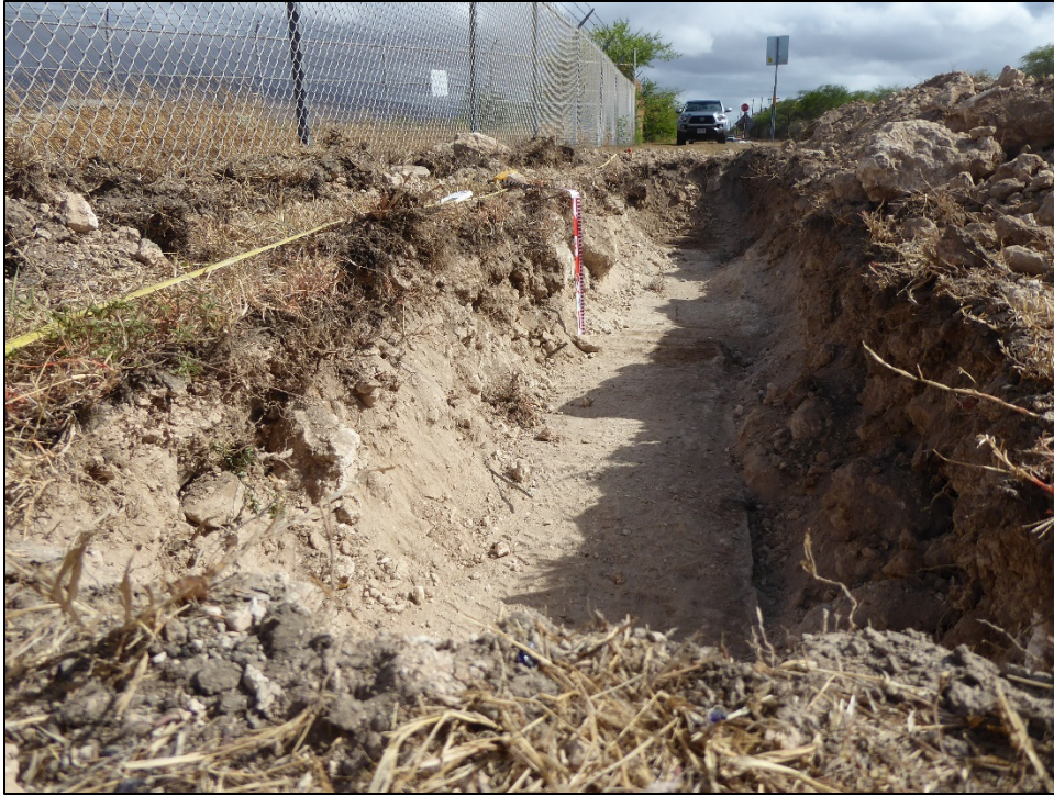
Figure 5. Trench 2 west wall profile, oblique view (view to north).
