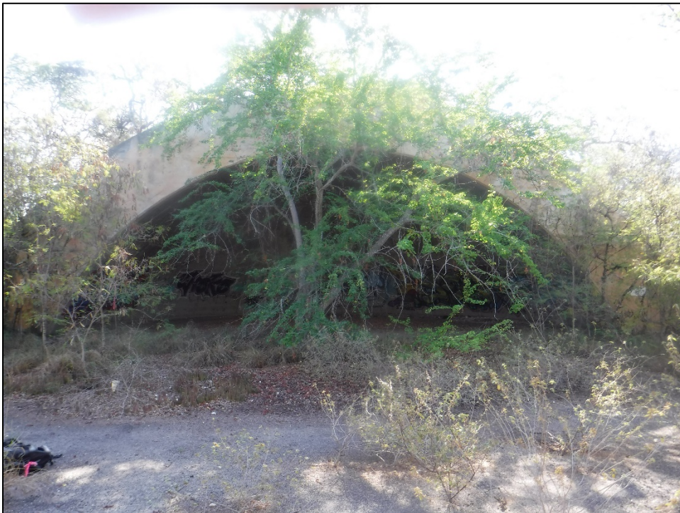
Figure 16. SIHP 50-80-12-XXXXX (T-02), Feature 2 revetment (view to east).
