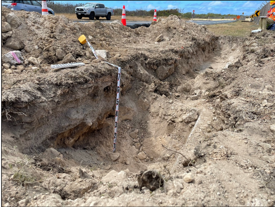
Figure 10. Trench 3, east wall profile, oblique view (view to southeast).
