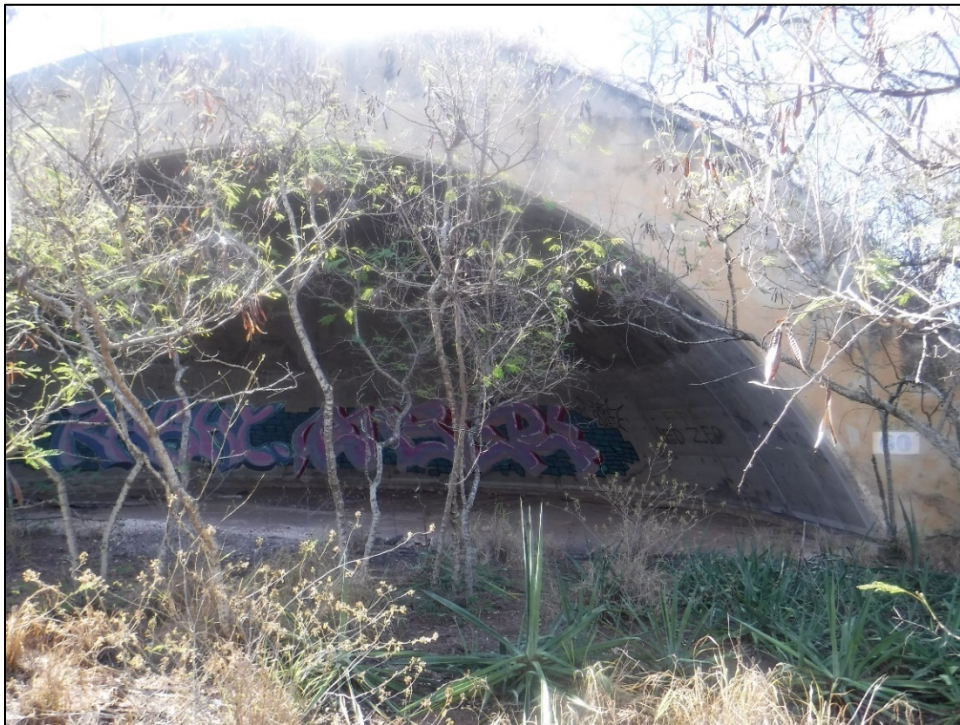
Figure 24. SIHP 50-80-12-XXXXX (T-02), Feature 12 revetment (view to southeast).
