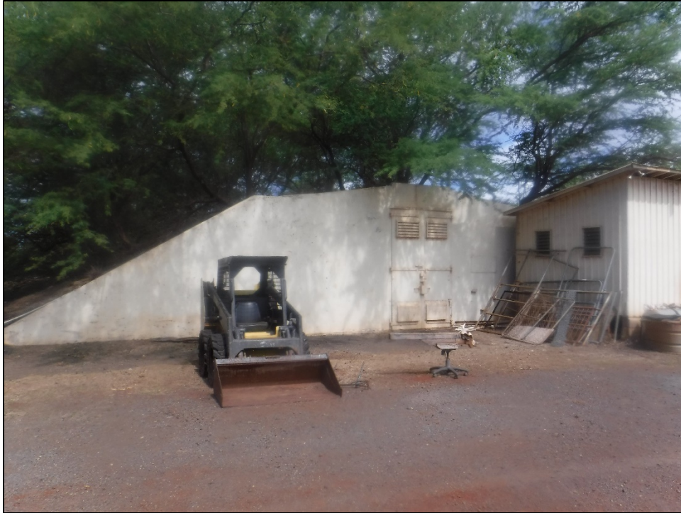
Figure 2. SIHP 50-80-12-XXXXX (T-01), east side of Feature 1 magazine (view to northwest).
