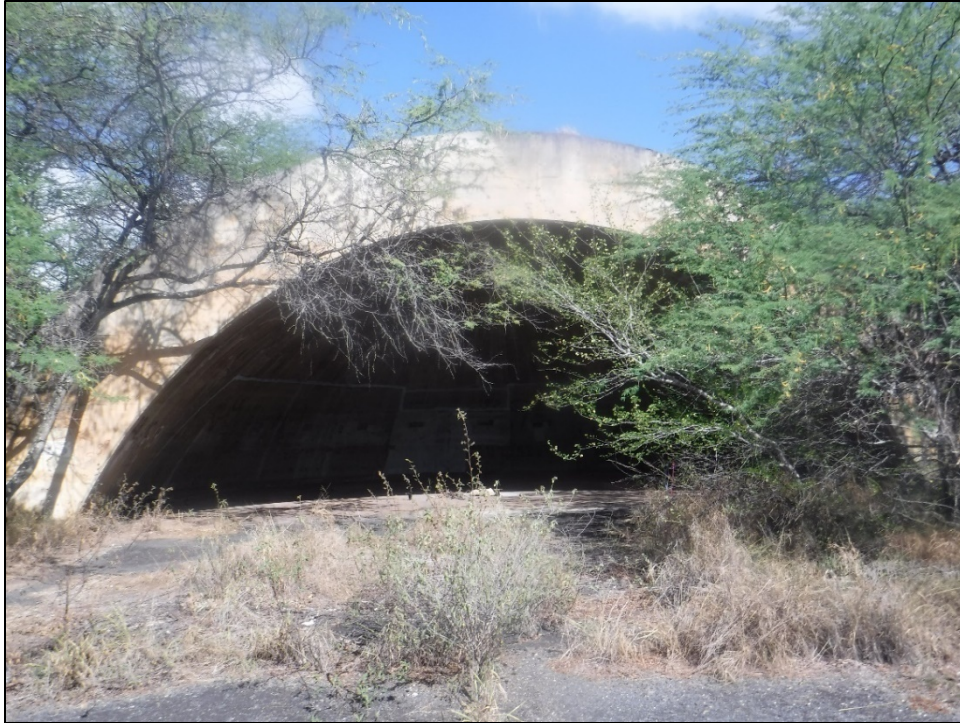
Figure 35. SIHP 50-80-12-XXXXX (T-02), Feature 29 revetment (view to west).
