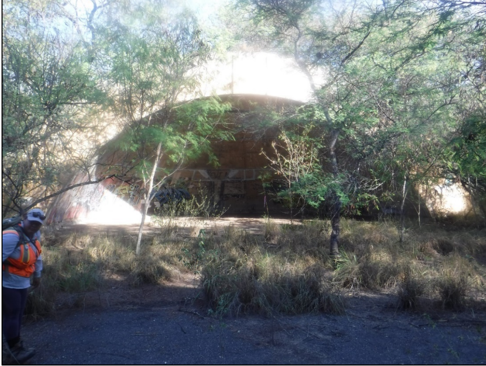
Figure 53. SIHP 50-80-12-XXXXX (T-02), Feature 53 revetment (view to west).
