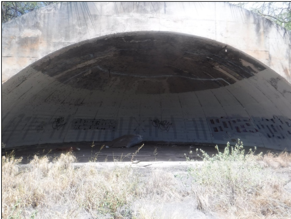
Figure 40. SIHP 50-80-12-XXXXX (T-02), Feature 38 revetment (view to southwest).
