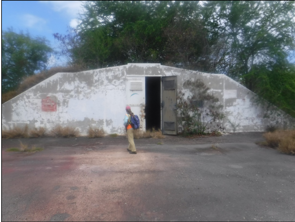
Figure 6. SIHP 50-80-12-XXXXX (T-01), east side of Feature 3 magazine (view to west).
