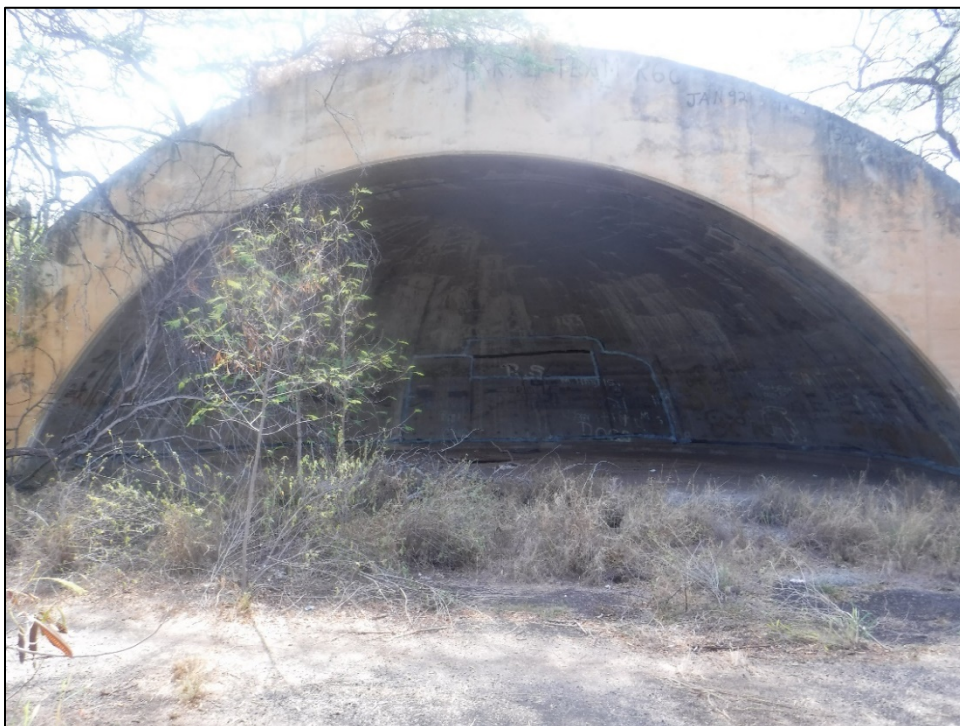
Figure 34. SIHP 50-80-12-XXXXX (T-02), Feature 28 revetment (view to east).
