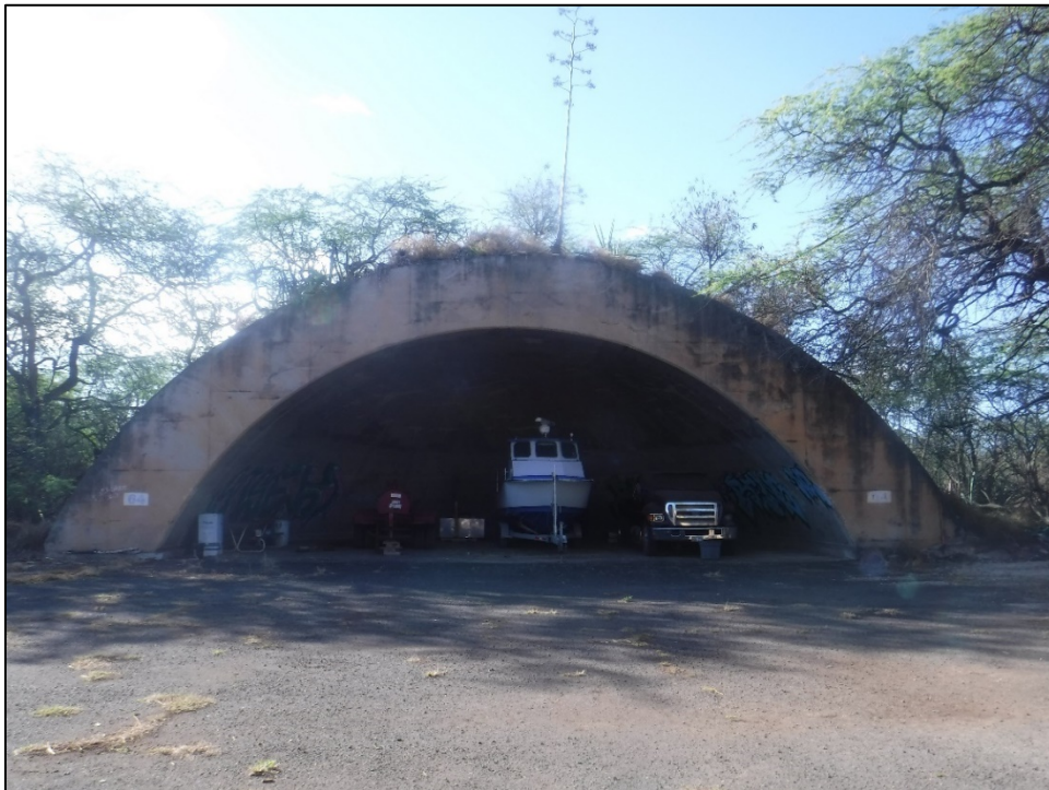
Figure 26. SIHP 50-80-12-XXXXX (T-02), Feature 14 revetment (view to southeast).
