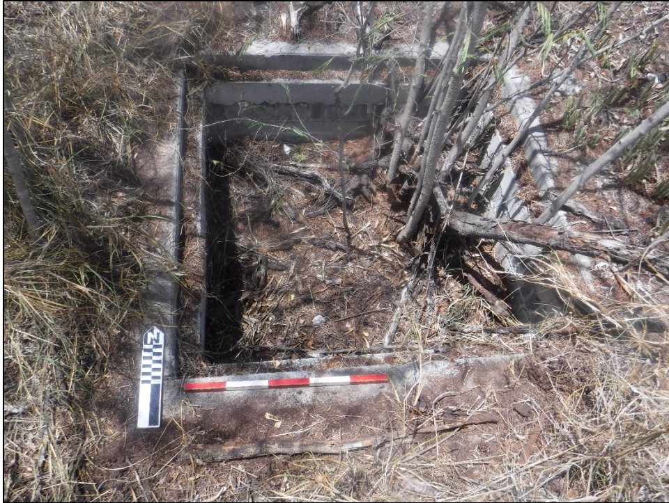
Figure 254. SIHP 50-80-12-XXXXX (T-08), Feature 3 concrete box (view to north).
