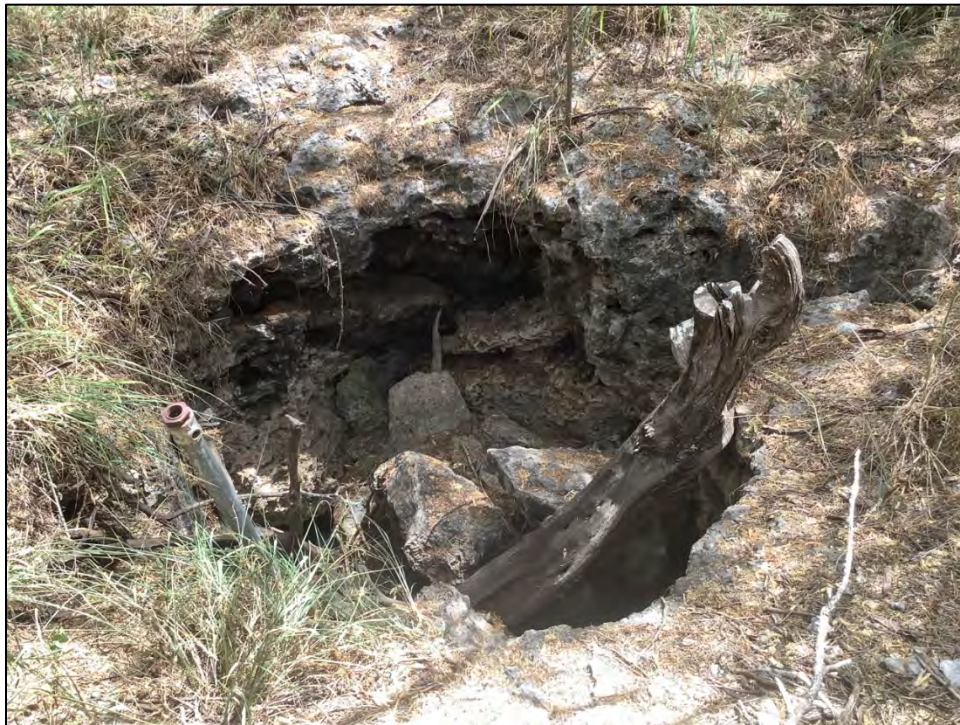
Photo 19. Sinkhole observed within Area 1x of the Study Area. Numerous sinkholes of various sizes occur throughout the entire Study Area. Location: 21.316323, -158.049555. June 3, 2020.
