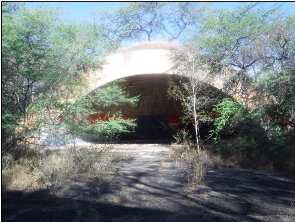
Figure 44. SIHP 50-80-12-XXXXX (T-02), Feature 42 revetment (view to west-northwest).
