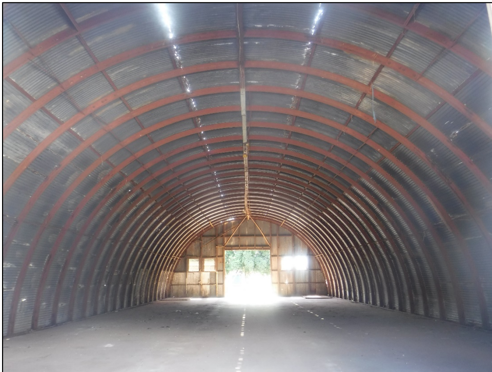
Figure 61. SIHP 50-80-12-XXXXX (T-02), Feature 20 building interior (view to east).
