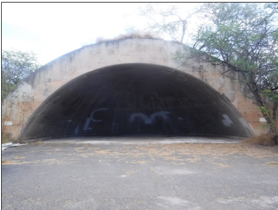
Figure 30. SIHP 50-80-12-XXXXX (T-02), Feature 24 revetment (view to north).
