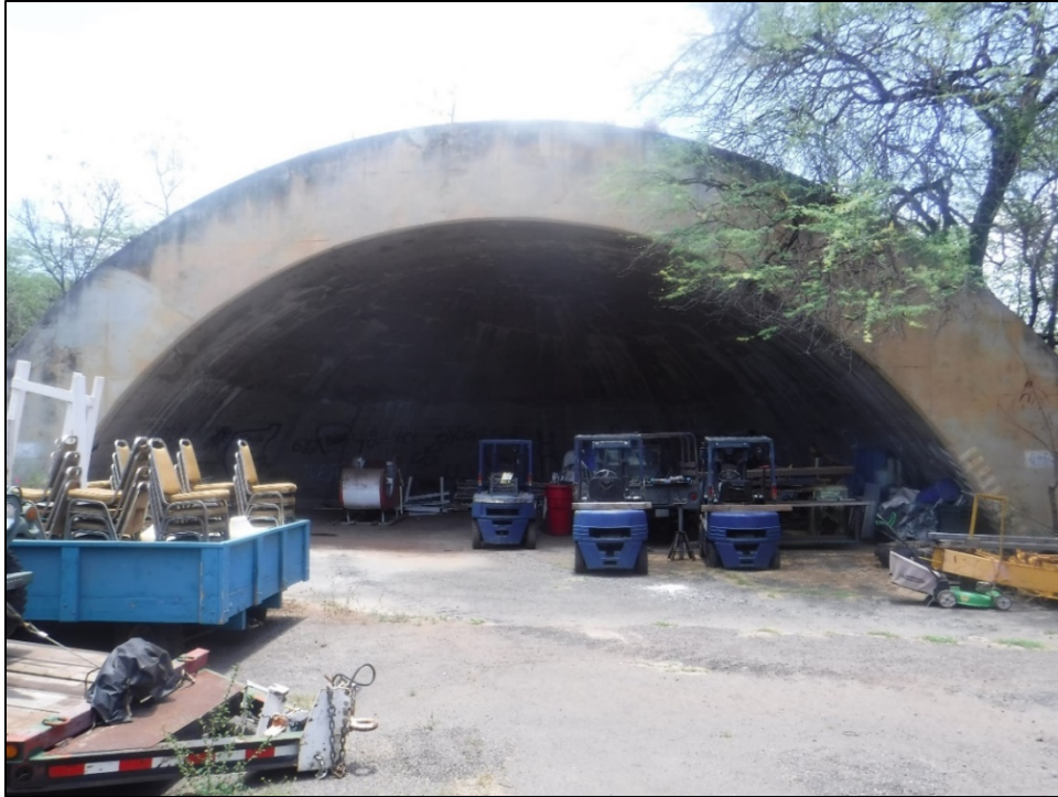
Figure 27. SIHP 50-80-12-XXXXX (T-02), Feature 15 revetment (view to west).
