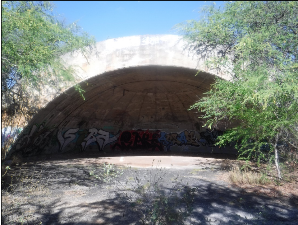
Figure 15. SIHP 50-80-12-XXXXX (T-02), Feature 1 revetment (view to west).
