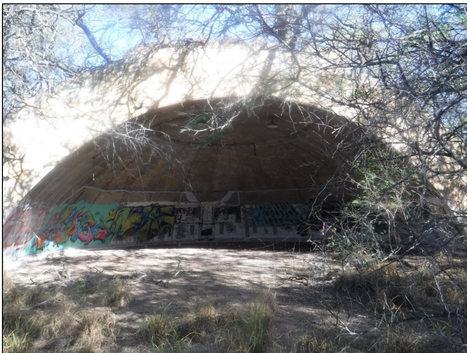
Figure 42. SIHP 50-80-12-XXXXX (T-02), Feature 40 revetment (view to west).
