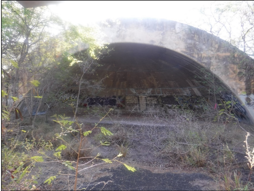
Figure 49. SIHP 50-80-12-XXXXX (T-02), Feature 49 revetment (view to east).
