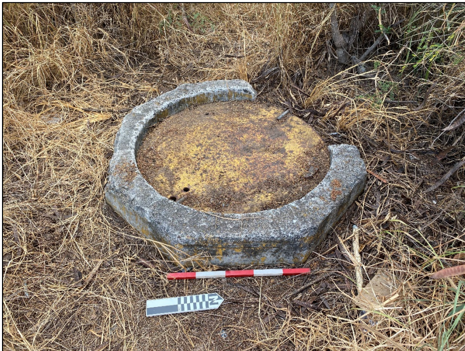
Figure 258. SIHP 50-80-12-XXXXX (T-09) Feature 2 concrete structure (view to west).
