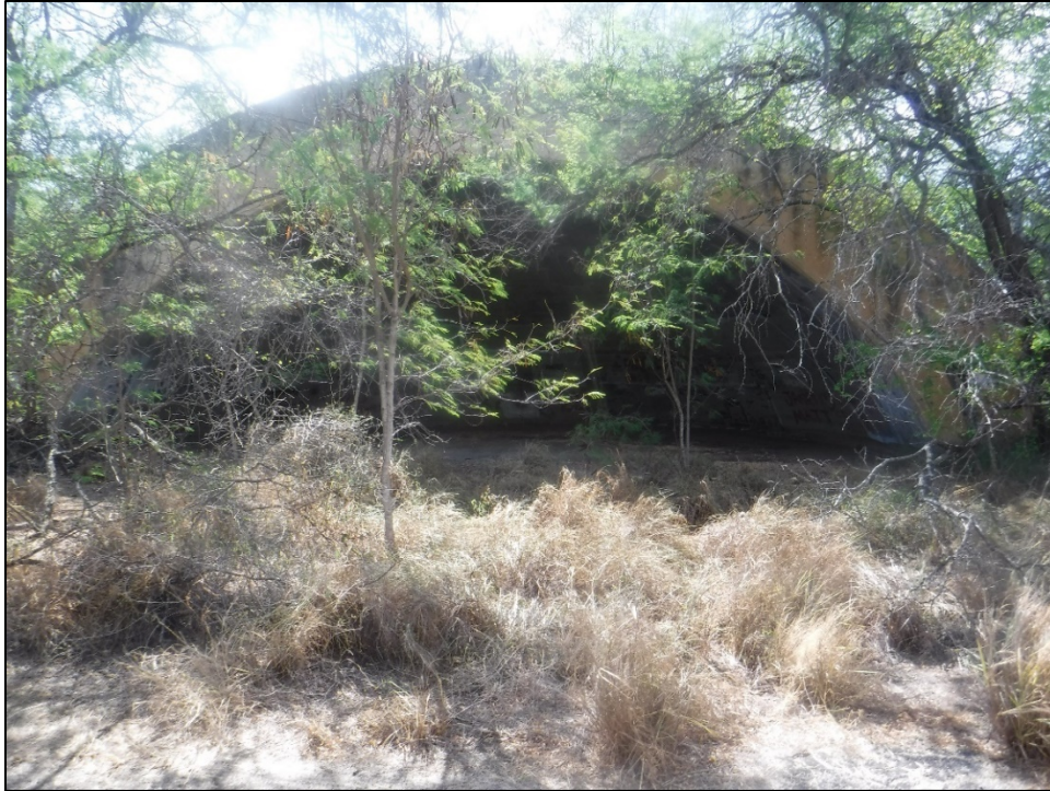
Figure 33. SIHP 50-80-12-XXXXX (T-02), Feature 27 revetment (view to east).
