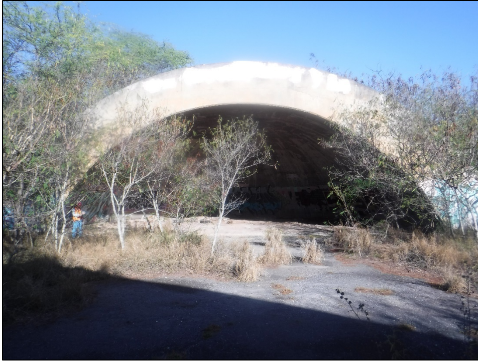
Figure 17. SIHP 50-80-12-XXXXX (T-02), Feature 3 revetment (view to west).
