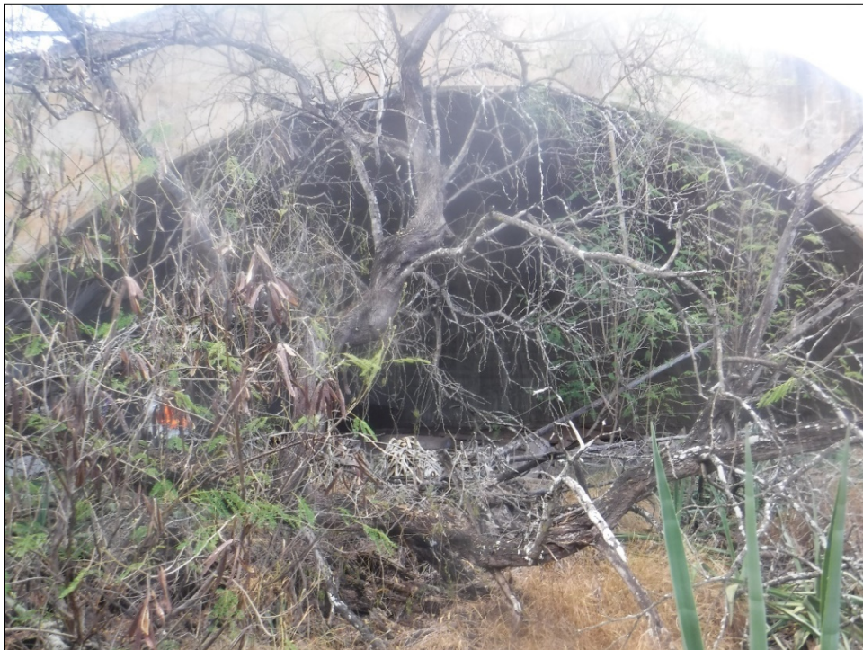
Figure 36. SIHP 50-80-12-XXXXX (T-02), Feature 30 revetment (view to northeast).
