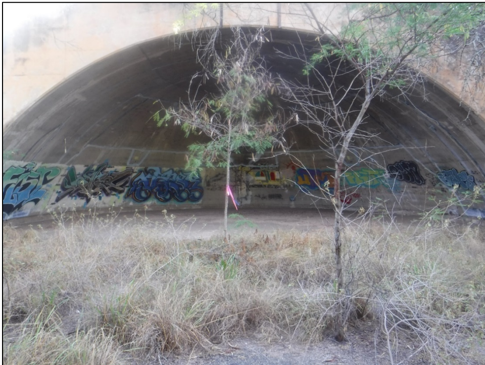
Figure 52. SIHP 50-80-12-XXXXX (T-02), Feature 52 revetment (view to east).
