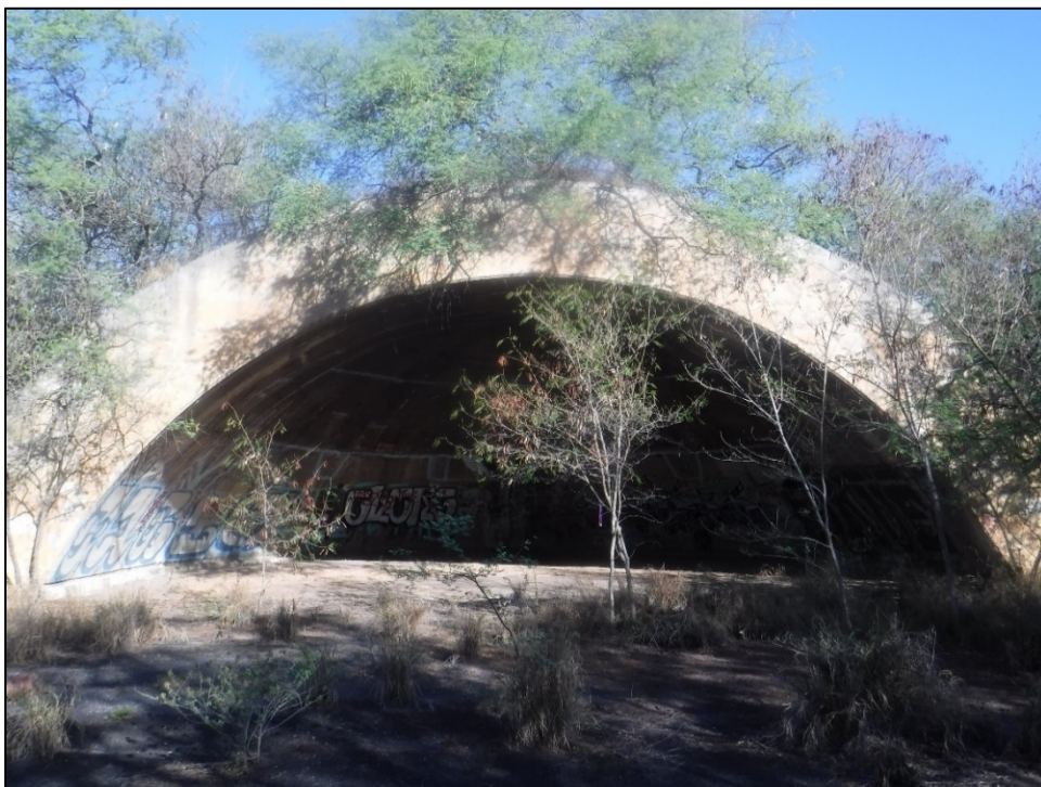
Figure 46. SIHP 50-80-12-XXXXX (T-02), Feature 44 revetment (view to west).
