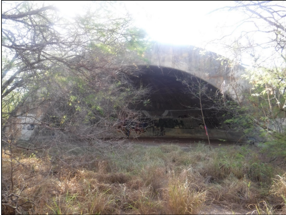
Figure 41. SIHP 50-80-12-XXXXX (T-02), Feature 39 revetment (view to east).
