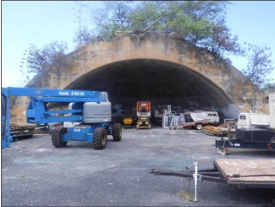
Figure 39. SIHP 50-80-12-XXXXX (T-02), Feature 33 revetment (view to south).
