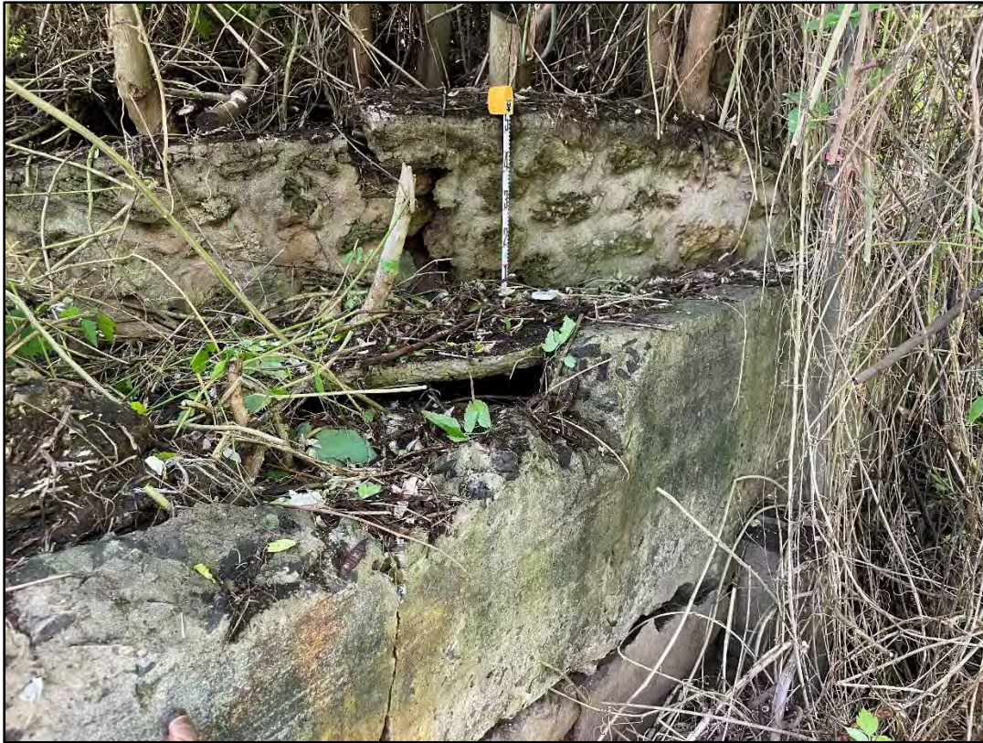
Figure 43. Photo M: Retaining wall(s) on south side of spillway, the upper wall is believed to be older and relate to the original construction of the reservoir and the lower wall is believed to relate to renovations ca. 1950, view to south
