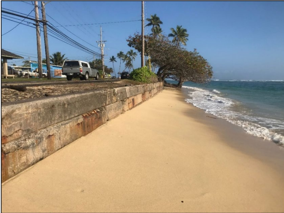
Figure 3-5. Concrete block seawall immediately south of project site
