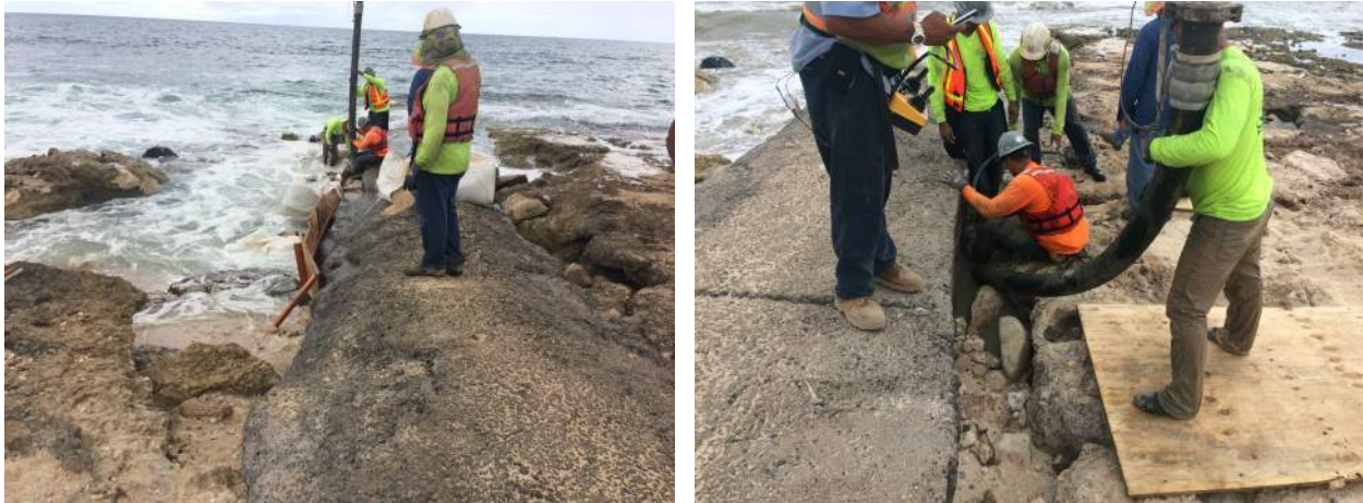
Figure 5-15. Concrete placement within formworks via boom truck ( left ); concrete pumped into gap ( right )
