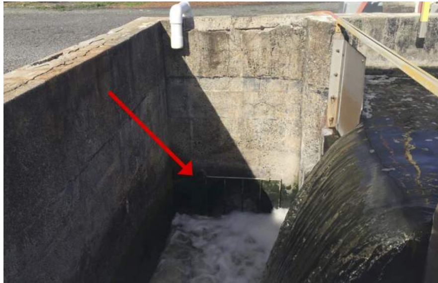
Figure 5-2. Tracer dye injection location, outfall entrance gate (red arrow)
