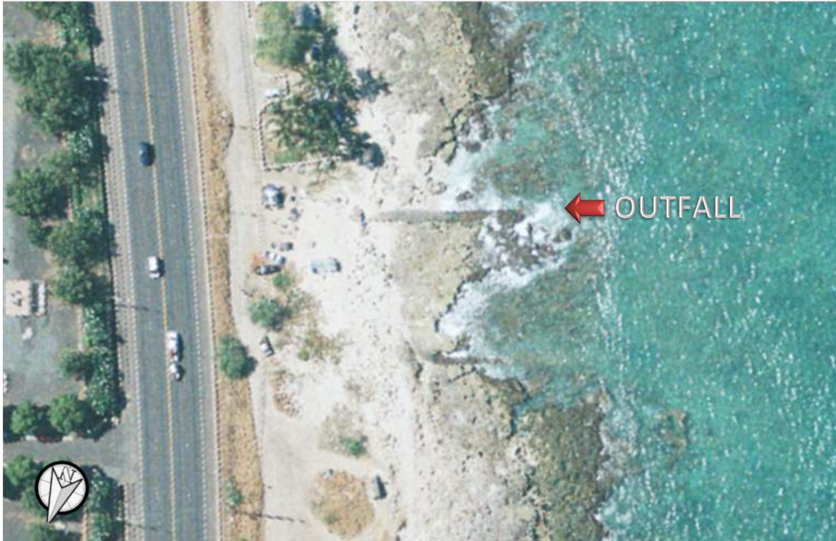
Figure 5-7. Outfall landing shoreline condition, 2007 (source: UH Coastal Geology Group, 2019)
