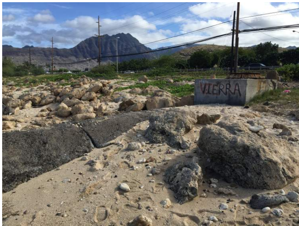
Figure 1-3. Outfall shoreline emergence with junction/valve box.
