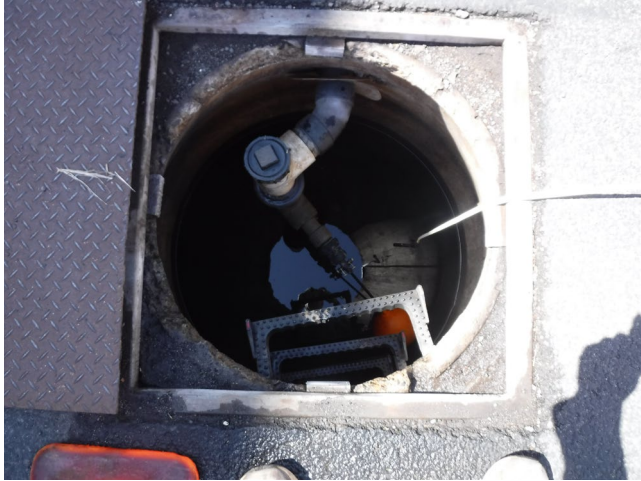
Photo 1: Overhead view of Well 1 All photos taken on August 24, 2022
