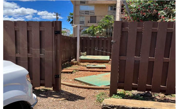
Photo 4: Gate to wastewater treatment system enclosure.
