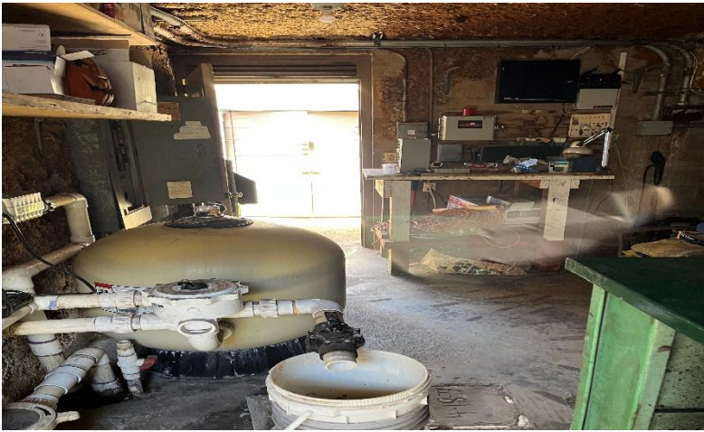
Photo 13: Interior of blower room.
