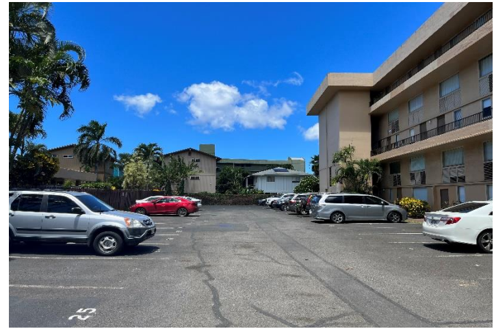
Photo 2: East parking lot facing north.
