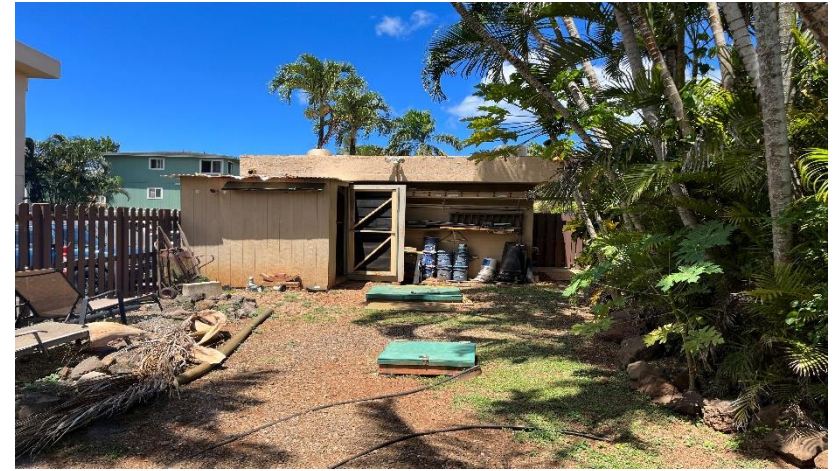
Photo 6: North portion of wastewater treatment system enclosure - facing north.
