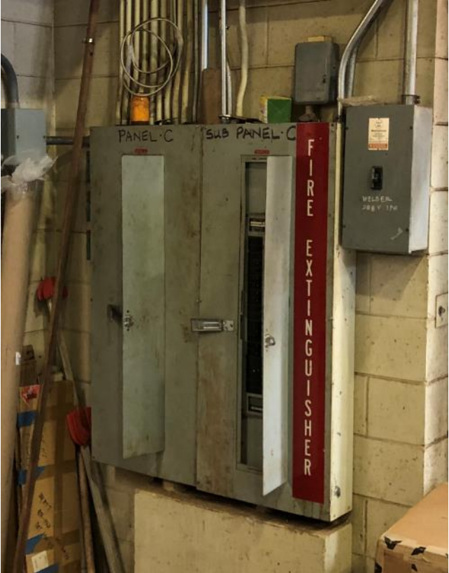
Photo 8: Electrical panels 'D(1)' 'D(2)' and 'C.' Examples of electrical panels in need of replacing.
