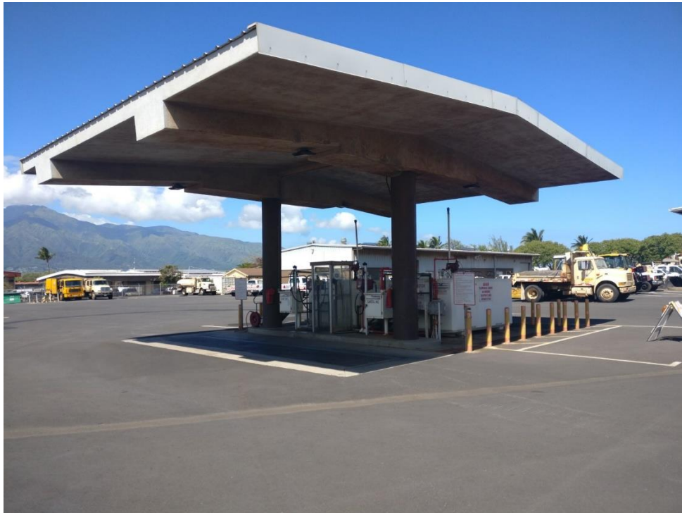
Photo 4: Fueling station. Looking southwest.
