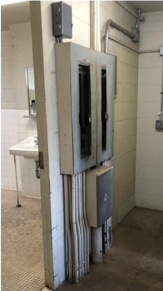
Photo 8: Electrical panels 'D(1)' 'D(2)' and 'C.' Examples of electrical panels in need of replacing.
