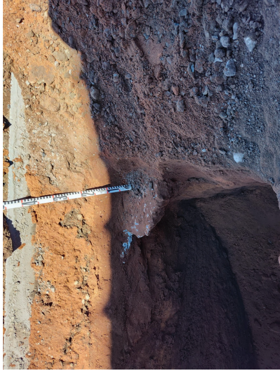
Figure 36: Photograph of the ST-8 east wall taken on September 28, 2022 with the concrete kicker visible in the foreground
