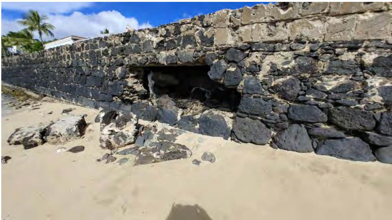
Figure 2-5: Seawall Repair That is Not Part of This Project
