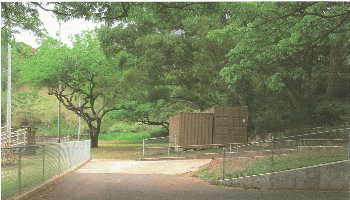
Photograph 2. East View of Building Site. Flat Area in Background and Hillside on the Right. Chain Link Fence at Left Generally Demarcates the Zoning District Boundary Between the Park (Left) and School (Right).
