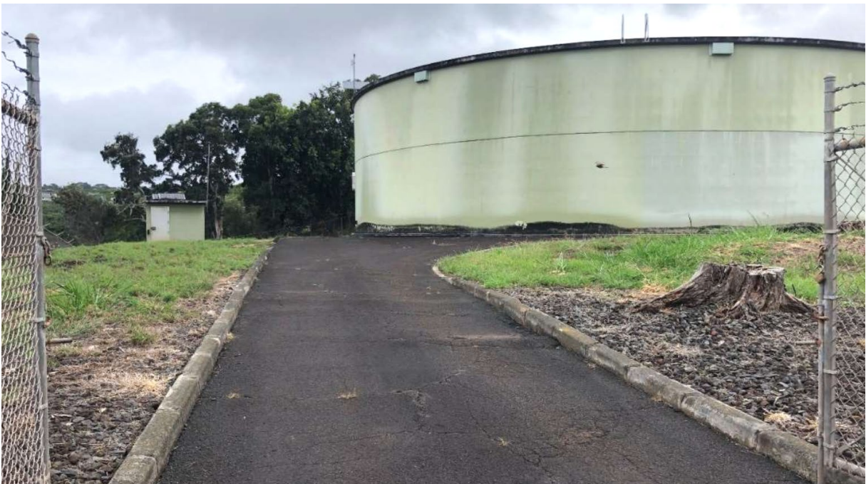
Photo #2. View of the existing above-ground reservoir tank and control building from the gated entrance along Piki Street. The project site is secured with perimeter chain link fencing topped with barbed wire. Access to the facility is restricted by a gated entry. The access road to the reservoir is paved.
