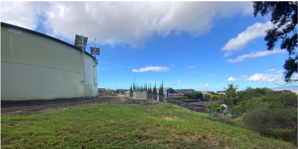
Photo #10. View looking west from the rear portion of the project site and behind the existing reservoir. The northwestern corner of the project site slopes towards the adjacent wooded area beyond the perimeter chain link fencing.
