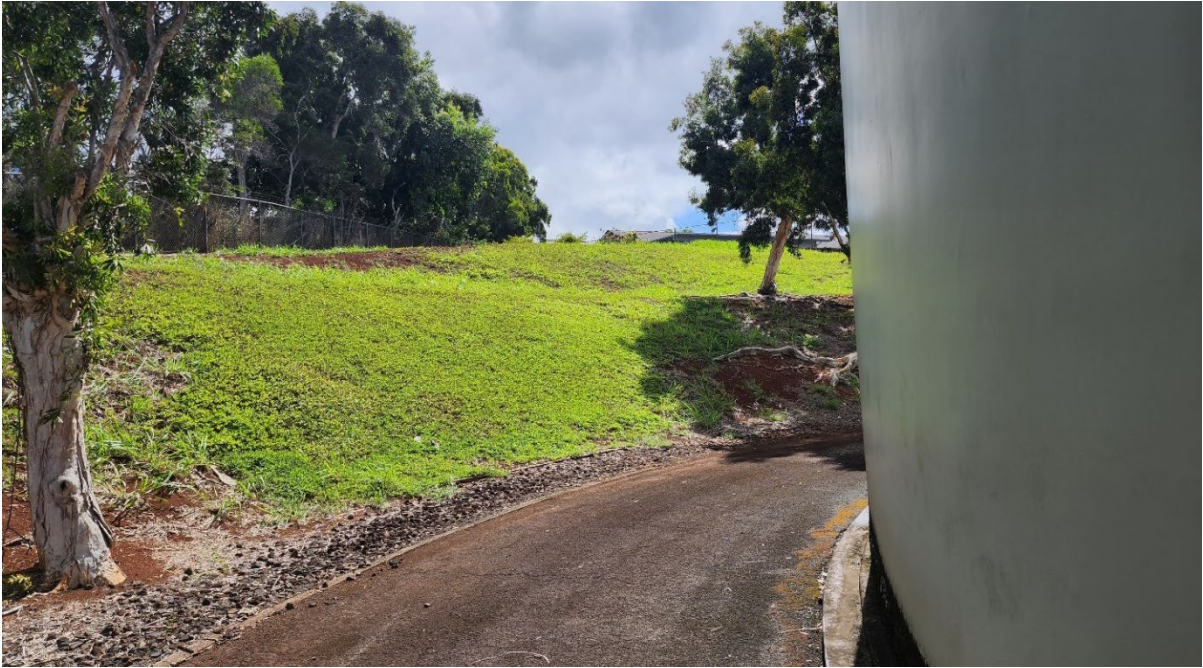
Photo #7. View of the steeper areas behind the existing reservoir and along the rear portions of the project site. A densely wooded area defines the rear property line and is behind and along the perimeter chain link fencing. Vegetation within the project site includes grasses and a few tall trees around the reservoir.
