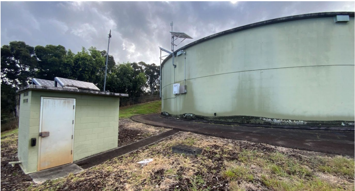
Photo #6. View of the reservoir and control building from within the project site. The built structures are painted green, which is the typical color currently used for BWS facilities.
