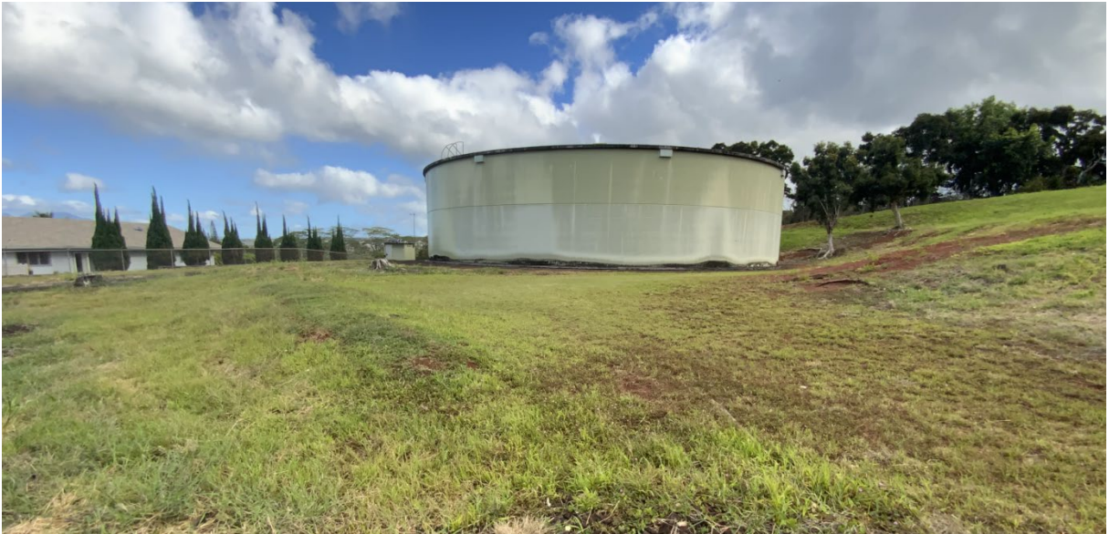
Photo #1. View looking northwest towards the existing above-ground reservoir tank and control building. The project site was previously graded for the initial site development of the Newtown 550' facility and the flatter portions are towards the front of the parcel. An adjacent single-family residence along the western border of the project site is visible in the photograph.
