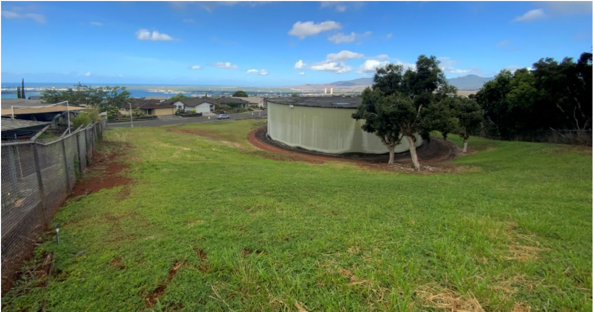
Photo #9. View of the existing reservoir from steeper areas on the eastern portion of the project site. There are a few tall trees around the reservoir. Single-family residences along the eastern site boundary and along Piki Street are visible in the photograph. The steeper areas of the project site provide glimpses of Pearl Harbor.
