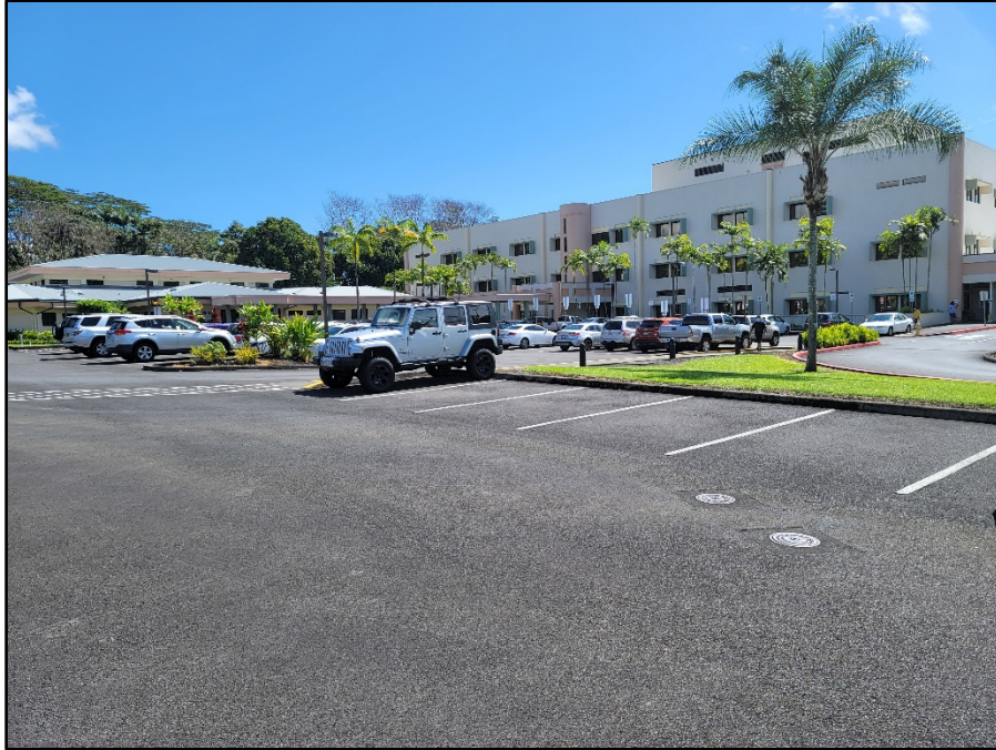
Figure 16. Photo overlooking the project area (within the existing HMC parking lot) with the hospital facility visible in the background; view to northeast
