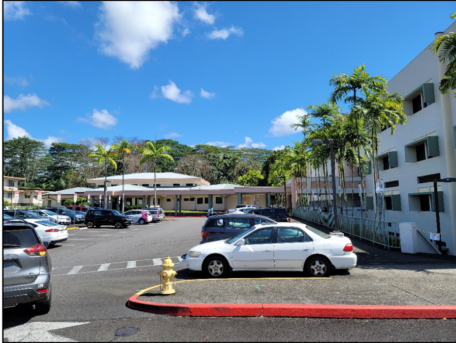
Figure 18. Photo overlooking the project area (within the existing HMC parking lot) with the hospital facility visible in the background and to the right; view to north
