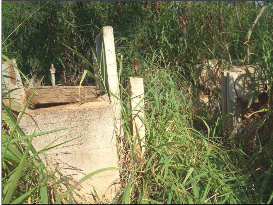
Figure 54. Photo of the historic water diversion structure (SIHP # -4664), Sluice Gate Location 1
