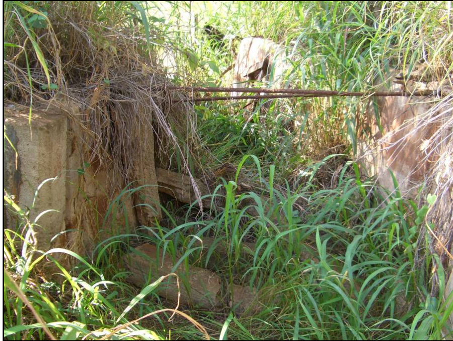
Figure 56. Photo of the historic water diversion structure (SIHP # -4664), Sluice Gate Location 2
