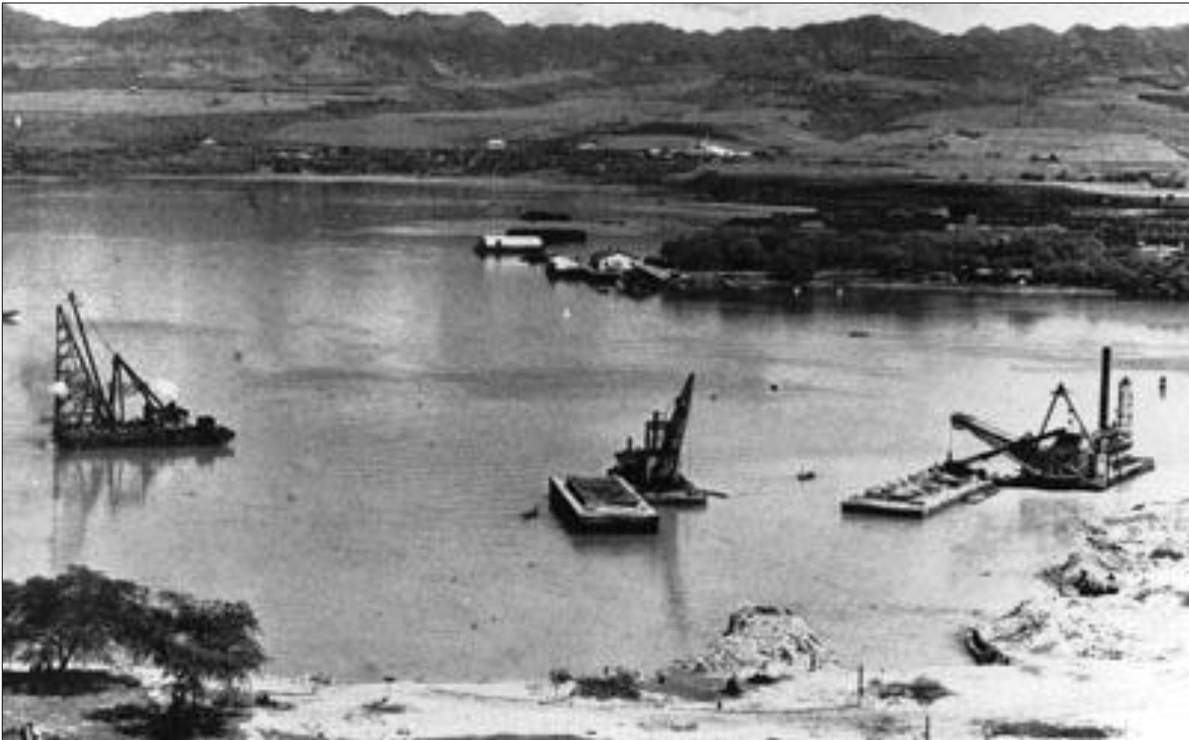
Figure 25. Dredging in Pearl Harbor ca. 1908 (Hawai'i State Archives)
