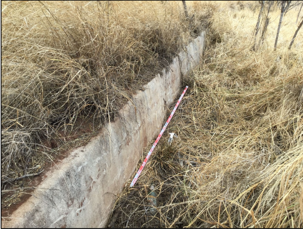
Figure 48. Retaining wall, portion of CSH 1, view to north
