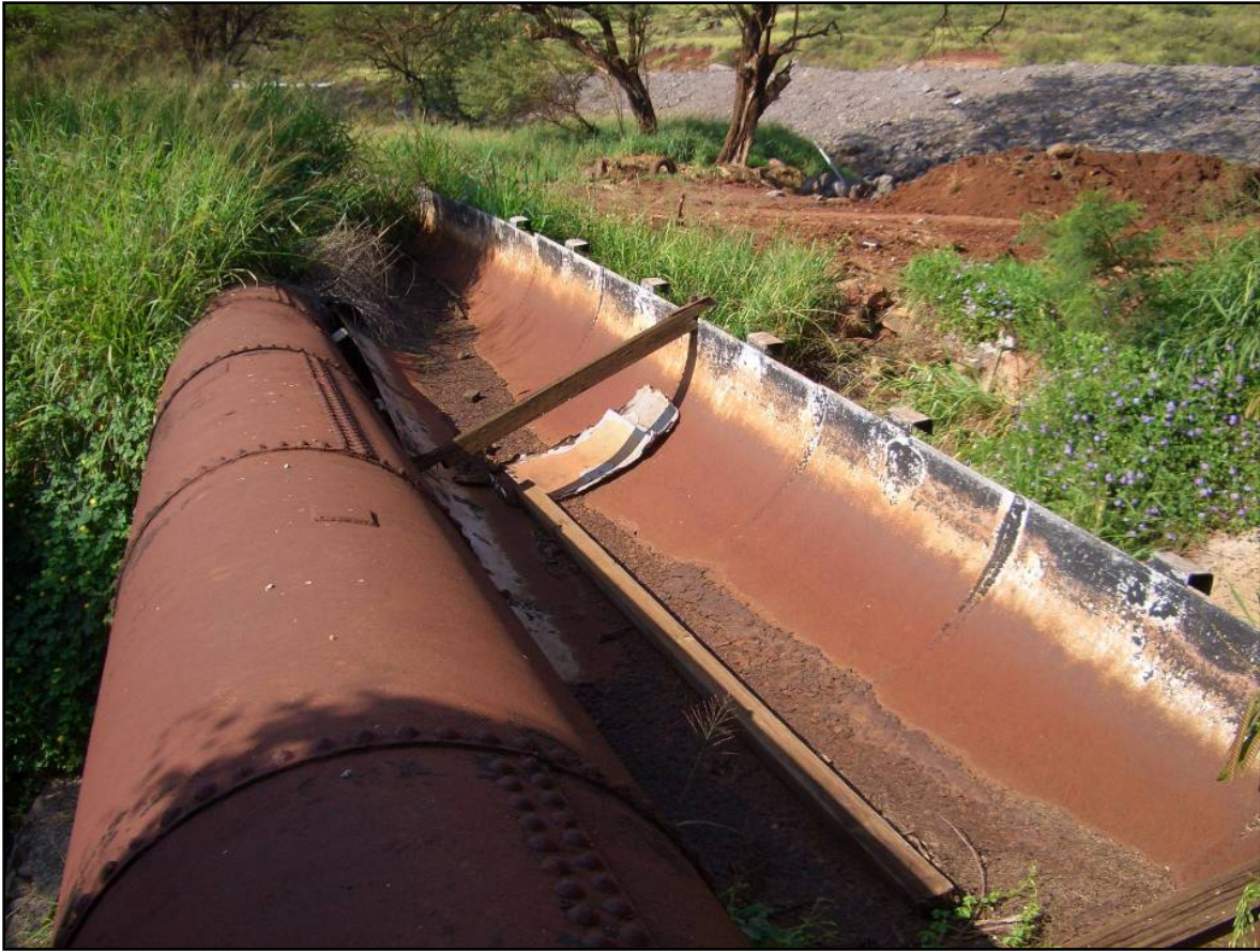
Figure 52. Photo of the large metal siphon pipe (left) and metal flume (right) located along the southwest edge of Ramp C crossing Hunehune Gulch (SIHP # -4664), view to west
