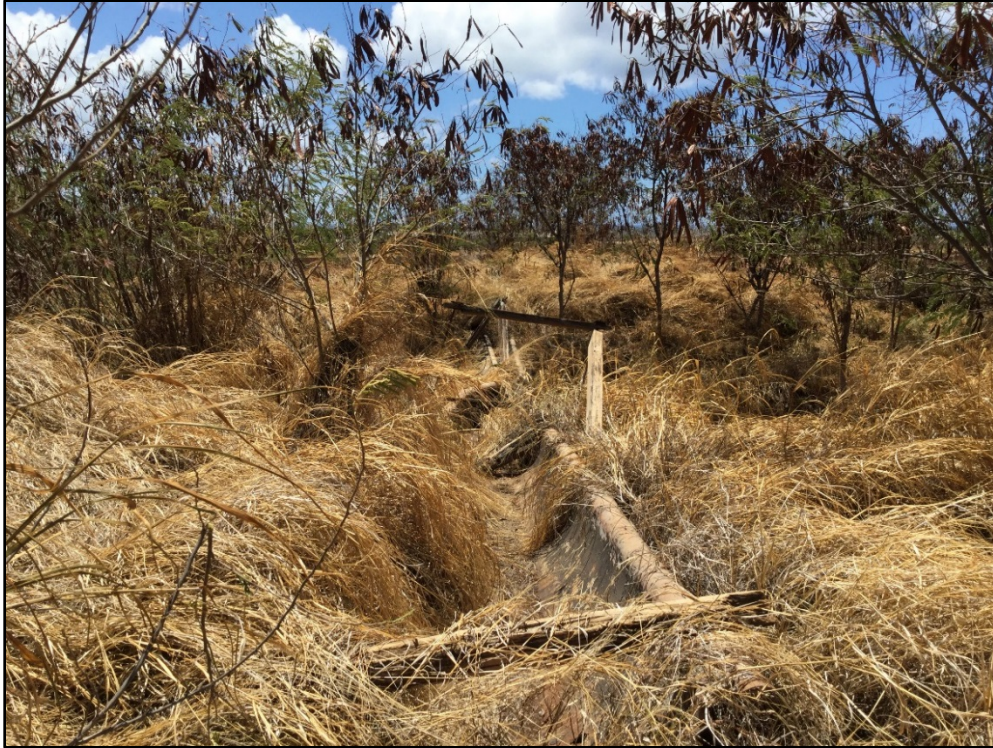
Figure 38. Broken flume remnant located south of the proposed R-1 reservoir, view to southwest
