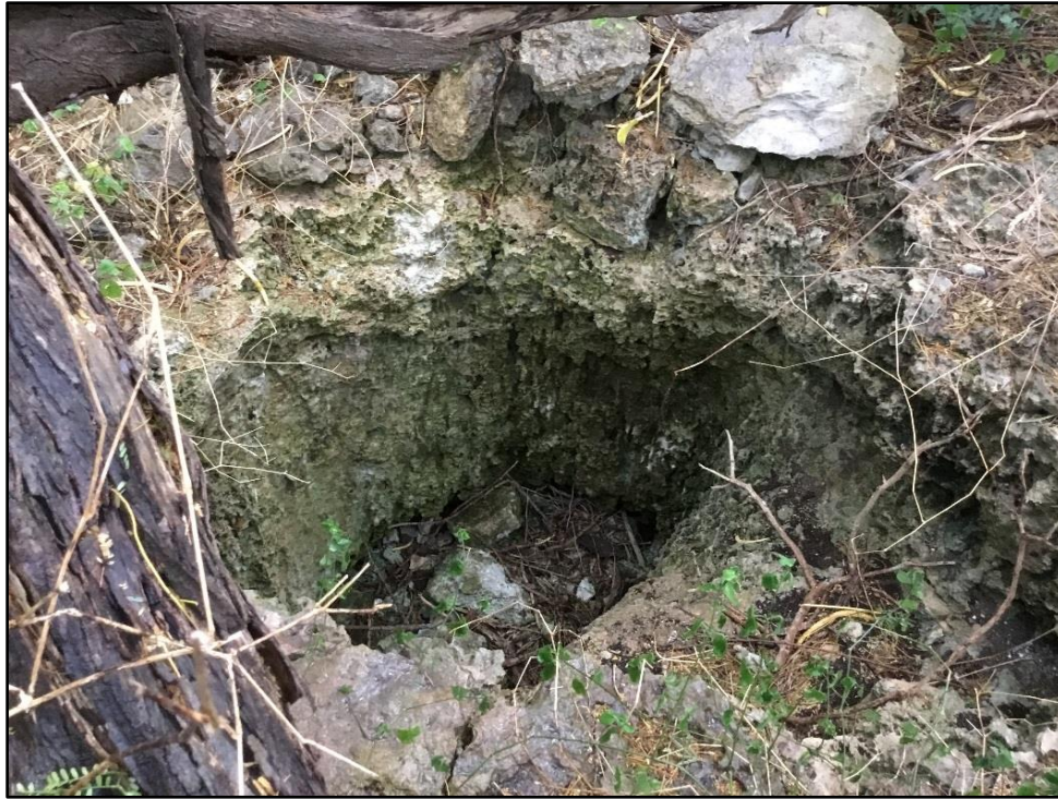
Figure 35. General view of interior of sinkhole; it is believed to have once functioned as a well or cistern, within the Kalaeloa Heritage Park
