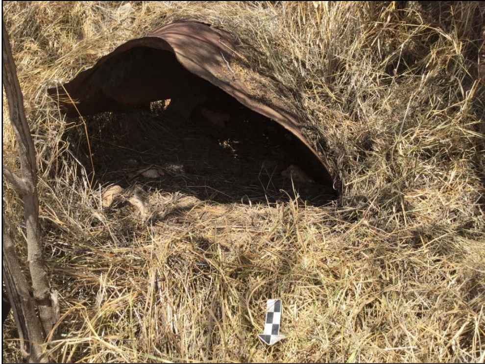
Figure 46. Exposed metal culvert, portion of CSH 1, view to south
