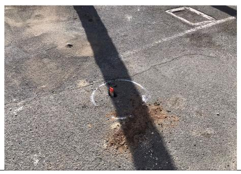
Temporary groundwater wells were installed at two locations within the DU (one upgradient, one downgradient)
