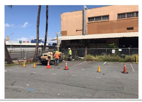
FAI retained Geotek to conduct drilling using a track-mounted, direct push drill rig.
