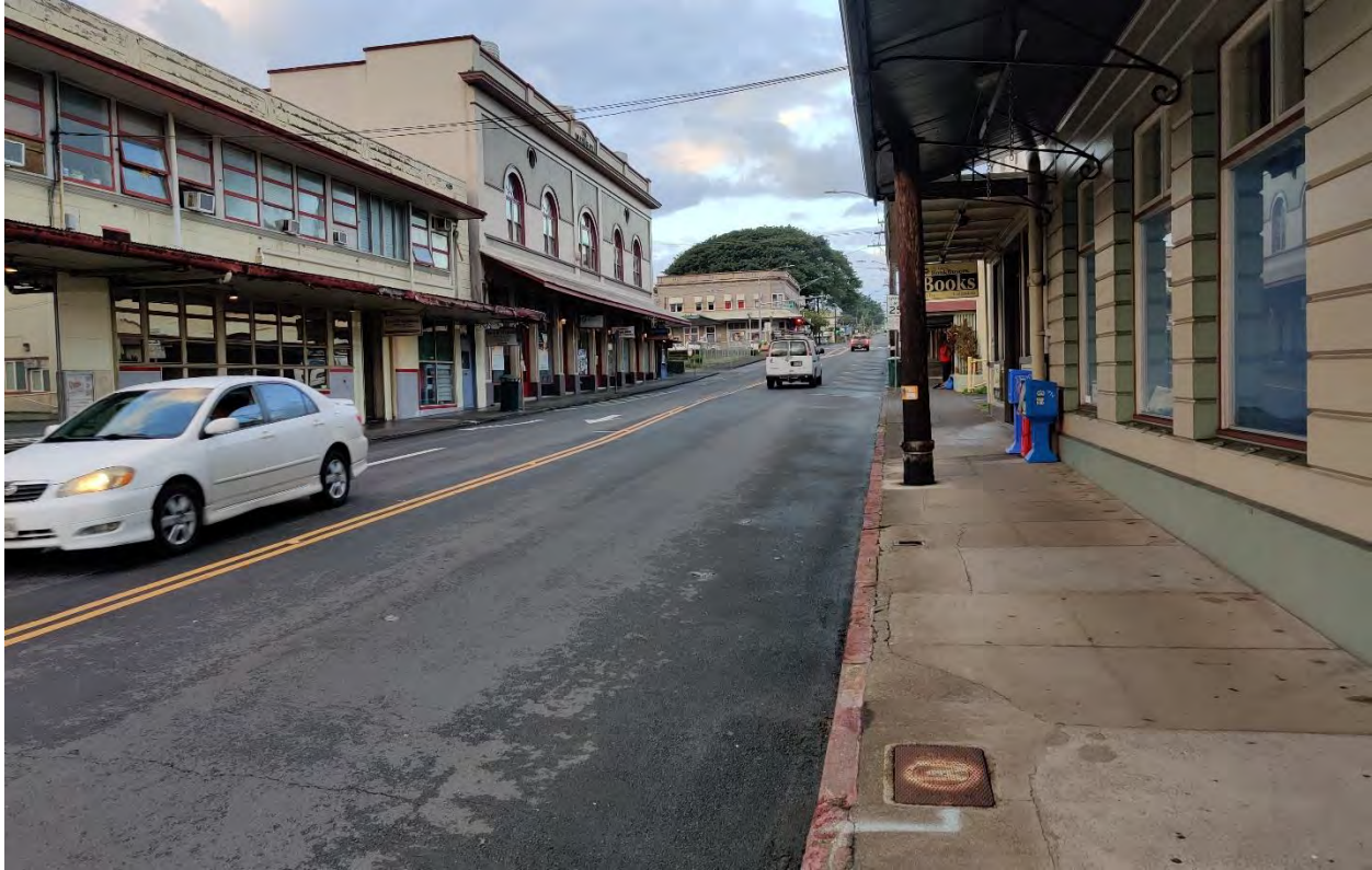
Figure 7 Mauka-bound View of Waiānuenue Avenue
