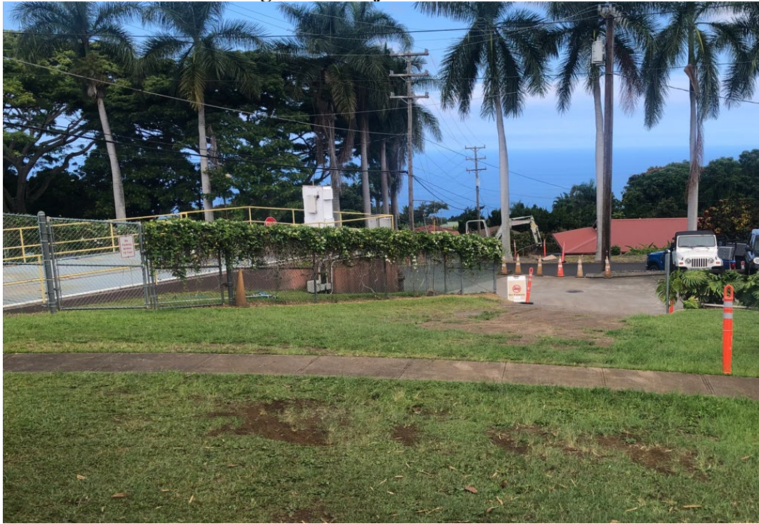
2a, Existing WWTs (left) and Proposed Site of Redundant System (right)
