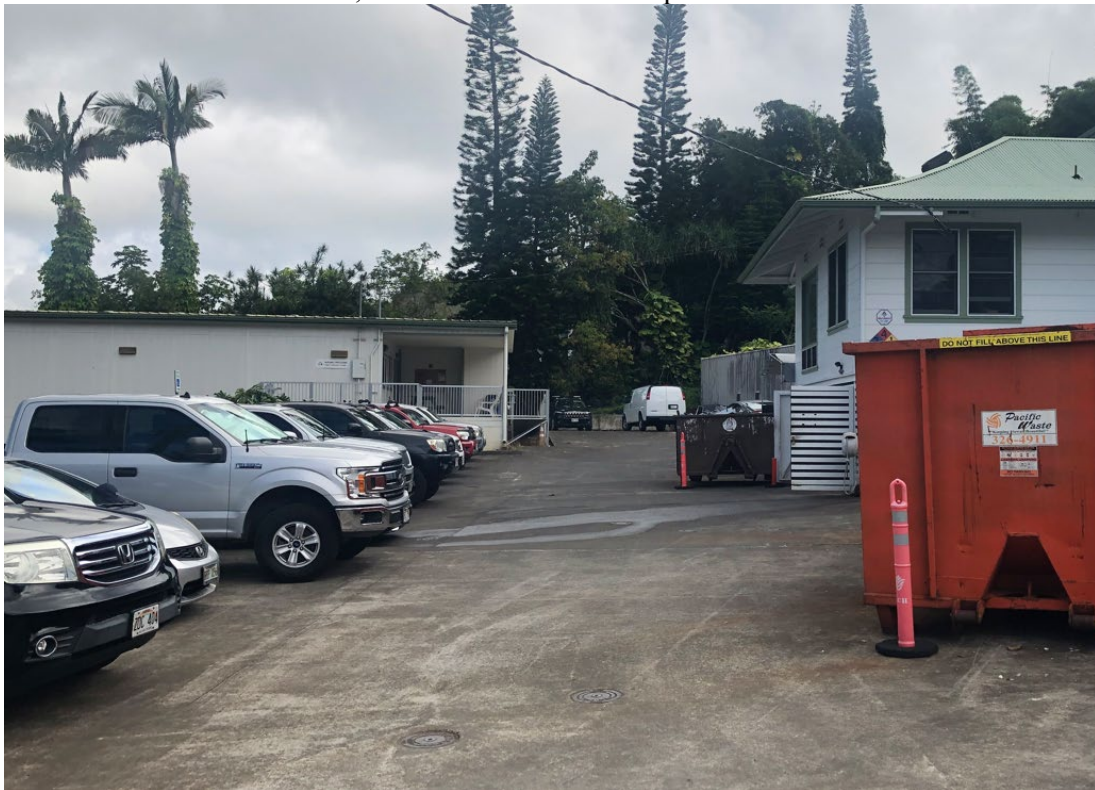
2b, Site of Subsurface Absorption Bed
