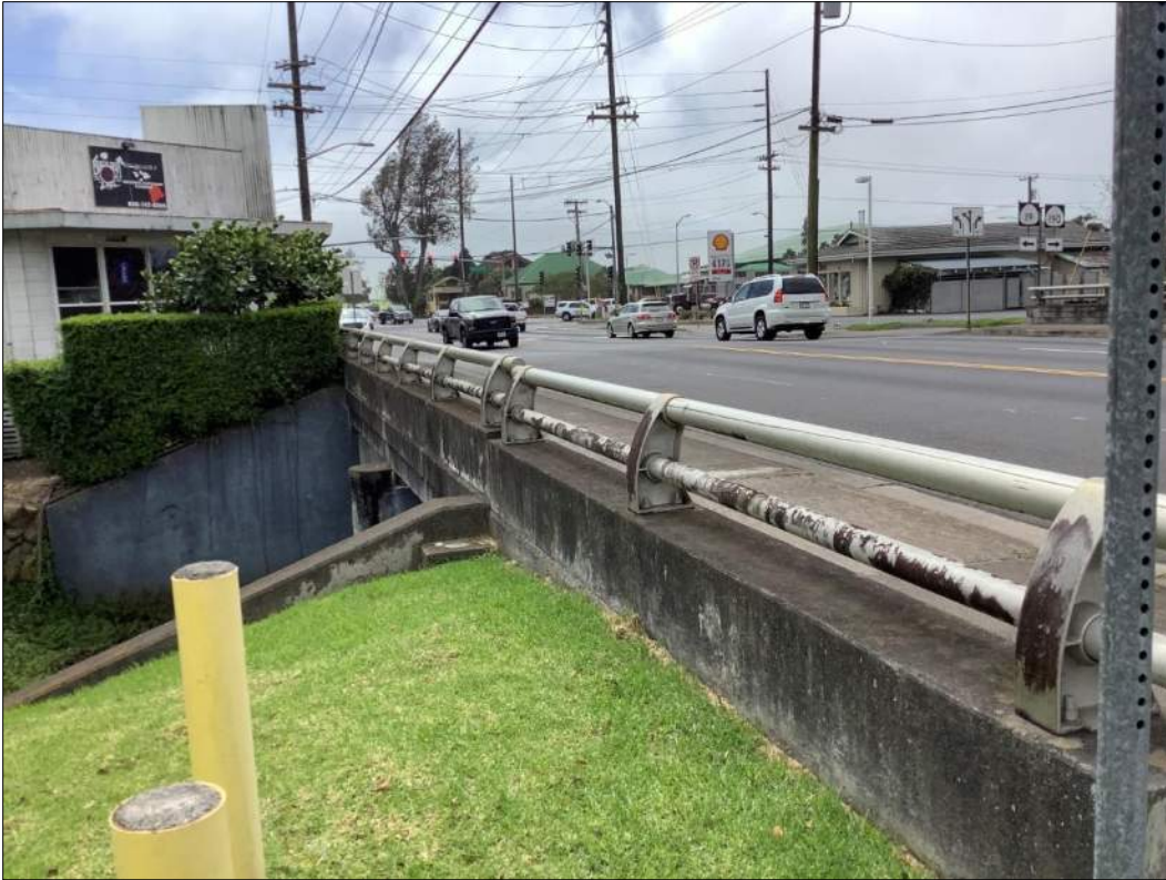
Figure 23. Waikoloa Bridge, view to the south.
