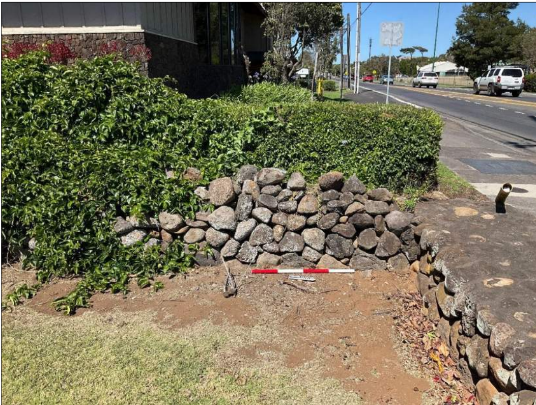
Figure 58. Site T-1 rock wall on western parcel boundary, view to the west.
