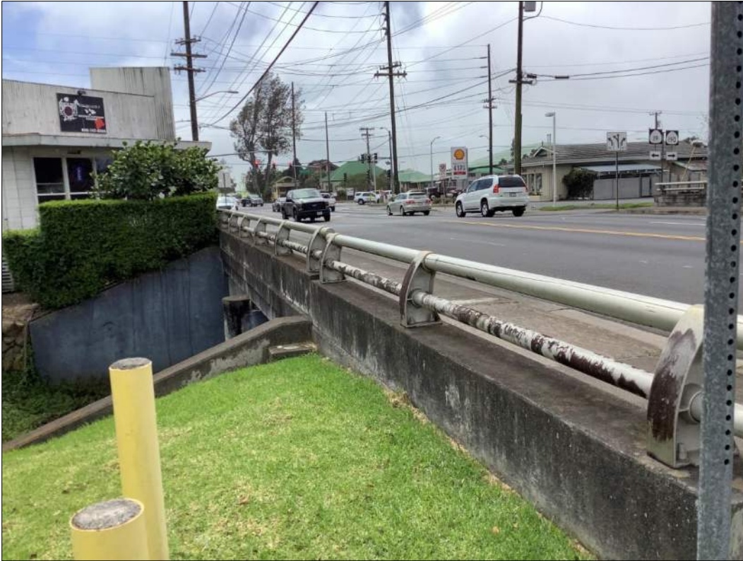
Figure 23. Waikoloa Bridge, view to the south.
