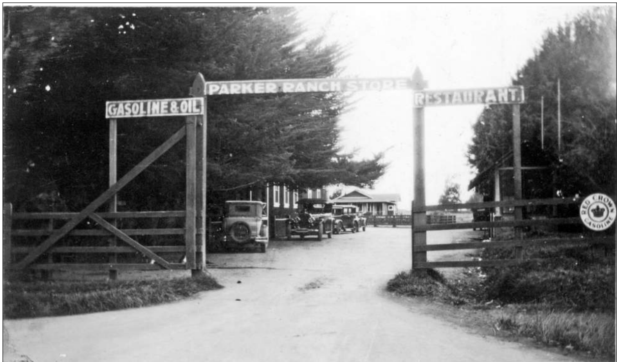
Figure 34. Entrance to the former Parker Ranch store and restaurant ca. 1930s (photo courtesy of the Kō Education Center, Honoka‘a).
