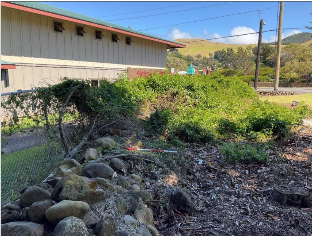
Figure 56. Site T-1 rock wall on western parcel boundary, view to the north.
