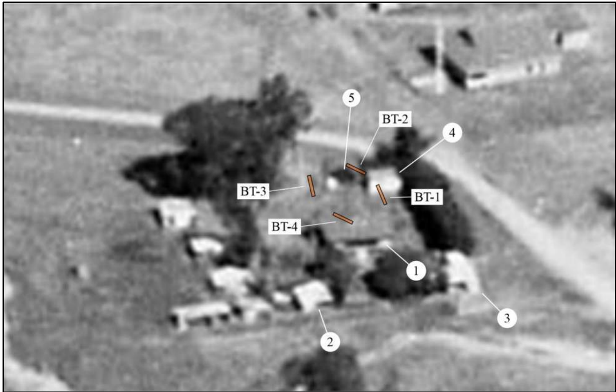
Figure 48. Location of trenches relative to buildings shown in the 1925 aerial image (USAAF 1925).
