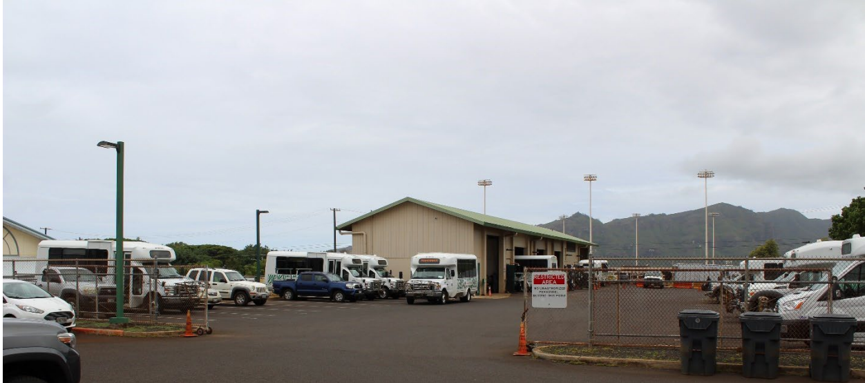
View of the existing maintenance building, looking south.
