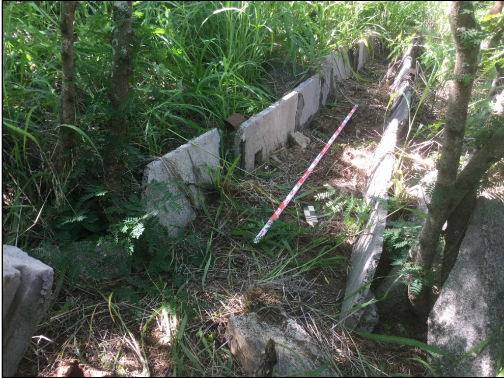
Figure 39. Photo E: Portable Ditch Unit (PDU) alignment 1, view to south
