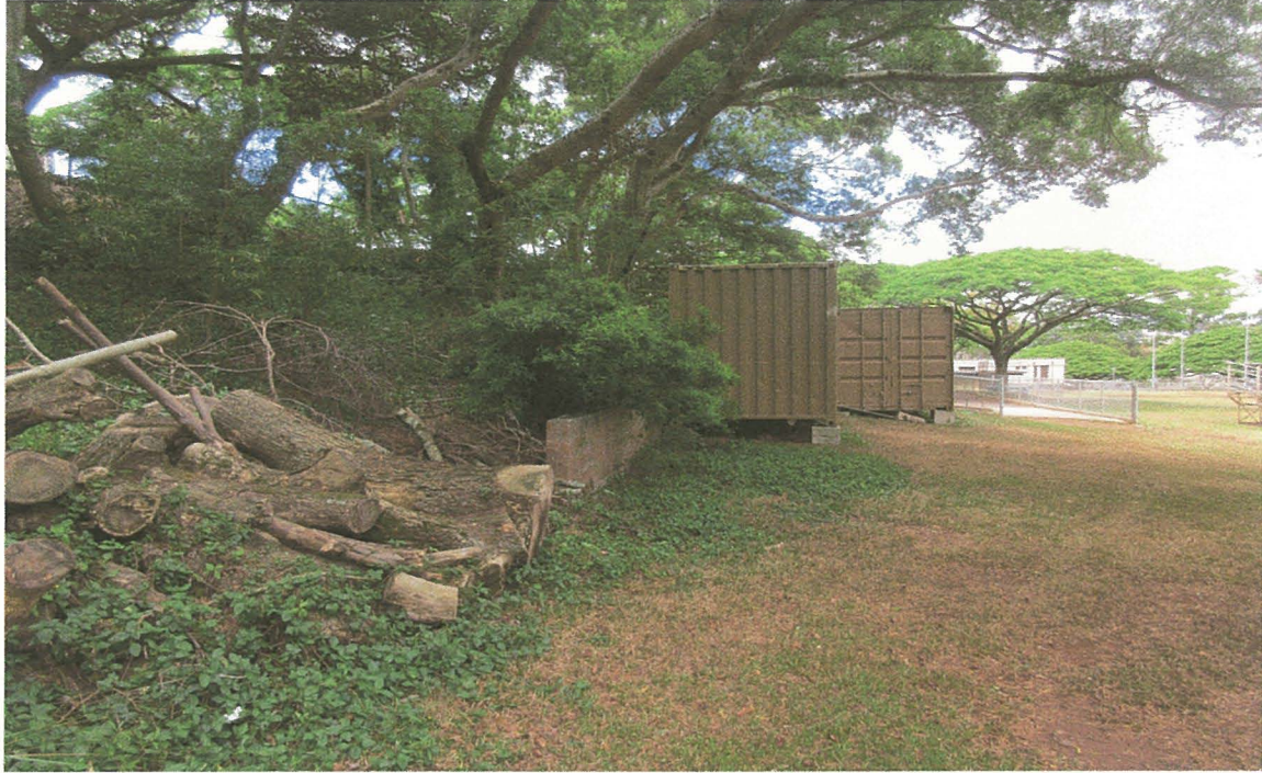
Photograph 1. West View of Building Site. Flat Area on Right, Hillside on Left.
