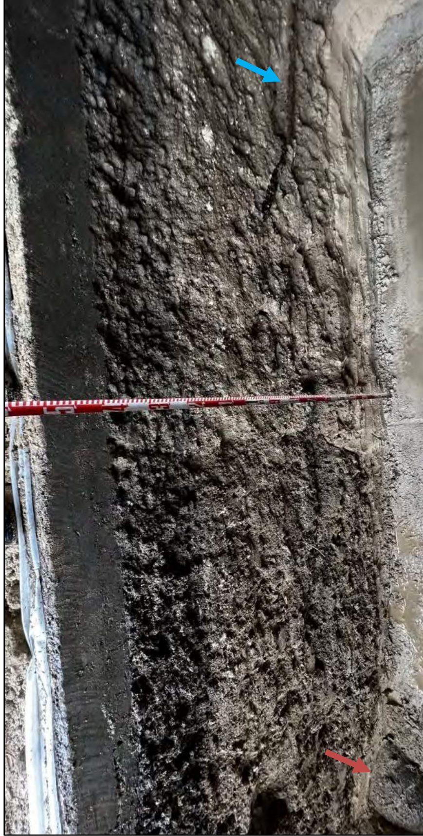
Figure 72. T-2 northeast sidewall, view to northeast; note 4-cm diameter metal utility pipe in Stratum Ic (indicated with blue arrow) and 24-inch sewer line in Stratum If (indicated with red arrow)
