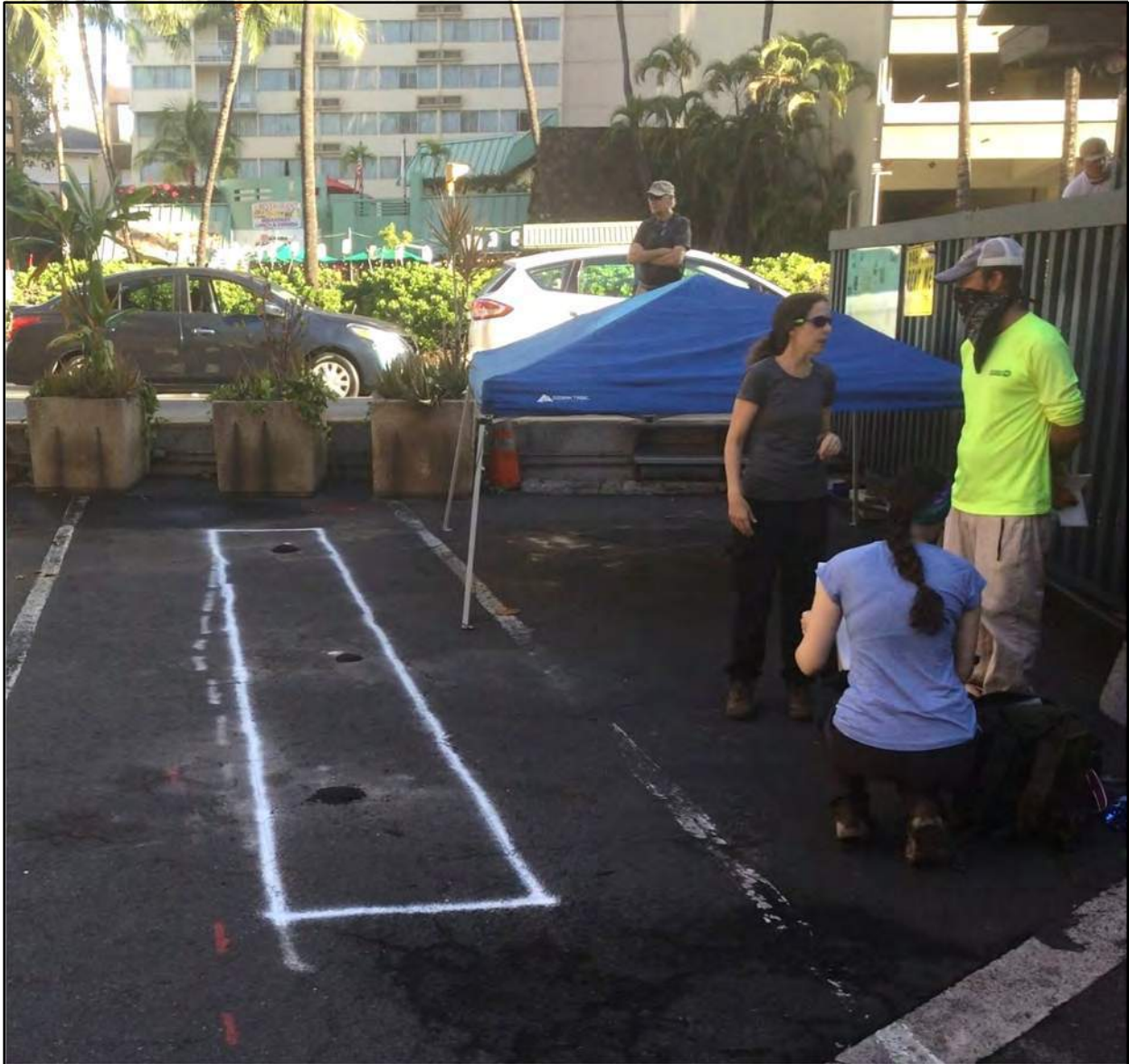
Figure 91. Location of T-5, view to northwest; Paradise Rent-A-Car building on right, Ala Moana Boulevard in background; note the red spray paint indicating a subsurface utility southwest of the trench
