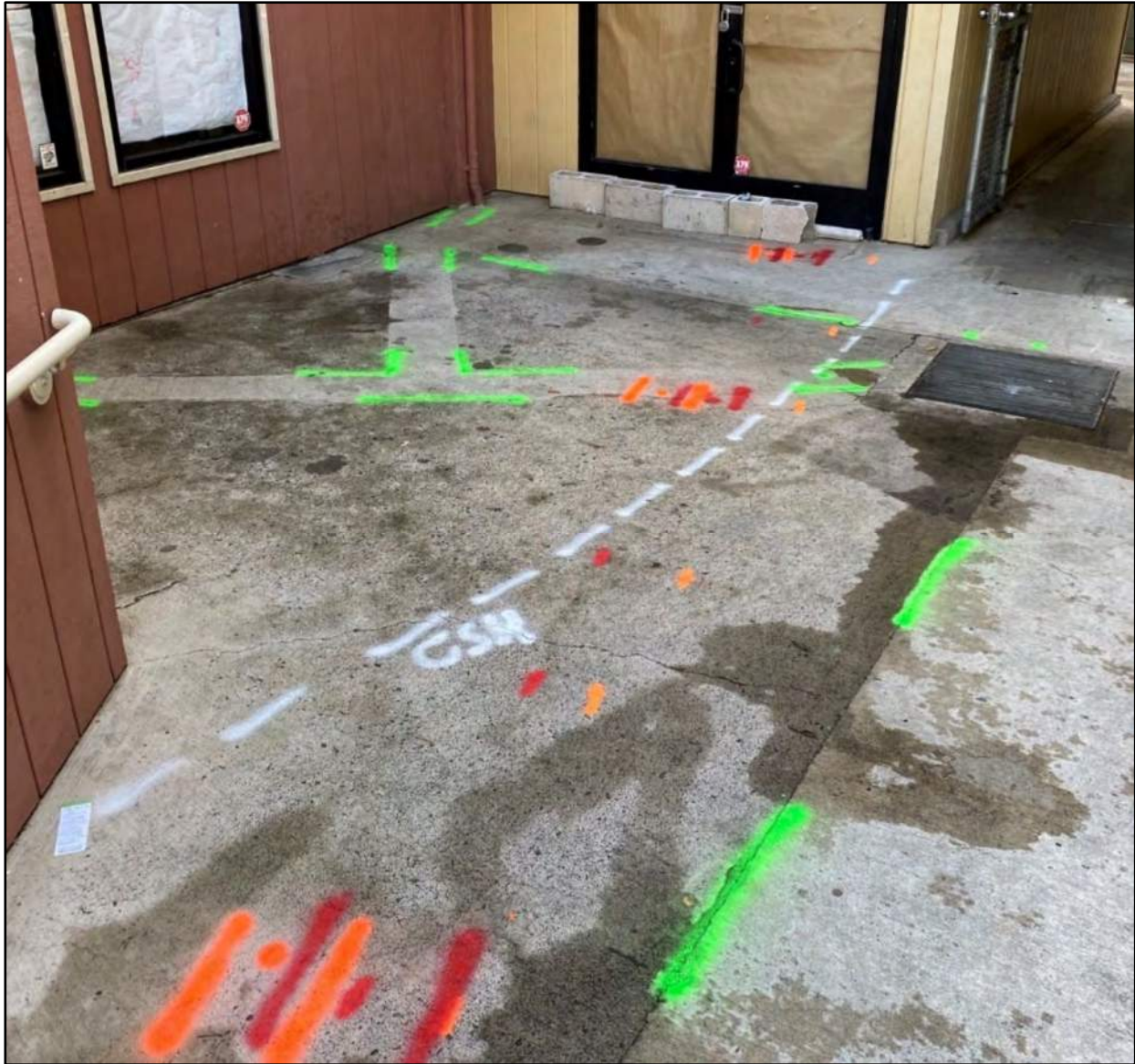
Figure 17. Subsurface utilities (orange, green, and red spray paint) in the planned location of T-3 (dashed white line), view to east
