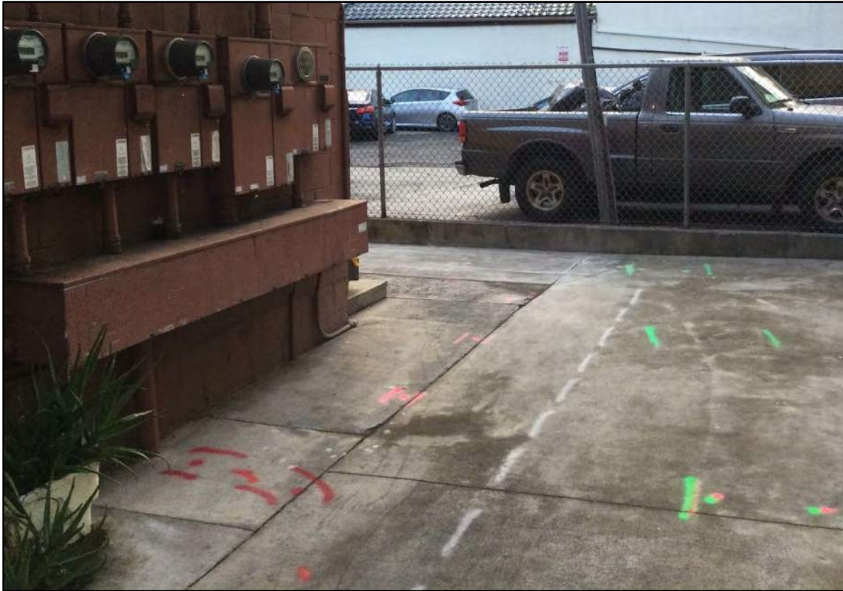
Figure 15. Subsurface utilities (green, pink, and orange spray paint) in the planned location of T-1, view to northeast
