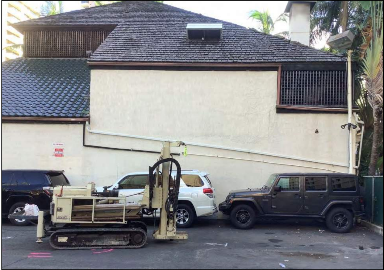
Figure 59. Boring at T-7, view to northeast; Kobe Steakhouse building in background
