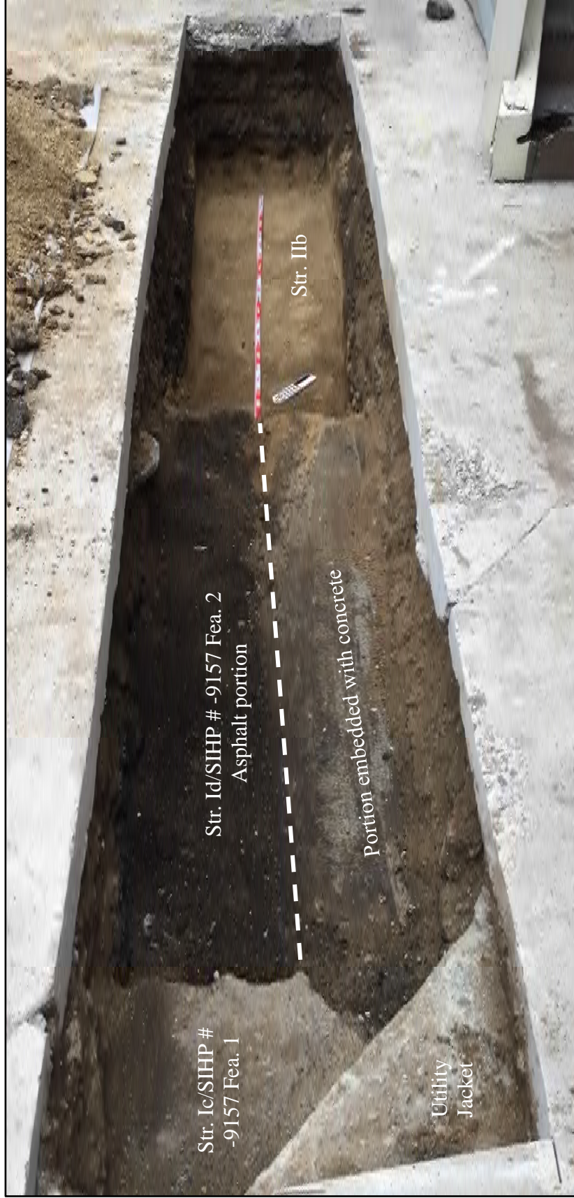
Figure 79. Plan view of T-3 at 19-112 cmbd, showing the concrete utility jacket at the west corner of the trench (bottom left); the portion of the Stratum Ic/SIHP # -9157 Feature 1 buried asphalt layer remaining after most of it was removed by the excavator (top left); and Stratum Id/SIHP # -9157 Feature 2, buried asphalt layer partially embedded with concrete, in the northwestern portion of the trench (center) atop the soil/sediment bench
