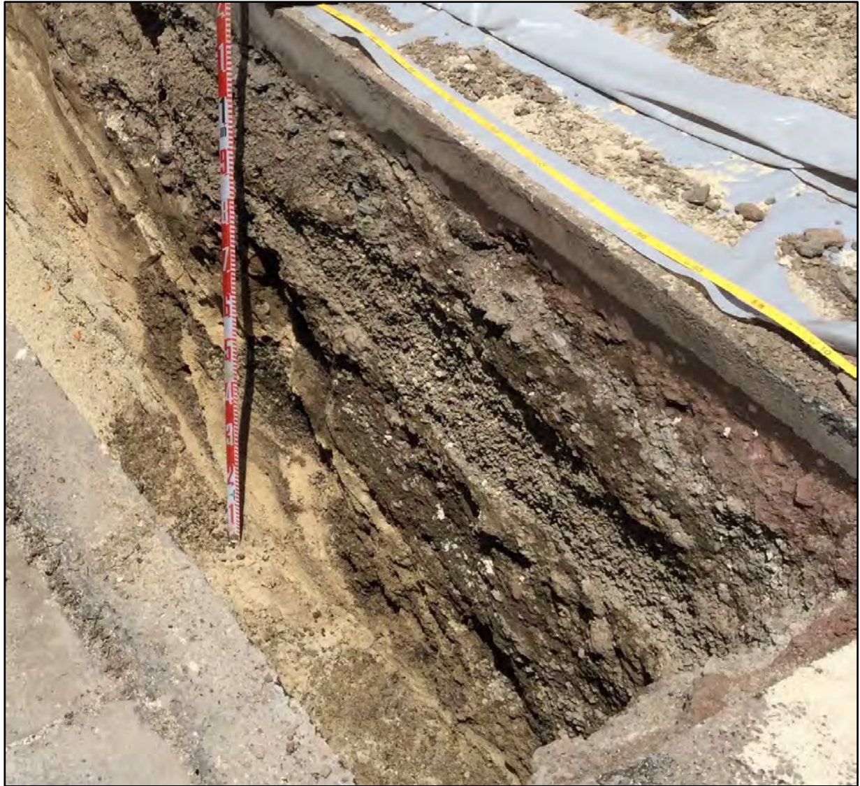
Figure 100. Southeast end of T-6 northeast sidewall, showing a large area of disturbance
