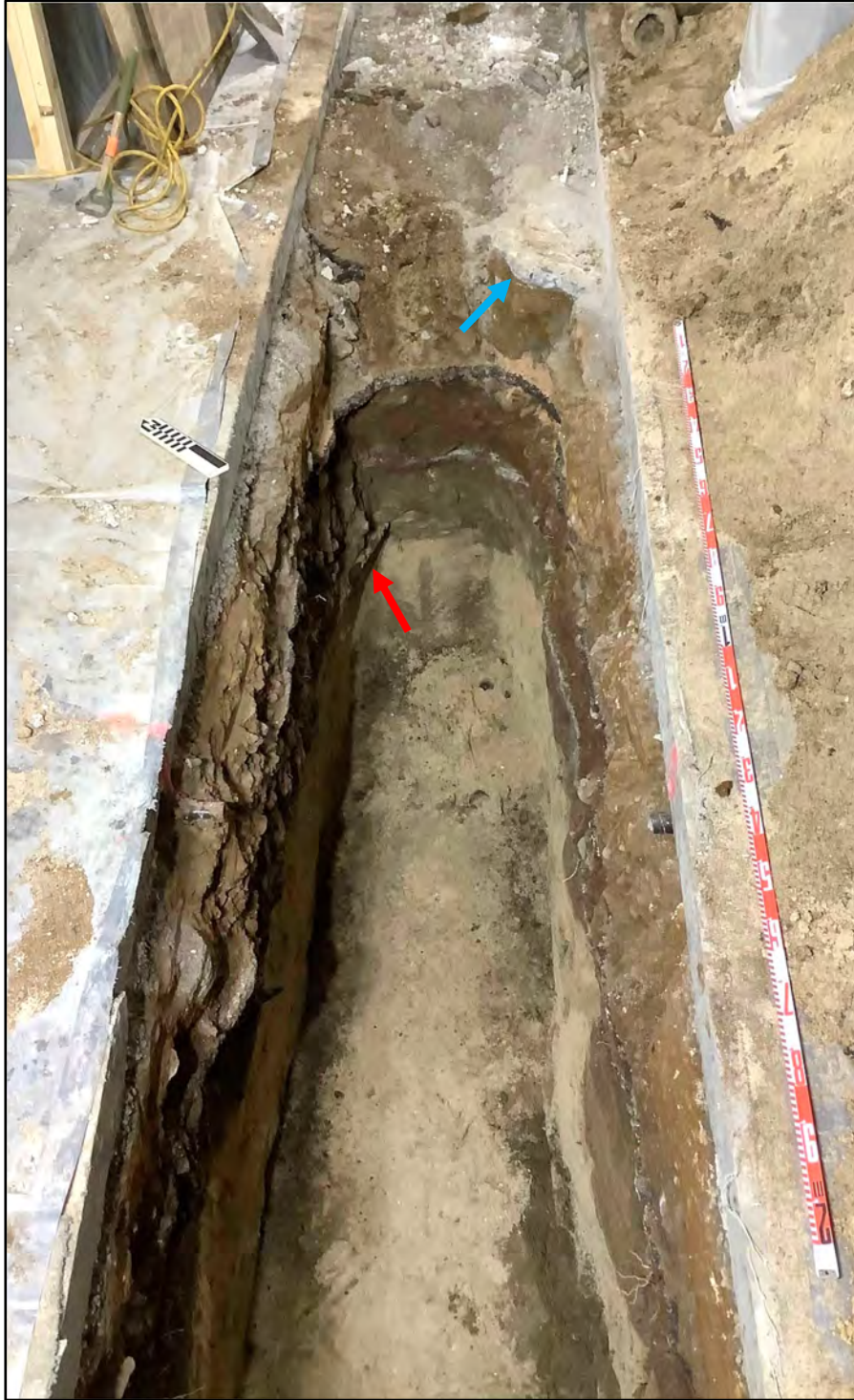
Figure 129. Plan view of T-9, showing a cast iron utility pipe at 100 cmbs (indicated with red arrow) extending from the northwest sidewall into the planned footprint of the trench) and a concrete footing (indicated with blue arrow) extending from the southeast sidewall into the planned footprint of the trench
