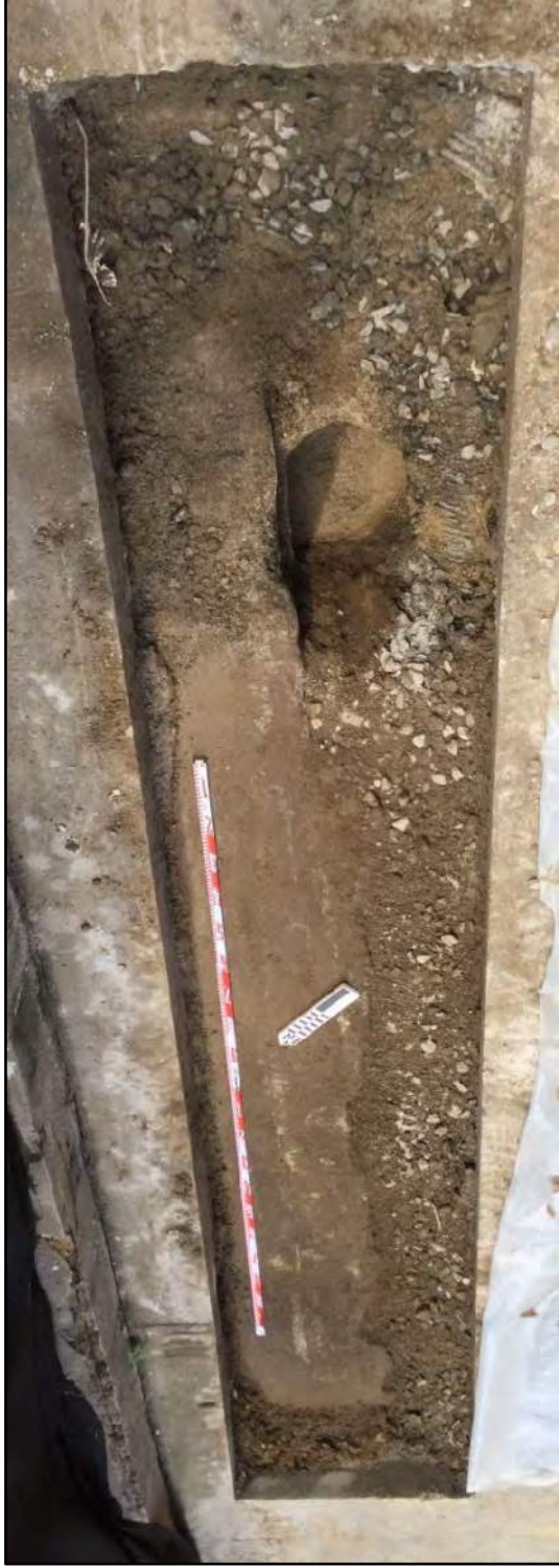
Figure 65. Plan view of T-1 showing a concrete utility jacket along the northeast sidewall (top), a plastic sump pump line at the south corner (bottom right), and a pothole excavated between the two (center/right)
