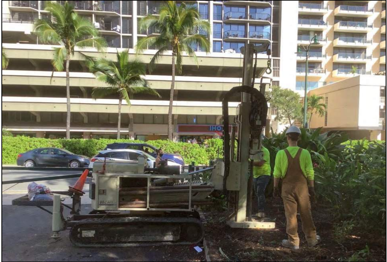
Figure 61. Boring at T-8, view to northwest; Ala Moana Boulevard in background
