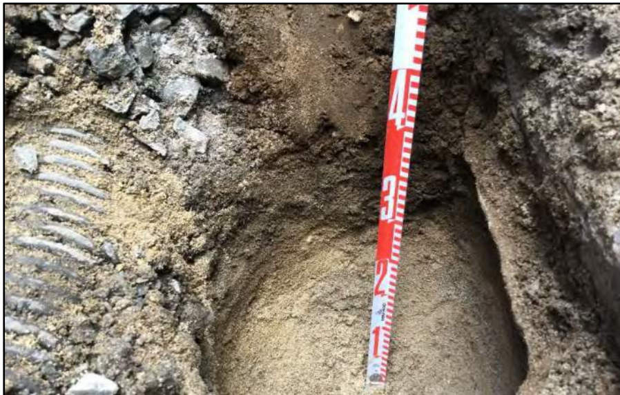
Figure 68. T-1 pothole, northwest wall, view to northwest; concrete jacket on right, plastic sump pump line on left
