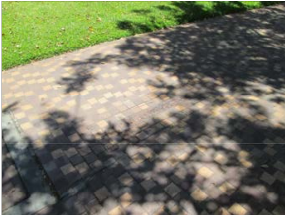
PHOTO 3: TRENCH DRAIN IN DEPRESSED AREA.
