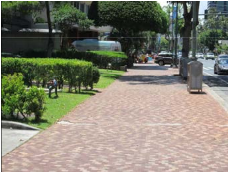
PHOTO 1: EXISTING SIDEWALK FRONTING THE PROJECT SITE. DEPRESSED SIDEWALK AREA IS ADJACENT TO EXISTING TREE ALONG CURB LINE
