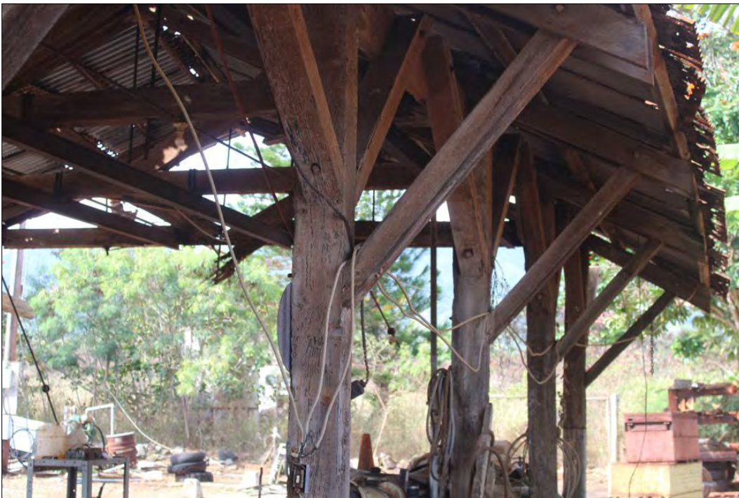
Figure 55. SIHP Site TS-02 3-way knee bracing and eave.
