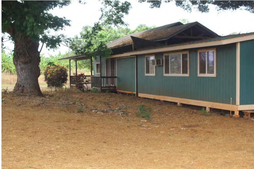
Figure 74. Front elevation of former camp store building (now completely renovated), view to the southeast.
