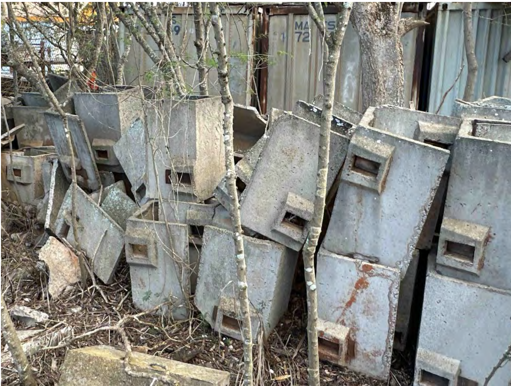
Figure 57. SIHP Site TS-02 concrete flume segments with sluice gates (Bulldogs) located to the west of the concrete facility, view to the east.
