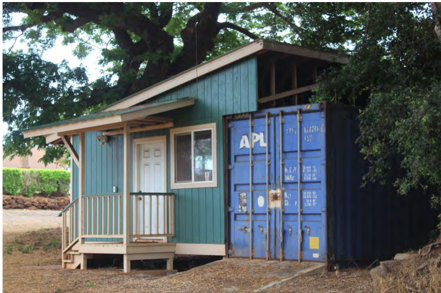
Figure 75. Side elevation of new construction attached to former camp store building, view to the northeast.
