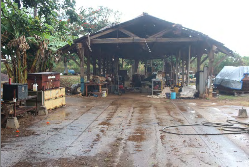
Figure 46. SIHP Site TS-02 missing portion (foreground) of main structure, view to the north.
