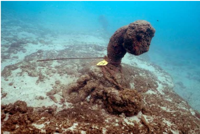
Photo 4 – Outfall Diffuser 29
