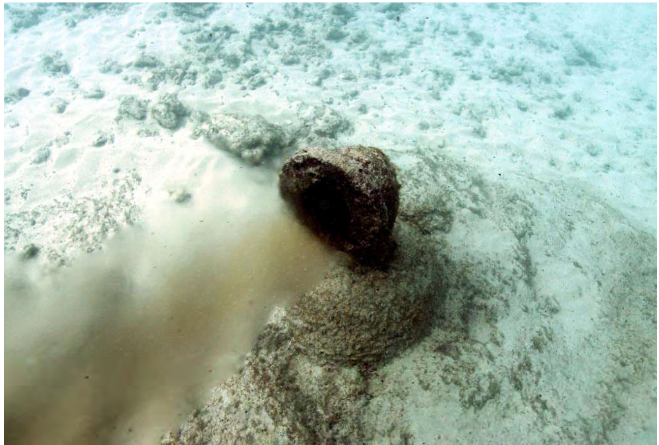
FIGURE 4. Photographs of two Wailua Wastewater Treatment Plant ocean diffuser ports discharging effluent taken on September 21, 2012. Note difference in sand cover of the area compared to photos taken in 2016 (Figures 2 and 3).
