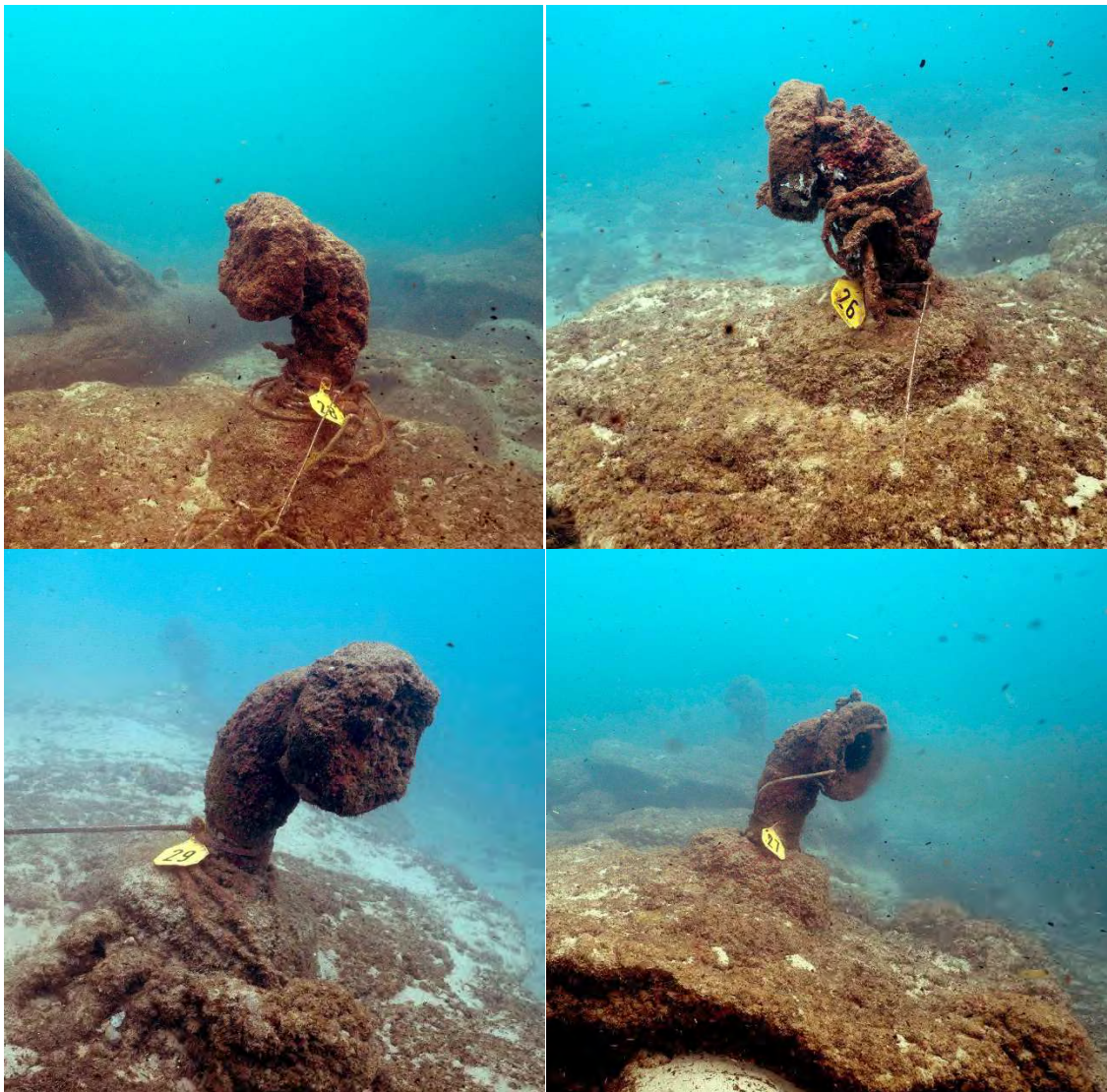
Figure 2. Wailua WWTP ocean outfall diffuser ports (MRC, 2021)
