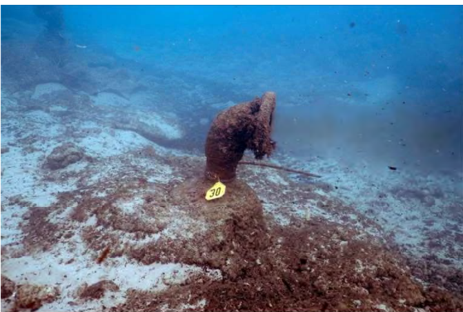
Photo 5 – Outfall Diffuser 30
