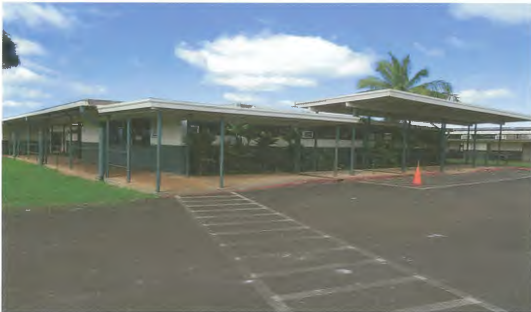
Photograph 1. West View of Administration Building
