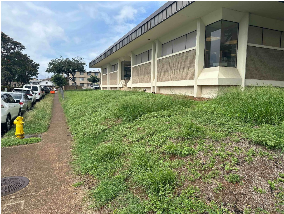
Figure 18. Southern side of Pearl City Public Library along Luehu St., view to the west.
