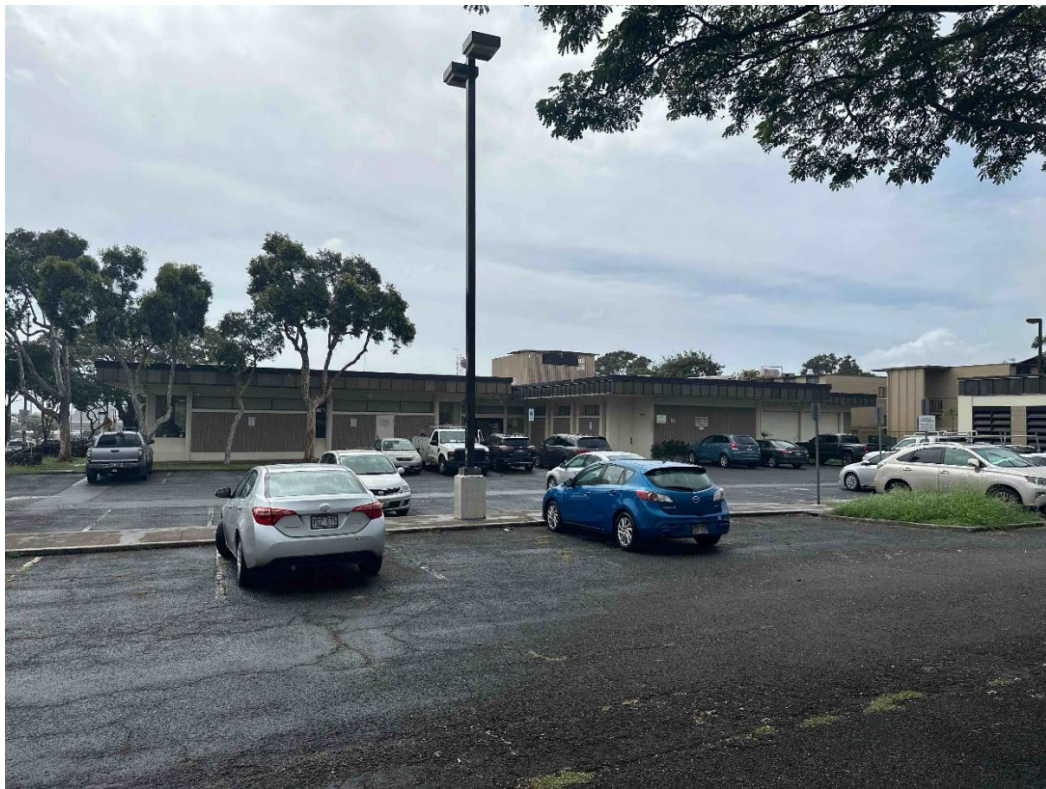
Figure 6. Northern side of Pearl City Public Library and parking lot, view to the south.
