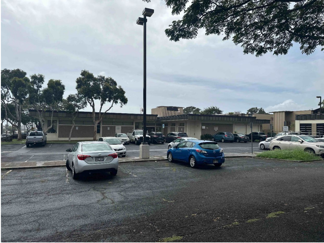
Figure 16. Northern side of Pearl City Public Library and parking lot, view to the south.
