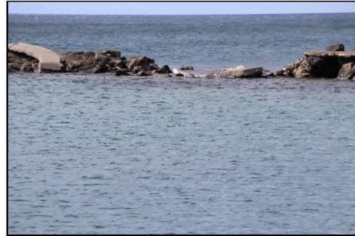
(b) January 2020. Breached section of Main Breakwater.
