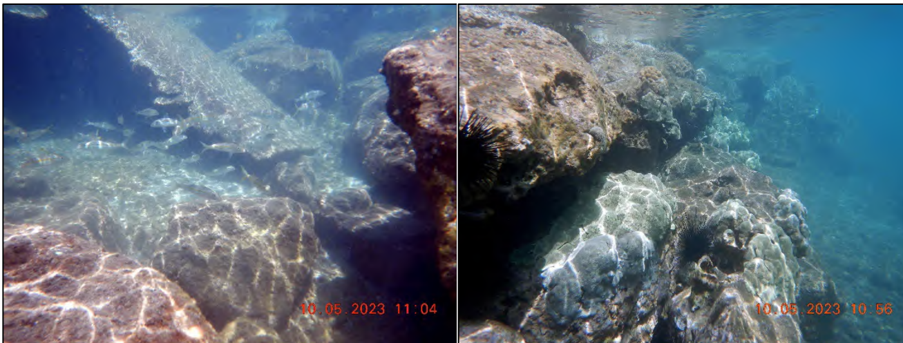
Figure 4. Inside the breakwater (within the yellow box in Fig. 3), broken pieces from the damaged structure occur on the seafloor; school of yellowfin goatfish ( M. vanicolensis ) are present (left). Corals ( Porites sp., and Poc. meandrina ) and urchins are abundant on the breakwater structure (right).
