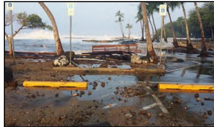
(d) January 2015. Parking lot during storm conditions. Waves can be seen overtopping main breakwater, resulting in flooding of parking lot.
