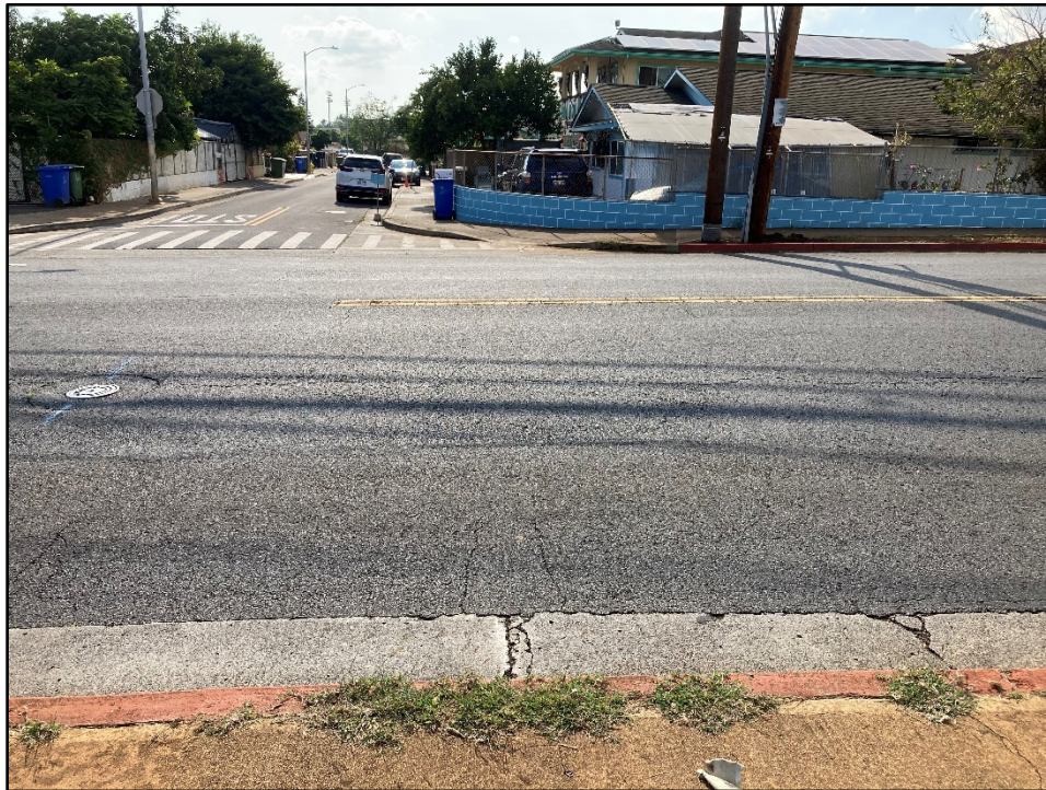
Figure 35. Photo F: General view of indicated Mahoe Street portion of the southwest project area (near the intersection with Hapapa Street at upper left), view to southwest
