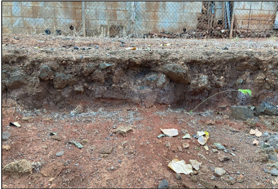
Figure 49. Photo T: View of an exposed face of the narrow terrace on the extreme north edge of the AAES campus, near the north corner of the campus (outside the present project areas), possibly showing a former plantation railroad bed, seemingly constructed of basalt boulder and cobbles, view to northwest
