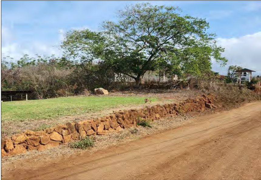
Figure 59. SIHP Site TS-06 retaining wall, view to the northeast.
