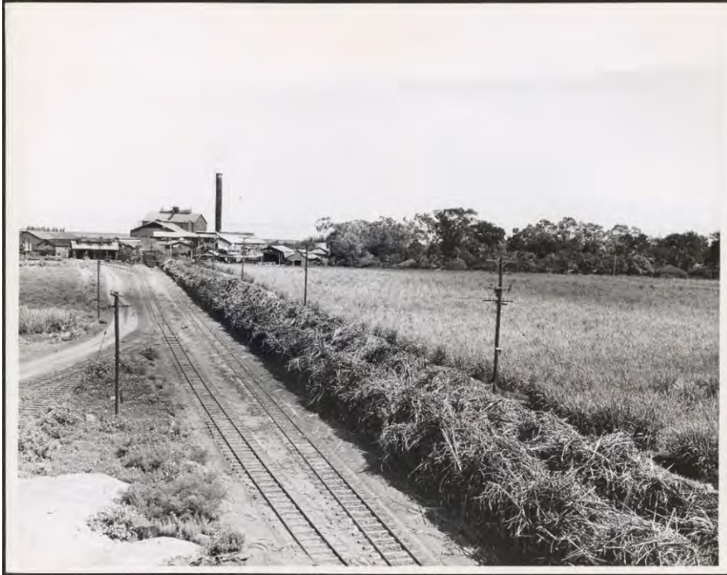
Figure 19. Photograph showing the railroad track leading to the Waiialua Sugar Mill.
