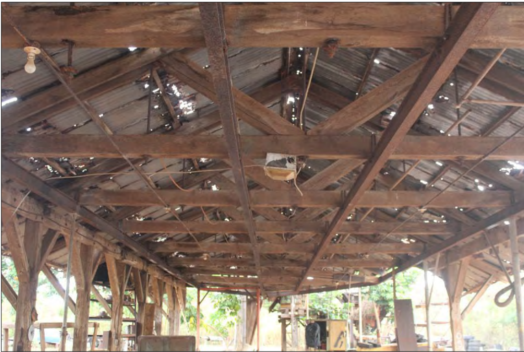
Figure 54. SIHP Site TS-02 wooden trusses on perimeter beams.
