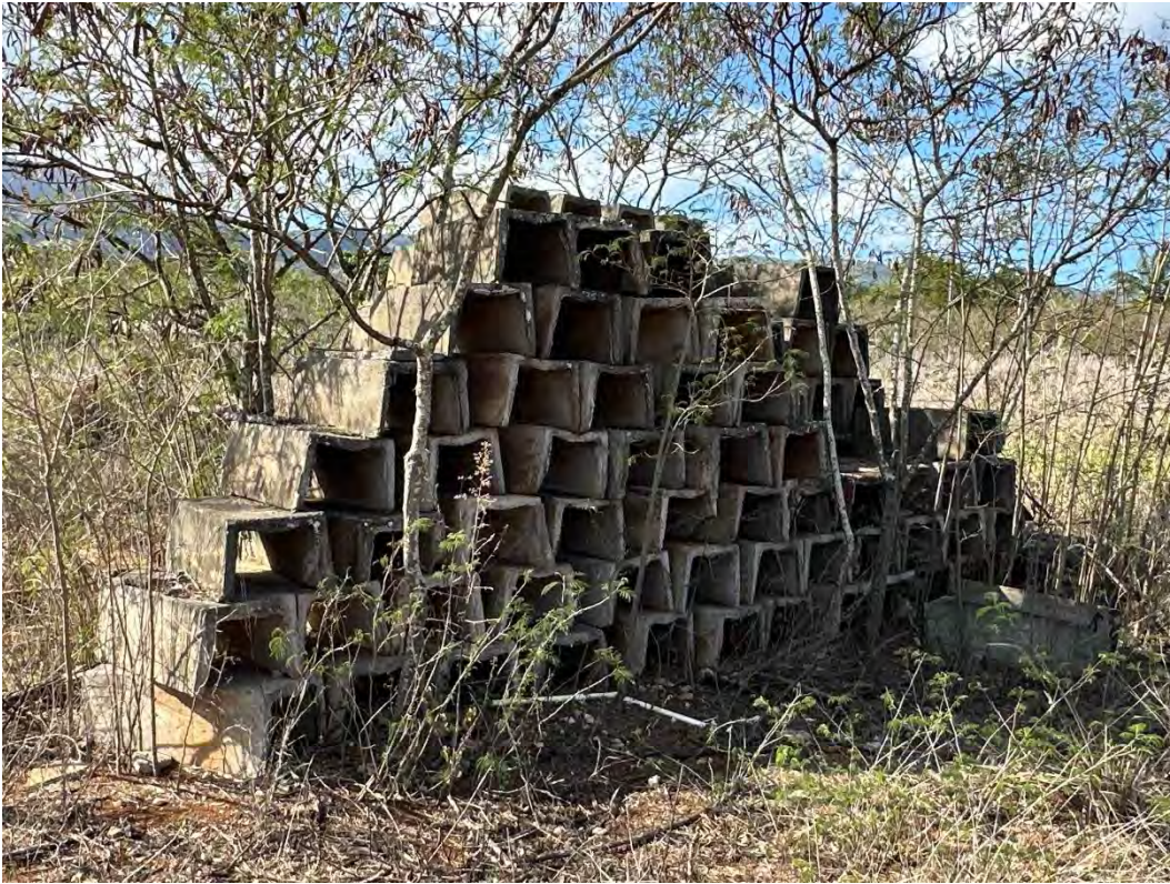
Figure 56. SIHP Site TS-02 piled flume segments located to the south of the concrete facility, view to the north.
