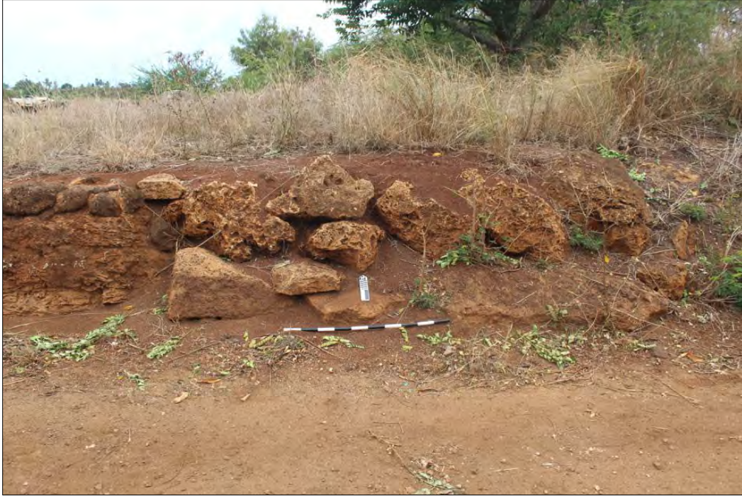
Figure 60. SIHP Site TS-06 eastern end of retaining wall, view to the north.
