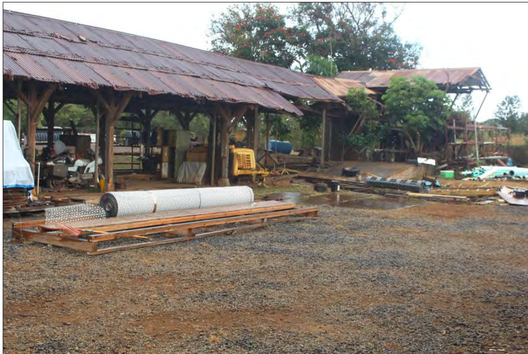
Figure 45. SIHP Site TS-02 roof junction, view to the north.
