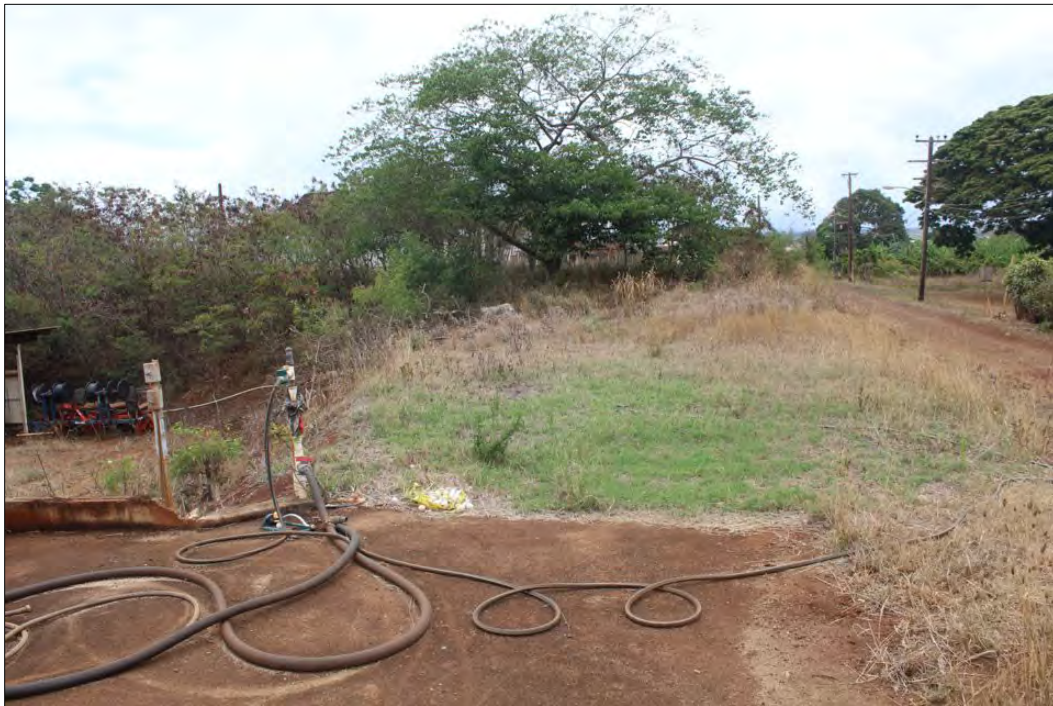
Figure 63. Current retained area north of wall, view to the east.
