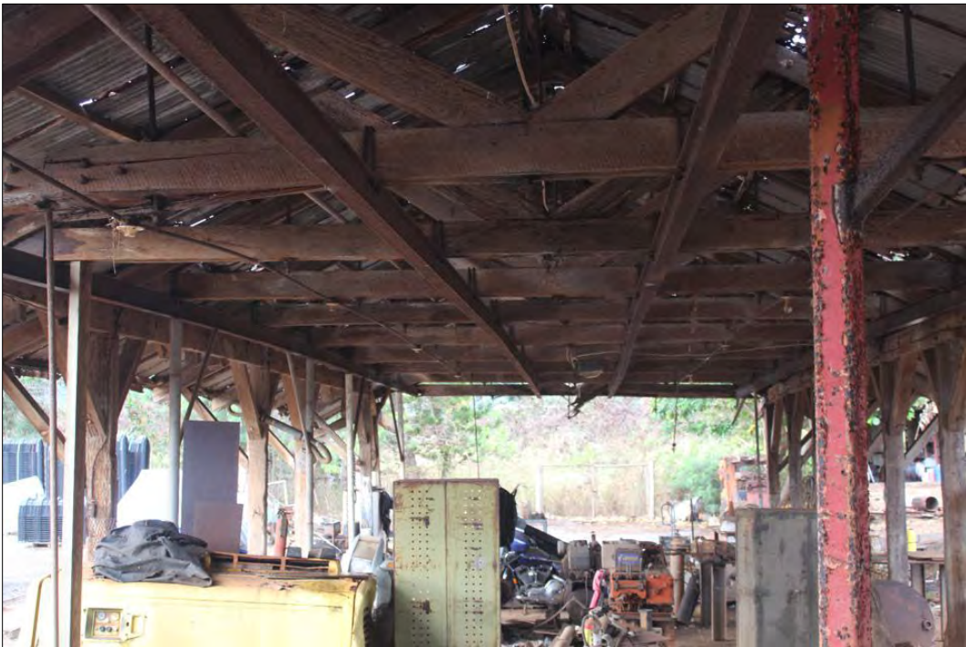
Figure 47. SIHP Site TS-02 metal bracing inside of wooden posts, view to the south.
