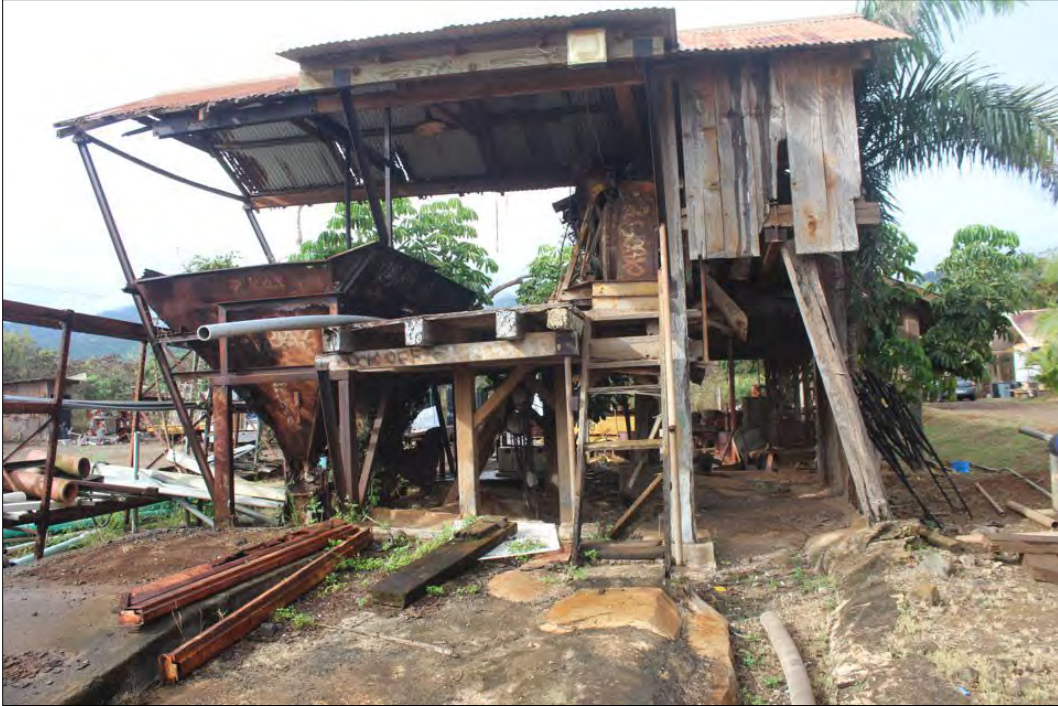
Figure 44. SIHP Site TS-02 attached structure, view to the southwest.
