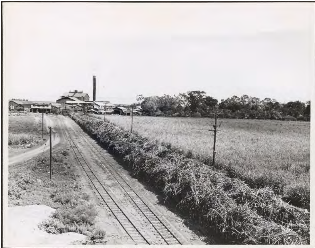
Figure 19. Photograph showing the railroad track leading to the Waialua Sugar Mill.
