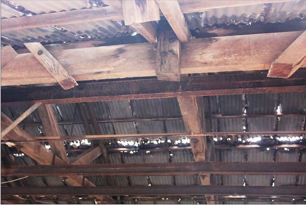
Figure 53. SIHP Site TS-02 cut and removed post and bracing.
