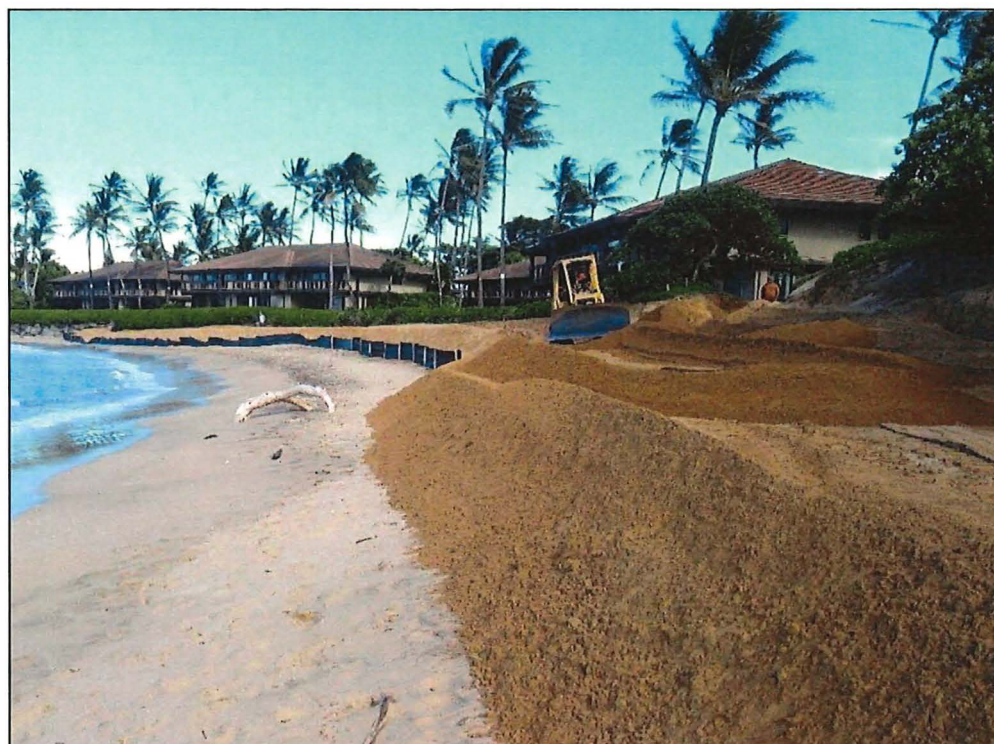
Figure 5-6 Small-scale beach nourishment at Paia, Maui (2016)
