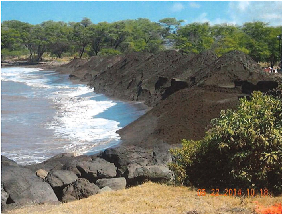
Figure 2-11: 2014 Sand placed in front of the project area.
