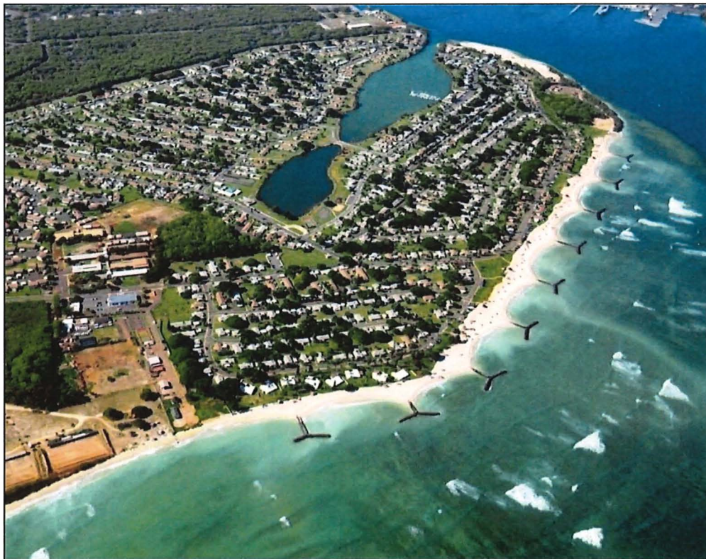
Figure 5-9 Beach stabilization with T-head groins (Iroquois Point, O‘ahu)
