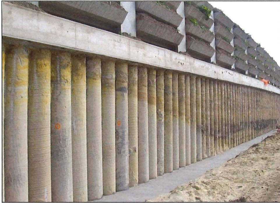
Figure 5-18 Example of a concrete secant pile wall
