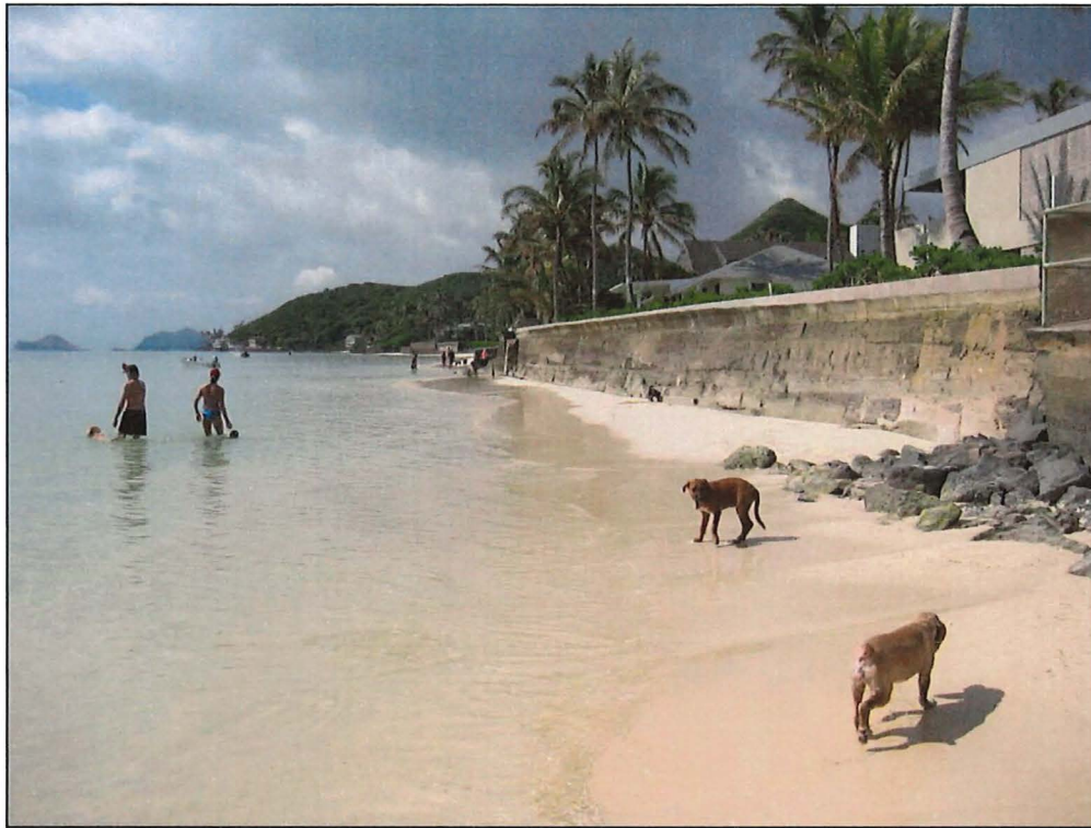
Figure 5-15 Typical concrete seawall providing hard shoreline protection
