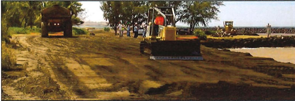
Figure 5-5: 2014 Placement of bypassed sand in front of the project area.
