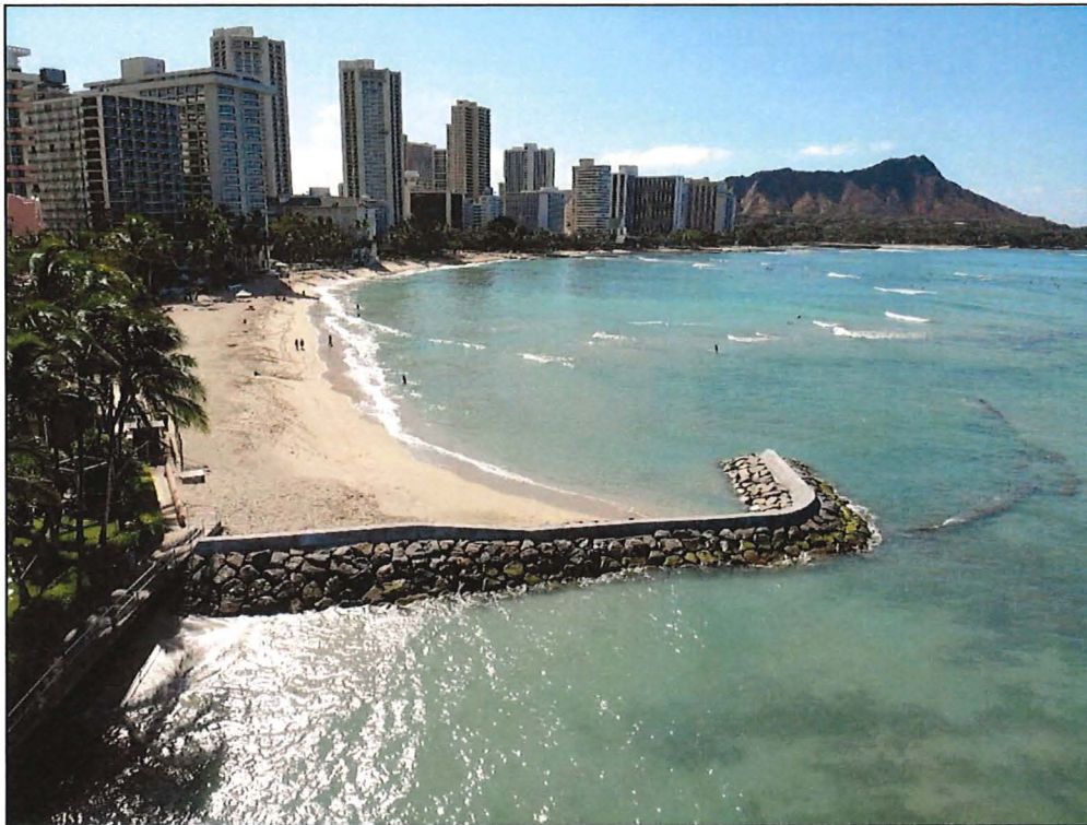
Figure 5-8 Beach stabilization with L-head groin (Waikīkī, O‘ahu)
