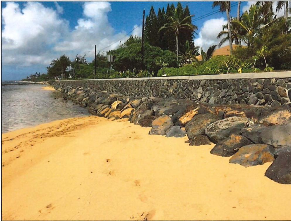
Figure 5-17 Hybrid seawall-revetment(Kapa'a, Kaua'i)
