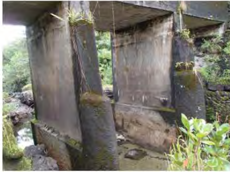
Concrete piers with rounded cutwater profile Courtesy of NOEI
