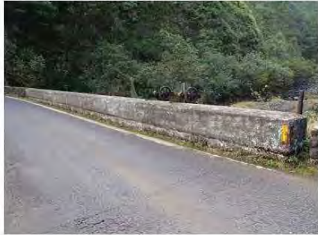
Concrete solid parapet, upstream side Courtesy of NOEI
