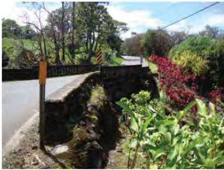
Setting of Ulaino Stream Bridge Courtesy of FAI
