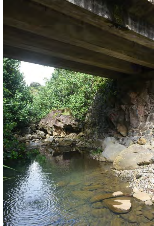
Fig. 8. Kailua Stream bridge, 685 ft., looking upstream below span.
