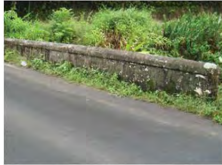
Solid concrete parapet with saddle coping, downstream side Courtesy of NOEI
