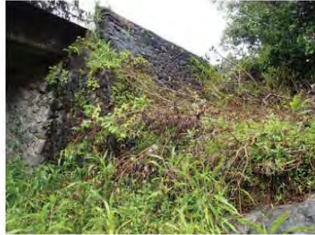
Downstream CRM wingwall, Kahului side Courtesy of NOEI
