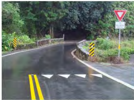
Hana approach to Makanali Stream Bridge toward Kahului Courtesy of NOEI
