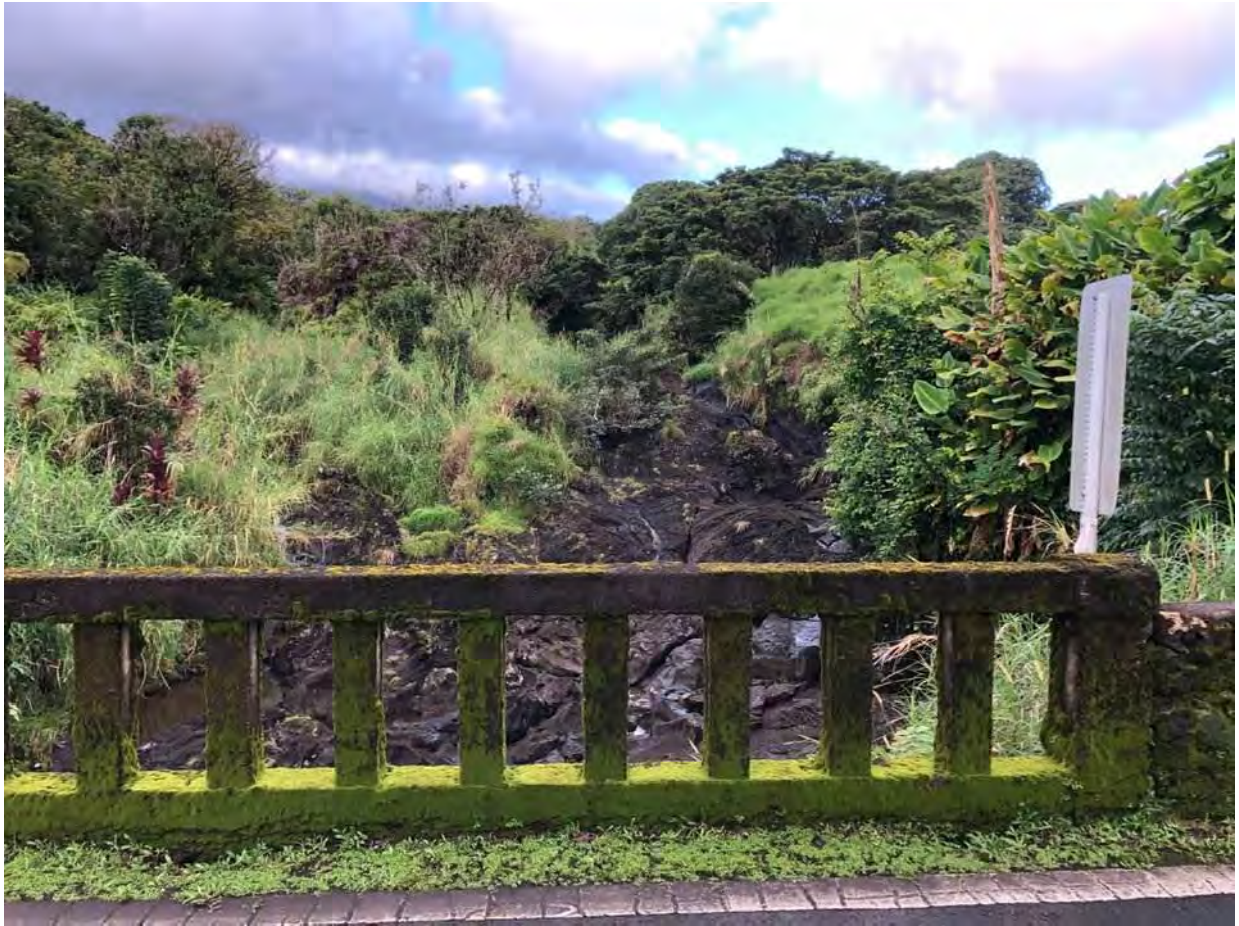
Figure 23. Mokulehua Bridge with view up the rocky stream bed.
