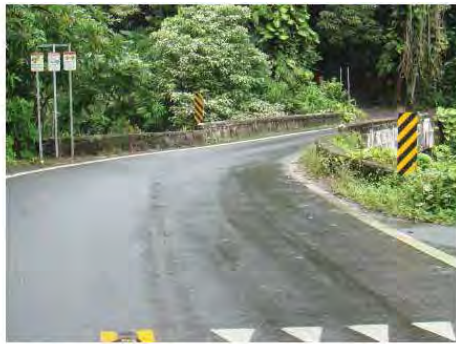
Hana approach to Puohokamoa Stream Bridge toward Kahului Courtesy of NOEI
