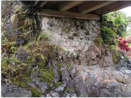
CRM abutment set on natural rock, Kahului side Courtesy of NOEI
