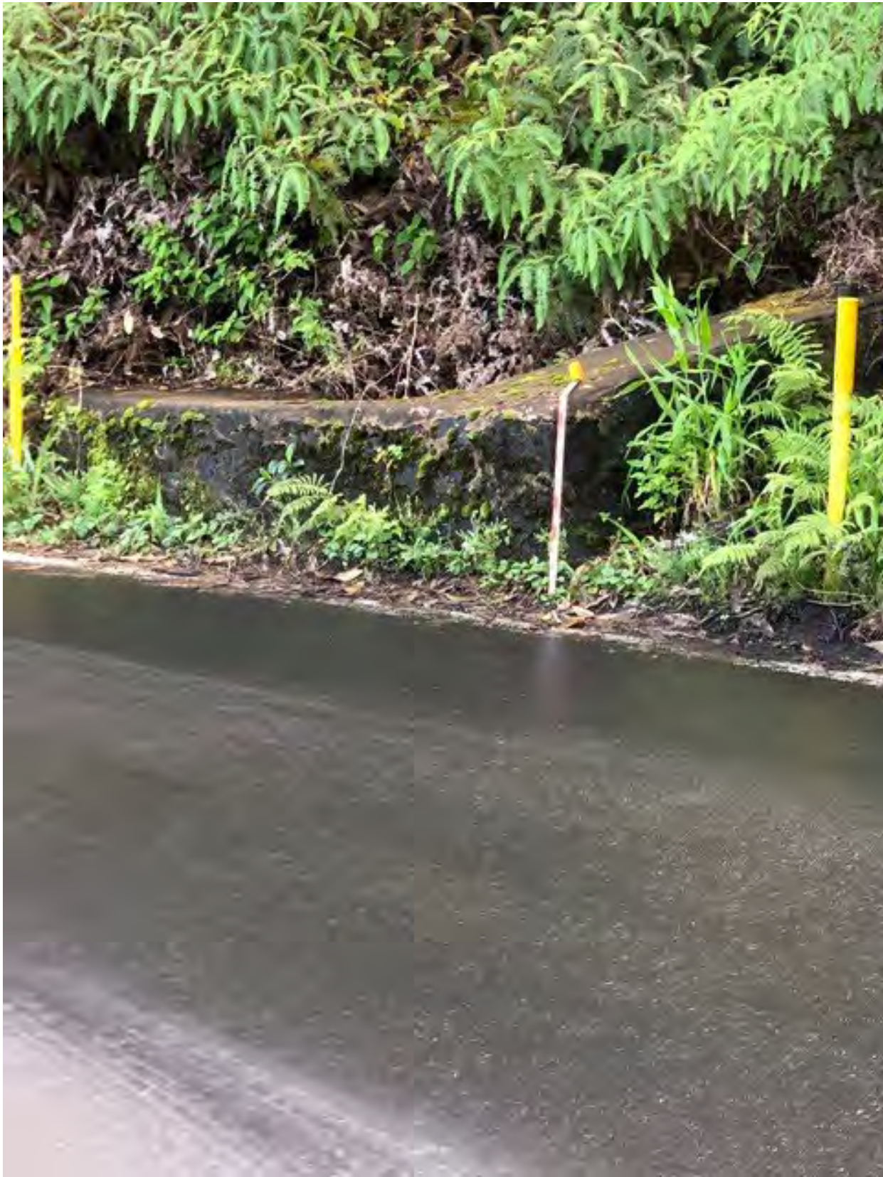
Figure 36: Photograph of Kopili`ula Stream Bridge Site, Feature 2. View to East.
