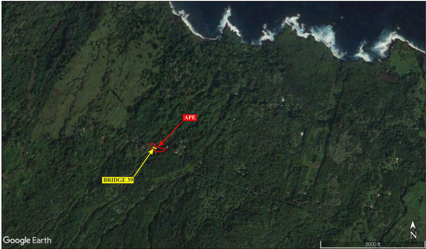
Figure 21: 2019 Google Earth Aerial Image of `Ula`ino Stream Bridge Area of Potential Effect.
