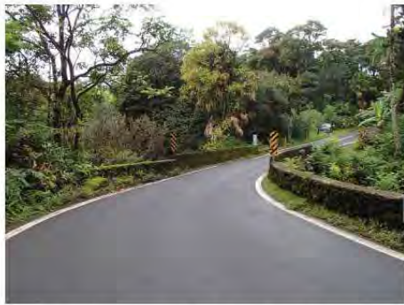
Hana approach to Mokulehua Stream Bridge toward Kahului Courtesy of NOEI
