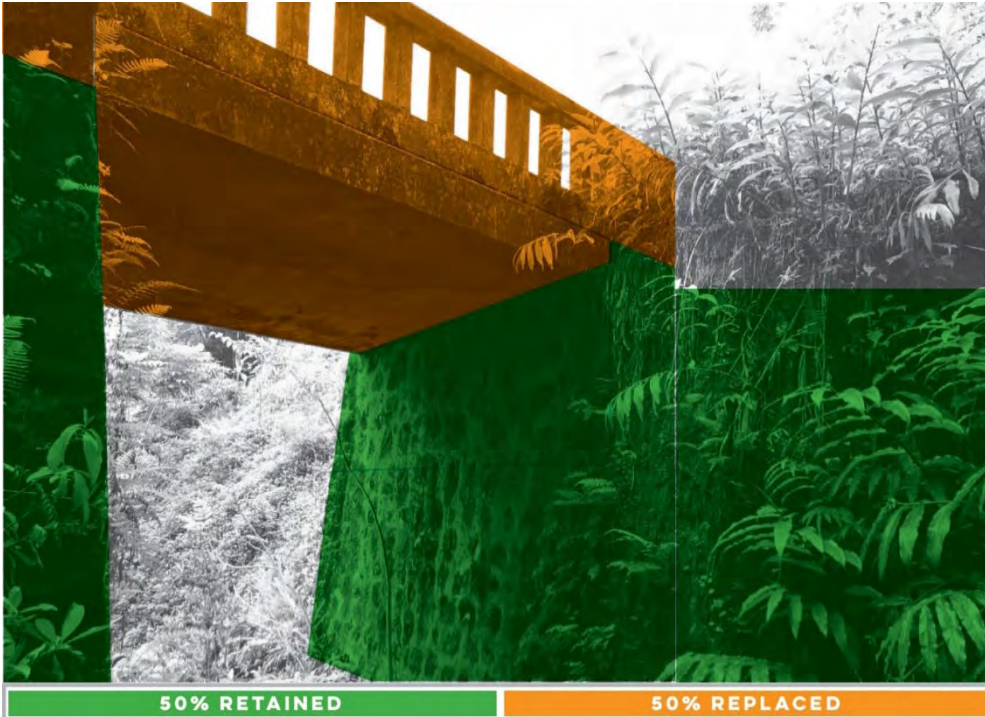
Figure 2: Makanali Stream Bridge, Overview of Effects and Rendering of the Proposed Action
