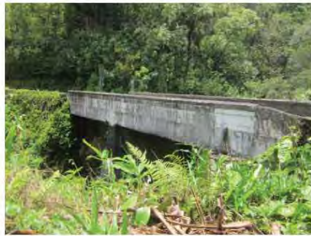
Puohokamoa Stream Bridge downstream elevation with inscription Courtesy of FAI
