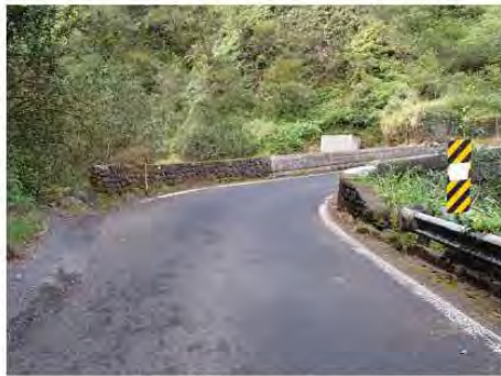
Hana approach to Kopiliula Stream Bridge toward Kahului Courtesy of NOEI
