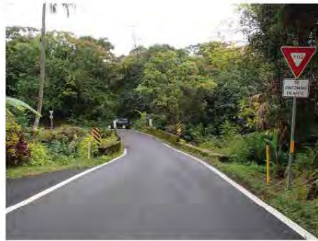
Kahului approach Mokulehua Stream Bridge toward Hana Courtesy of NOEI
