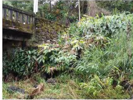
Upstream CRM wingwall, Hana side Courtesy of NOEI
