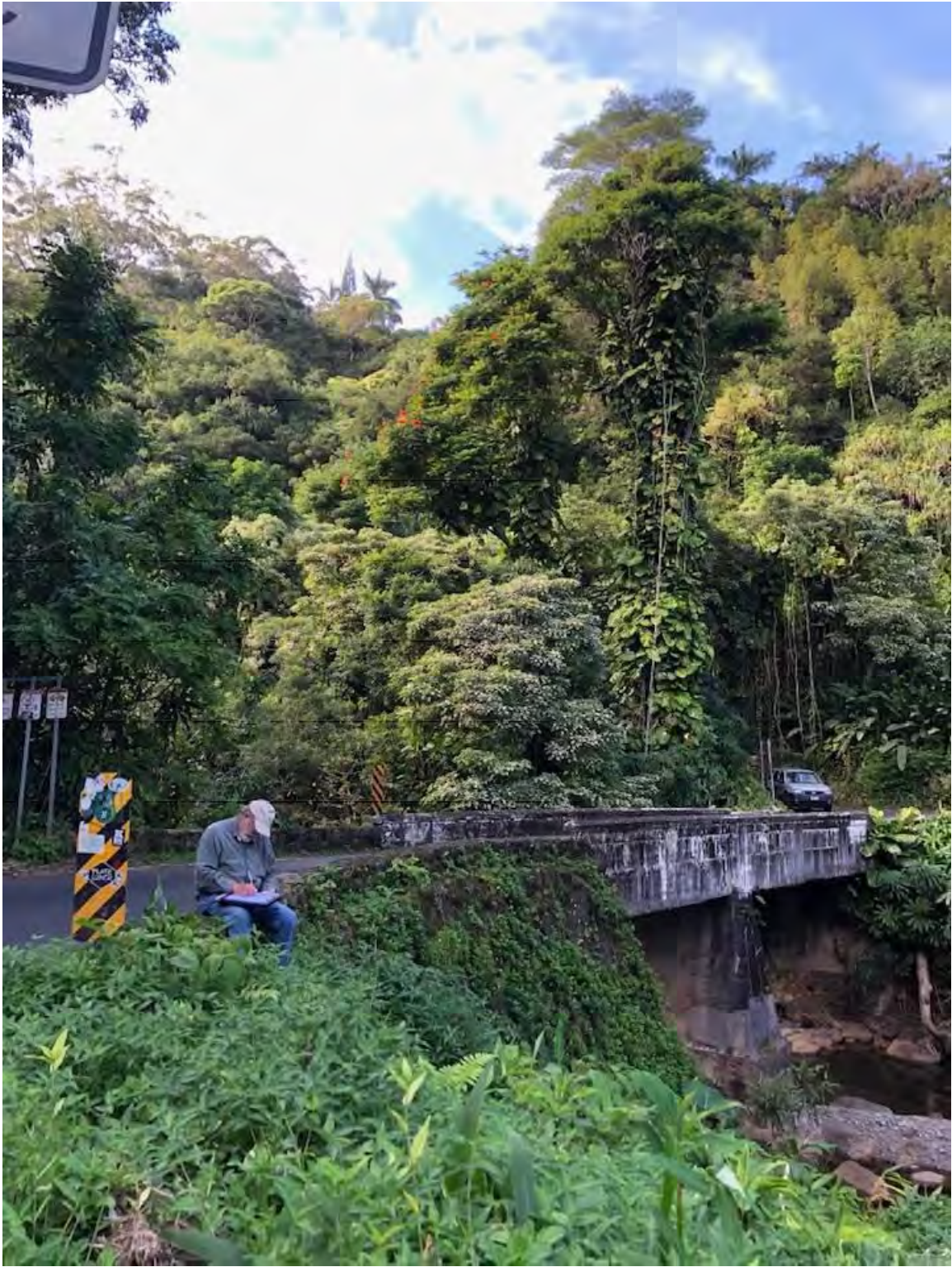
Figure 10. Puohokamo Bridge showing dense forest growth.
