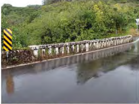
Concrete open vertical railing, upstream side Courtesy of NOEI
