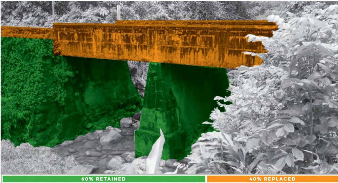
Figure 3: Puohokamoia Stream Bridge, Overview of Effects and Rendering of the Proposed Action
