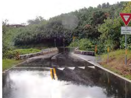
Kahului approach to Kailua Stream Bridge toward Hana Courtesy of NOEI
