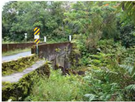
Setting of Mokulehua Stream Bridge Courtesy of NOEI
