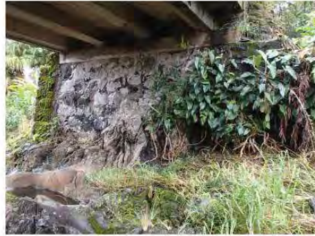
CRM abutment set on natural rock, Hana side Courtesy of NOEI
