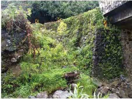
Downstream CRM wingwall, Hana side Courtesy of NOEI
