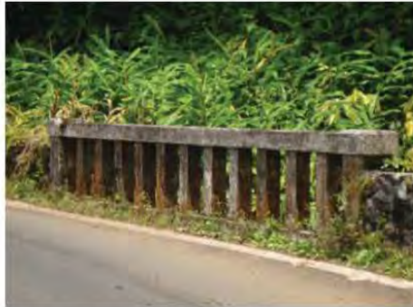
Concrete open vertical railing, upstream side Courtesy of FAI
