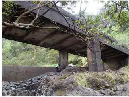
Setting of the Kopiliula Stream Bridge, downstream side Courtesy of NOEI
