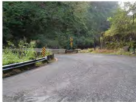
Kahului approach to Kopiliula Stream Bridge toward Hana Courtesy of NOEI
