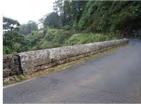
Concrete solid concrete parapet, downstream side Courtesy of NOEI
