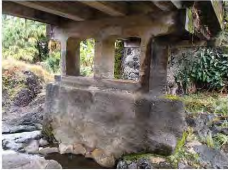
Concrete pier Courtesy of NOEI
