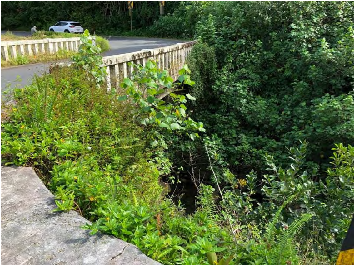
Figure 3. Kailua Bridge showing streamside vegetation.
