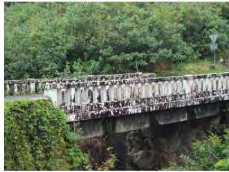
Kailua Stream Bridge downstream elevation Courtesy of FAI
