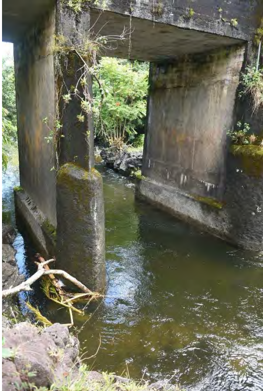
Fig. 35. Mokulehua Stream bridge, 525 ft., downstream beneath span.
