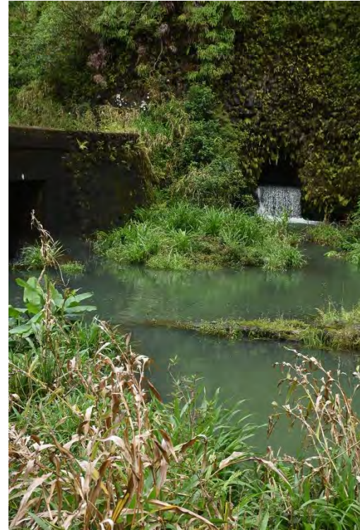
Fig. 22. Kopiliula Stream bridge, 1280 ft., ditch inflow tunnel adjacent to eastern abutment.
