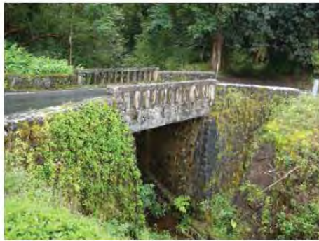
Setting of Makanali Stream Bridge Courtesy of NOEI
