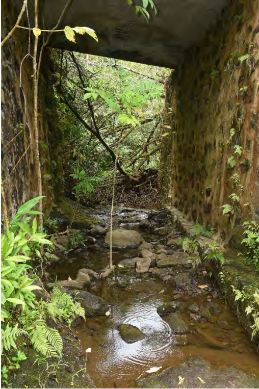
Fig. 11. Makanali Stream bridge, 695 ft., looking upstream below span.
