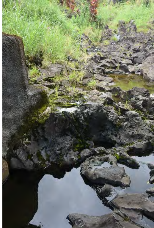
Fig. 28. Ulaino Stream bridge, 645 ft., looking upstream beneath span.
