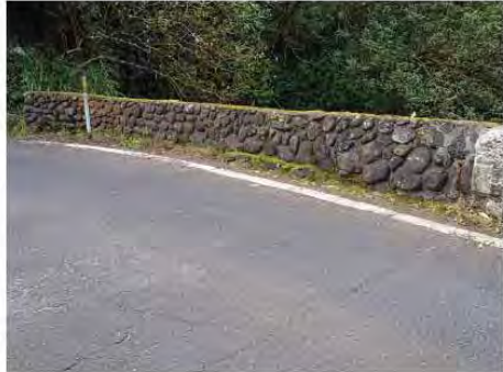
Upstream approach wall, Hana side Courtesy of NOEI
