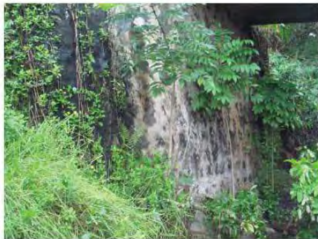
CRM abutment, Hana side Courtesy of NOEI
