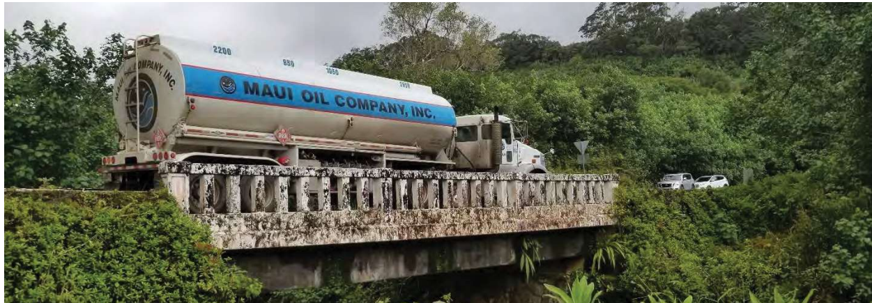
Photo 1-2. Oil Truck Crossing, Bridge #2—Kailua Stream Bridge
