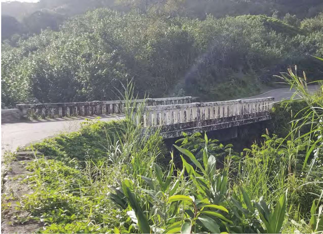
Figure 3-7. Existing Bridge #2—Kailua Stream Bridge
