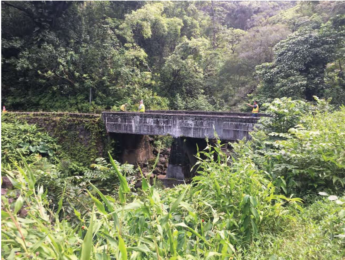
Figure 3-11. Existing Bridge #8—Puohokamoa Stream Bridge
