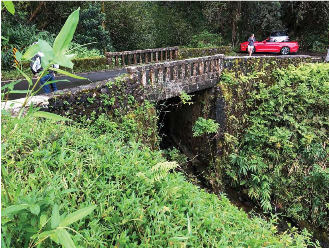
Figure 3-9. Existing Bridge #5—Makanali Stream Bridge
