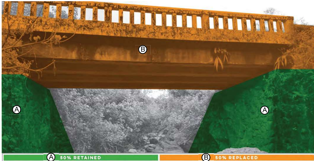
Figure 3-5. Bridge #2—Kailua Stream Bridge, Overview of Effects
