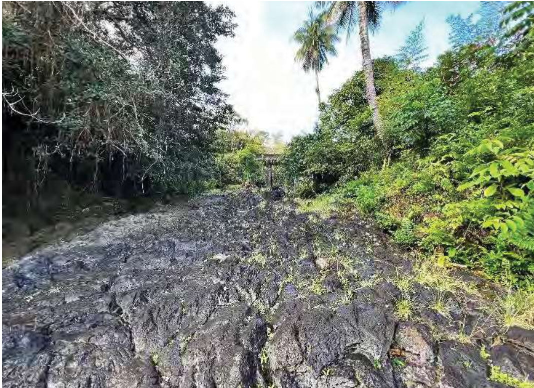
Photo 3-6. Bridge #40—Mokulehua Stream Bridge crossing the Kawakoe Stream (looking upstream from the makai side of the bridge)
