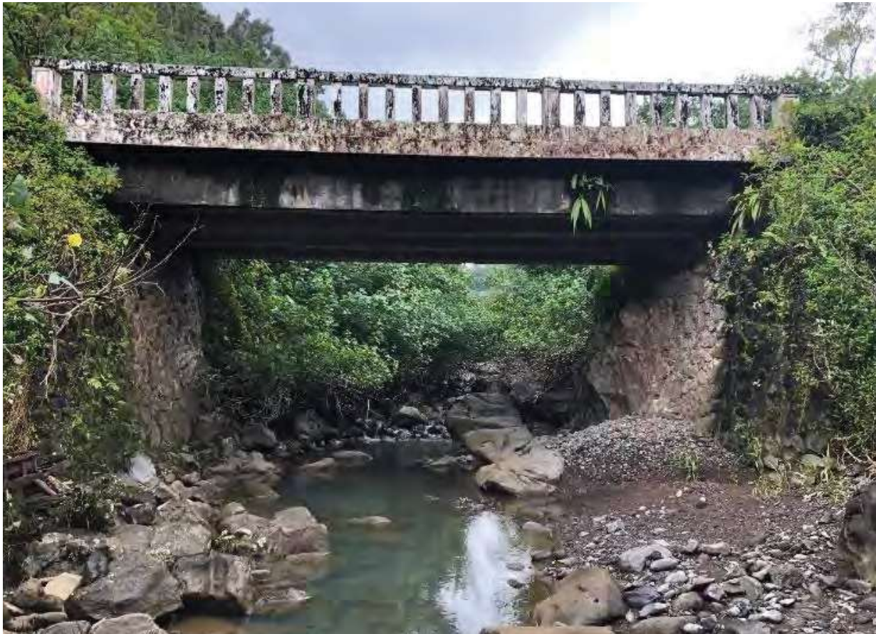
Photo 3-1. Bridge #2—Kailua Stream Bridge crossing the Kailua Stream (looking upstream from the makai side of the bridge)
