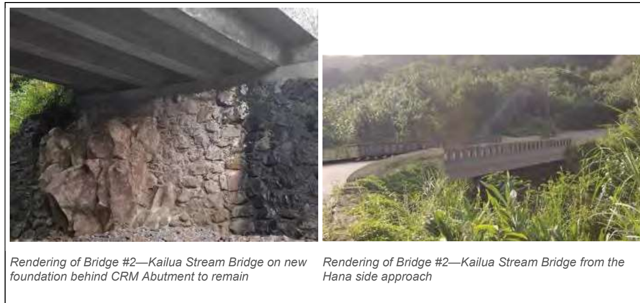
Figure 2-7. New In-Kind Superstructure at Bridge #2—Kailua Stream Bridge
