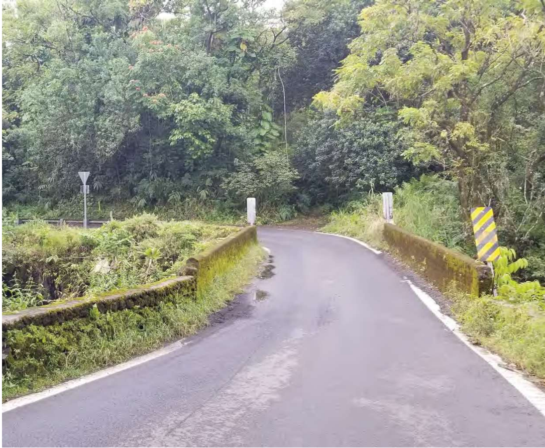
Figure 3-15. Existing Bridge #40—Mokulehua Stream Bridge
