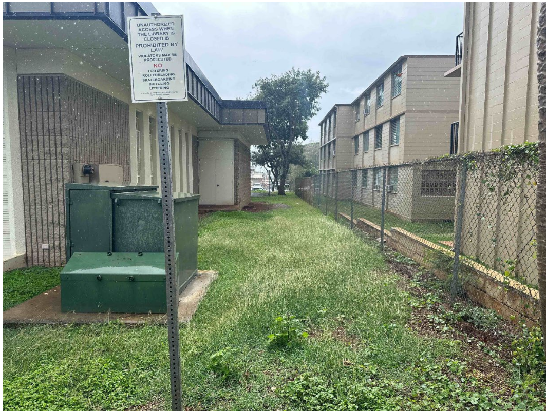
Figure 19. Western side of Pearl City Public Library, view to the south.
