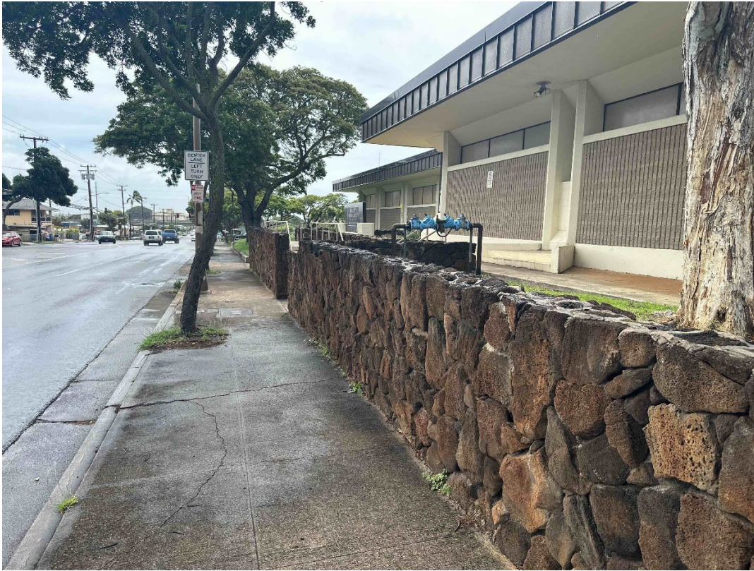
Figure 7. Eastern side of Pearl City Public Library along Waimano Home Road, view to the south.
