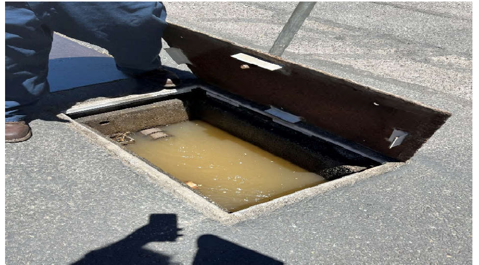
Photo 12: Interior of injection well #2.
