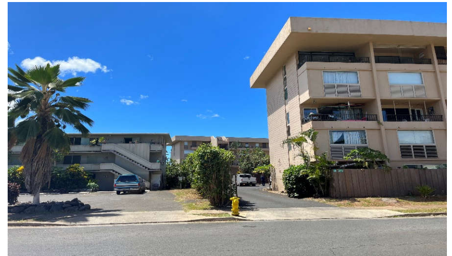
Photo 16: Driveways of Ono Vista Condominium and adjacent property – facing west.
