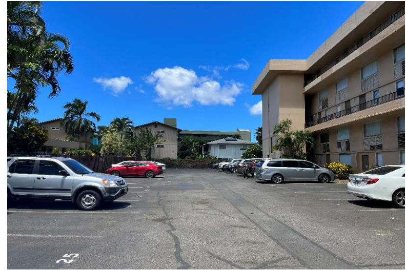
Photo 2: East parking lot facing north.
