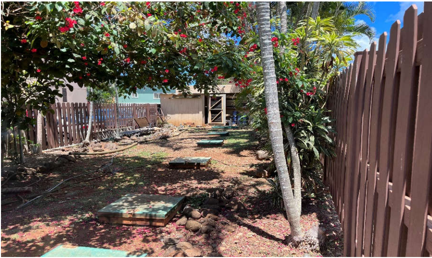
Photo 5: Inside current wastewater treatment system area - facing north.
