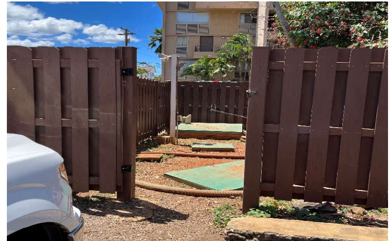
Photo 4: Gate to wastewater treatment system enclosure.
