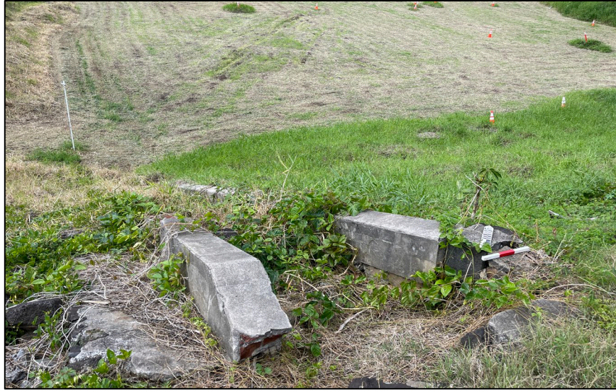
Figure 23. Feature 10 sluice, with Nu‘uanu Reservoir No. 1 below, facing north.
