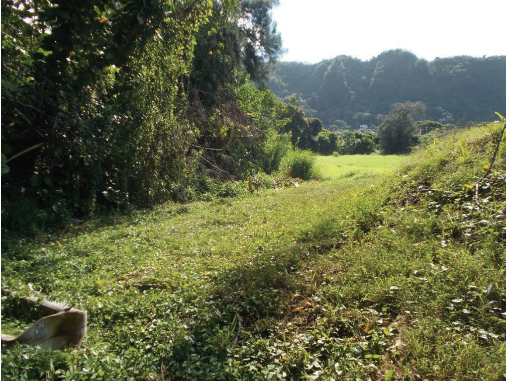
Figure 7. Spillway looking toward the impoundment in the background. View facing east.
