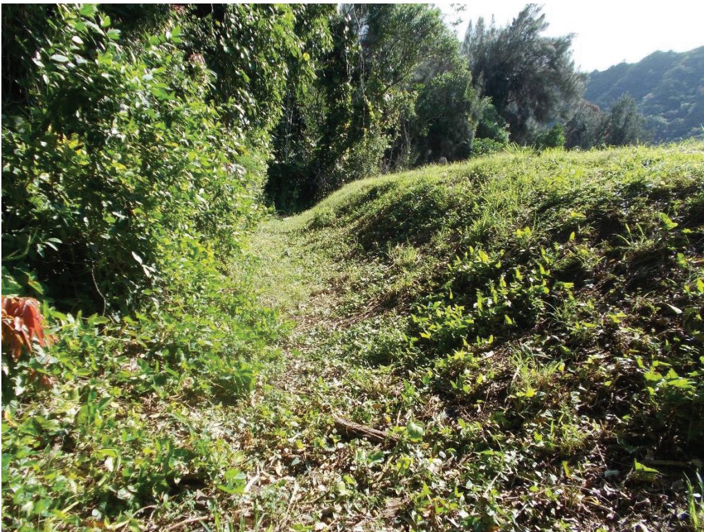
Figure 8. Spillway showing its narrow trough as it arcs around the end of the dam. View facing northeast.
