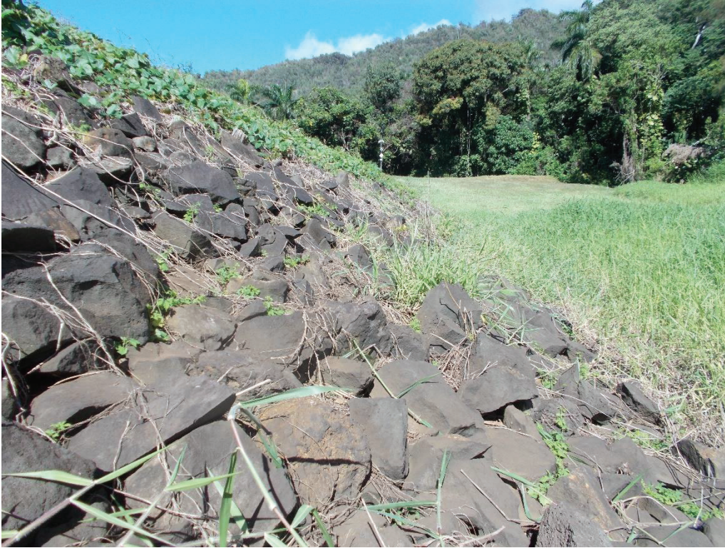
Figure 5. Lava rock face of the upstream slope. View facing northwest.
