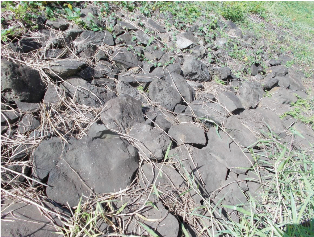
Figure 6, Lava rock face of the upstream slope. View facing southwest.
