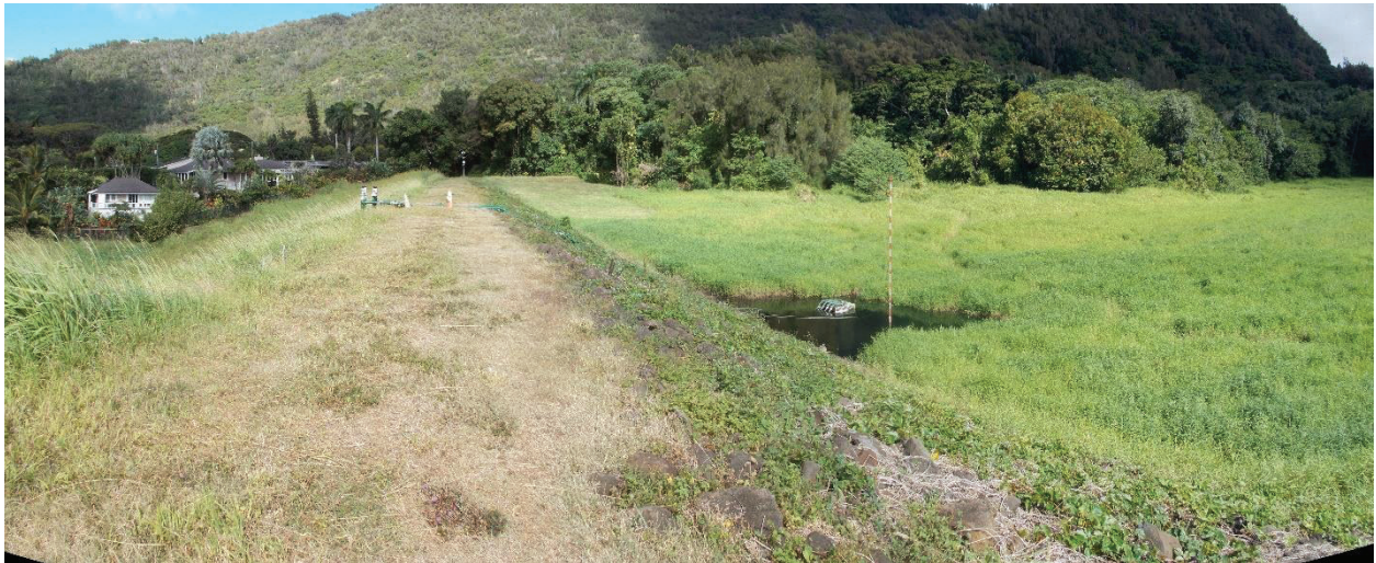
Figure 4. The crest of the dam. Note the open water of the sump and the impoundment on the right. View facing northwest.
