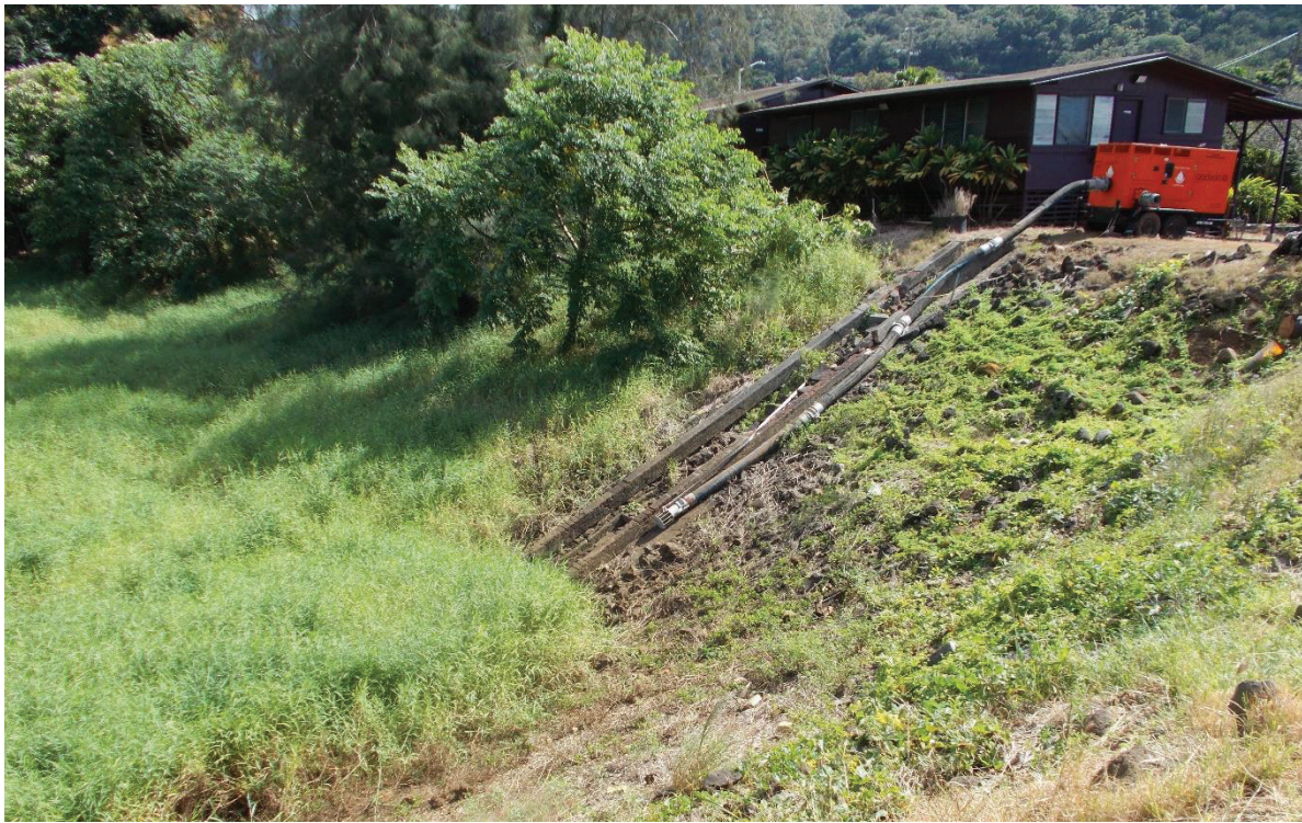
Figure 14. The brick sluice extending down the southeast side of the reservoir. The concrete sluice is out of view in the underbrush to the left. View facing east.
