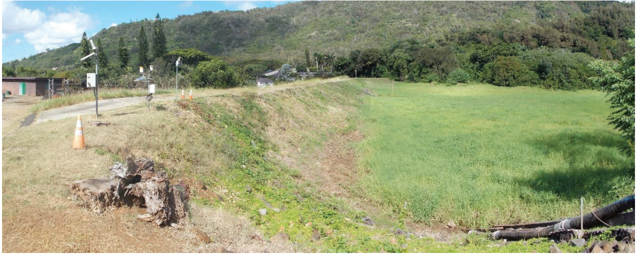
Figure 3. Overview of the Nuuanu Reservoir No. 1 Dam with a view of the upstream slope. Impoundment is on the right. View facing northwest.
