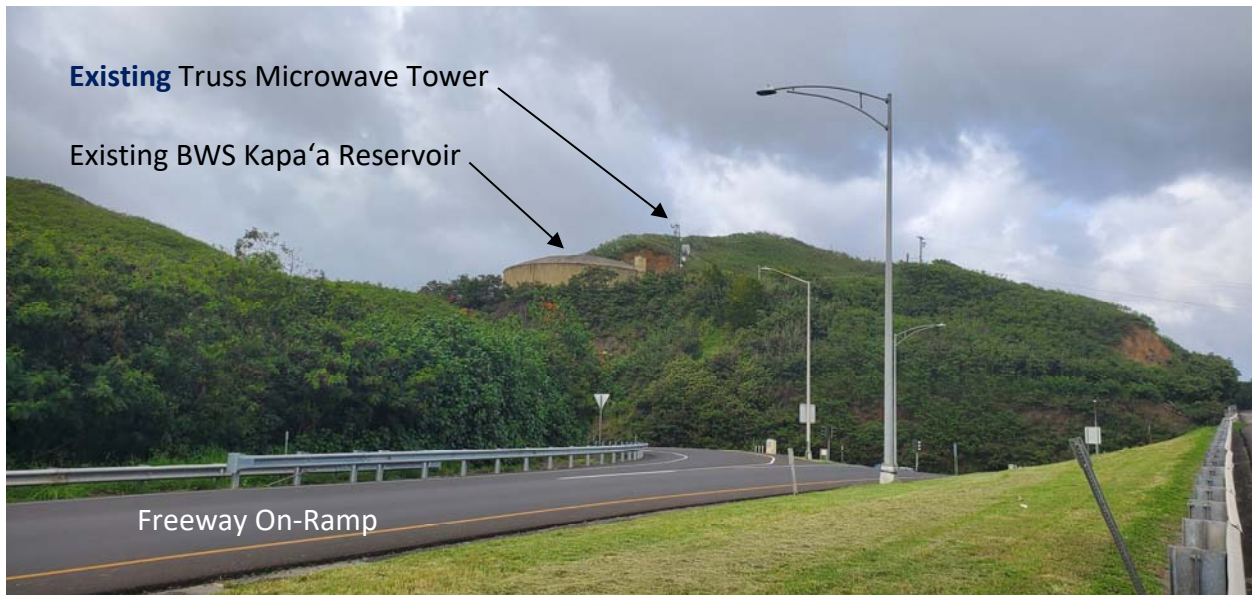
Existing View from John A. Burns (H-3) Freeway Looking North
