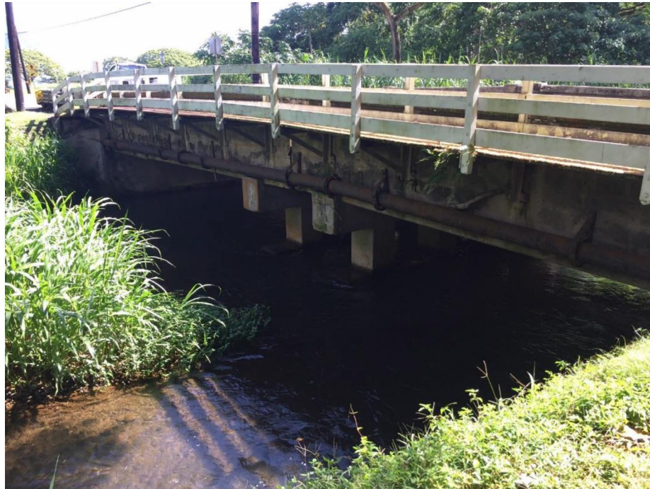
Photo 1: Mauka side of bridge, pedestrian walkway
