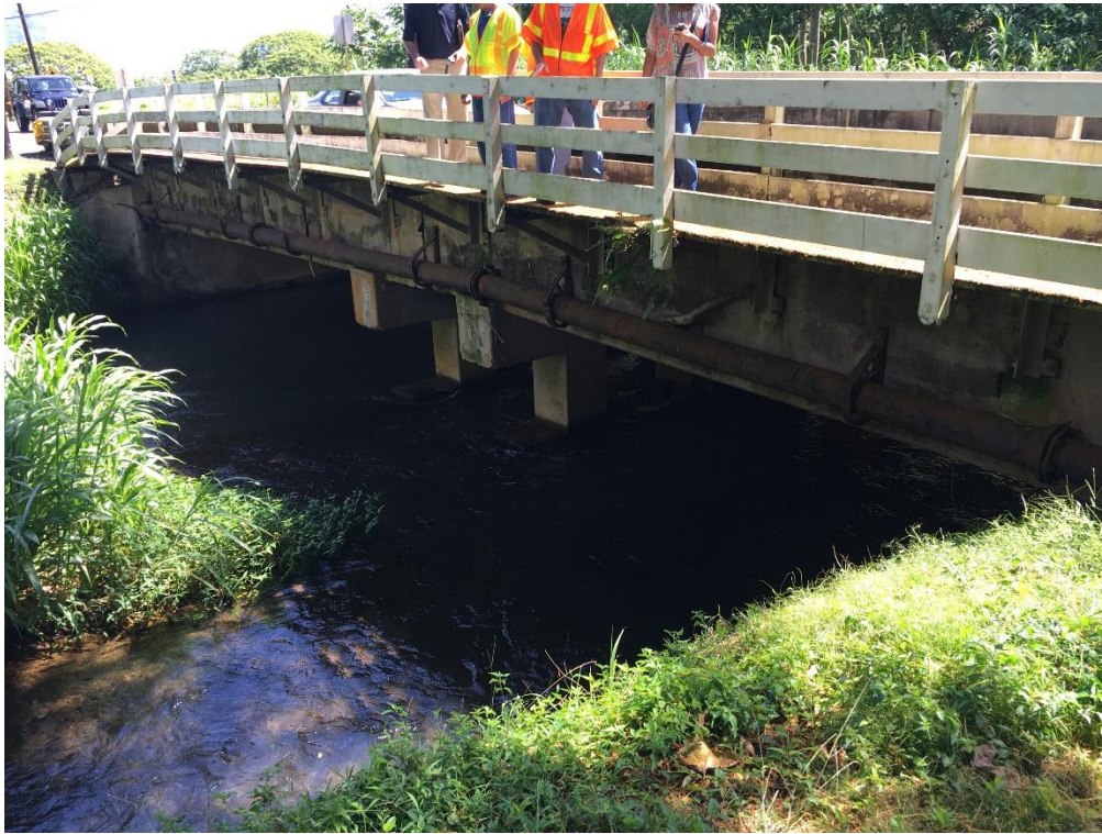
Photograph 1. Waiāhole Stream from mauka side of bridge.
