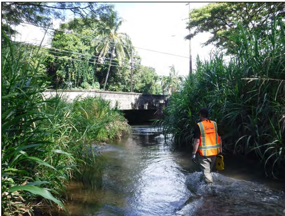
Photograph 4. Waiāhole Stream from downstream of bridge. Wetland B on the right.
