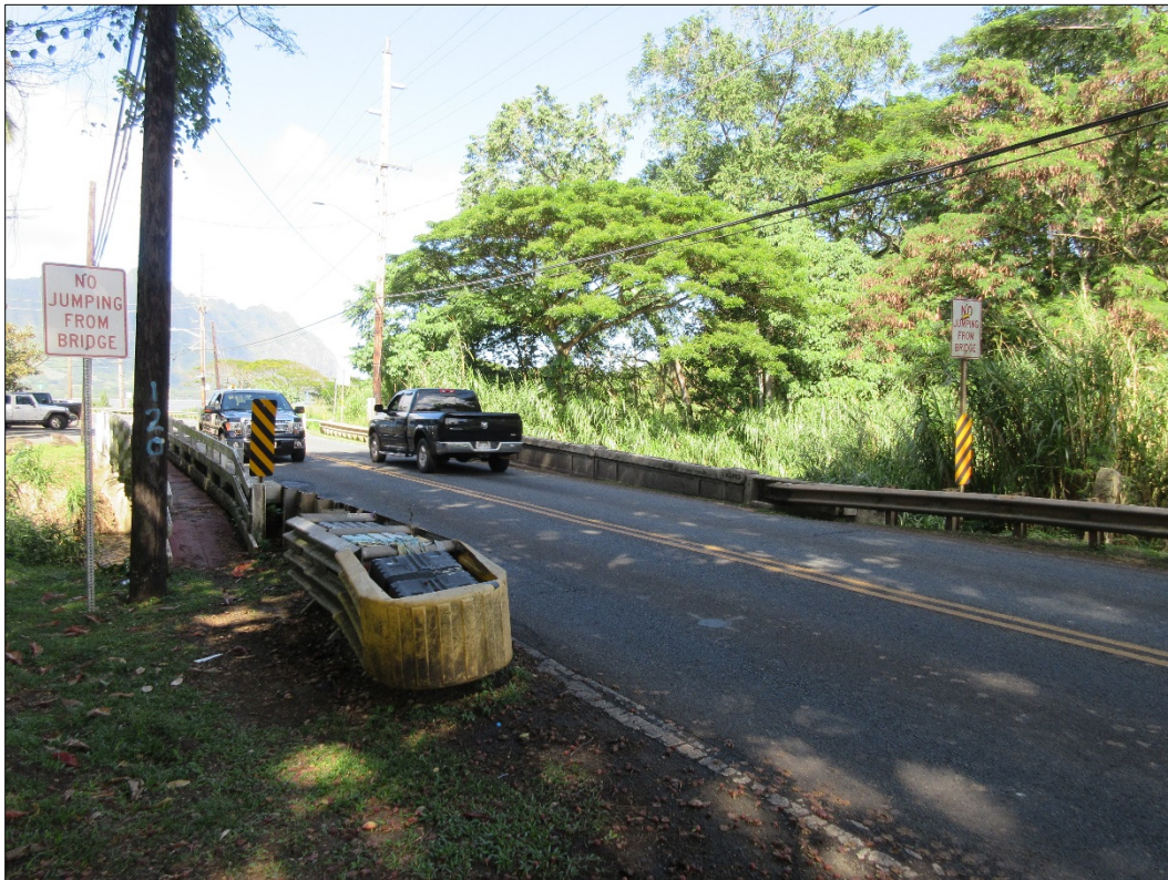
Figure 4. Waiāhole Bridge (view to the northeast).
