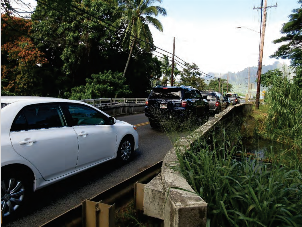
Figure 14. Makai side of Waiāhole Bridge, view to the northwest.
