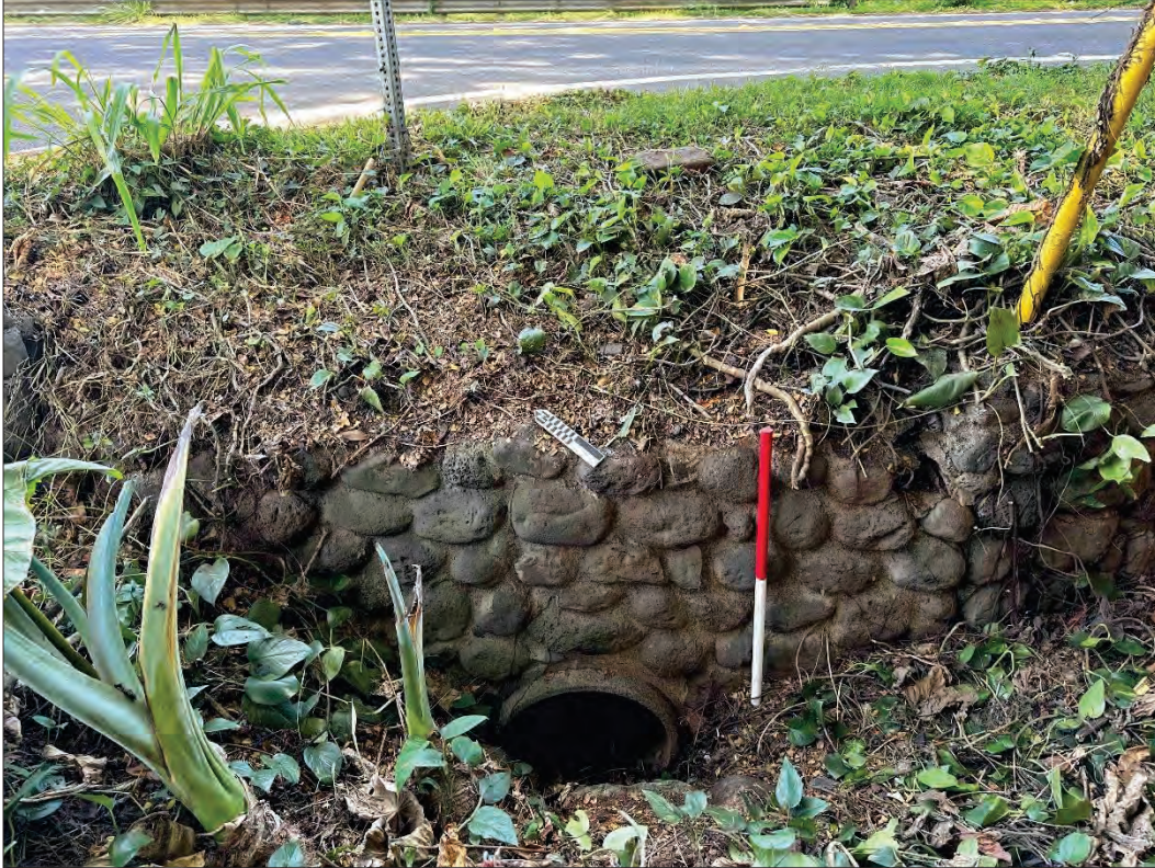
Figure 47. T-1, culvert and retaining wall. View to the northeast.
