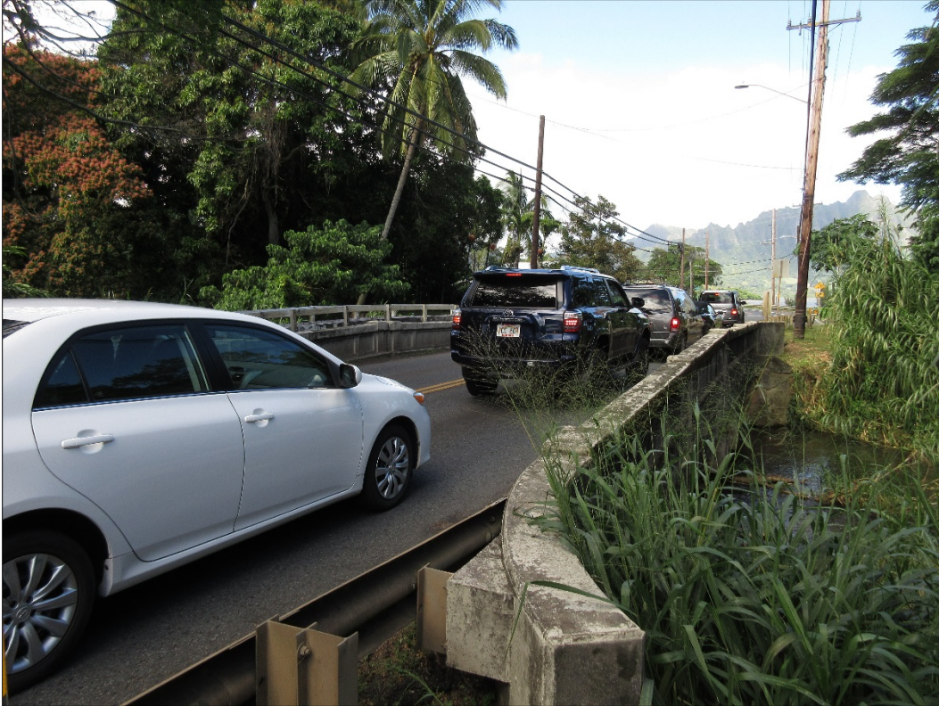
Figure 7. Makai side of Waiāhole Bridge (view to the northwest).
