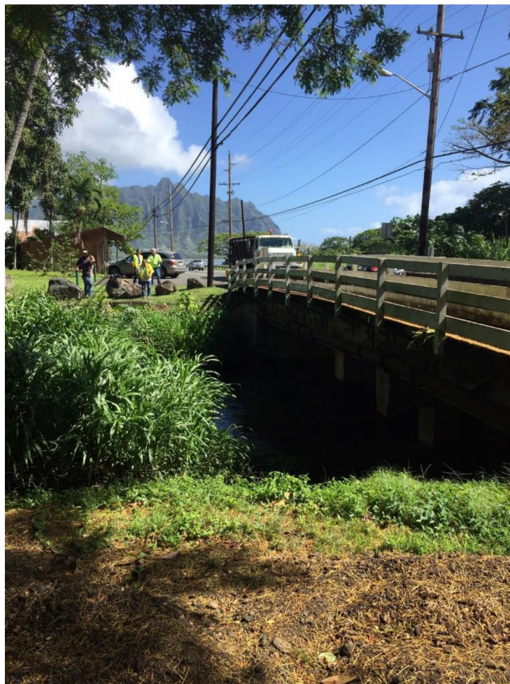
Photo 4: Mauka side of bridge, pedestrian walkway, stream bank conditions
