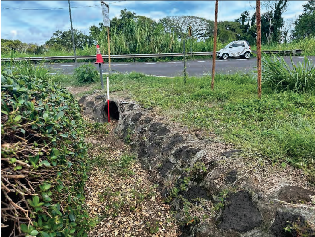
Figure 49. T-1, culvert and retaining wall. View to the east.
