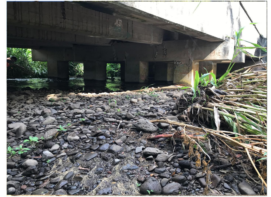
Photo 3: Waiahole Bridge center pier
