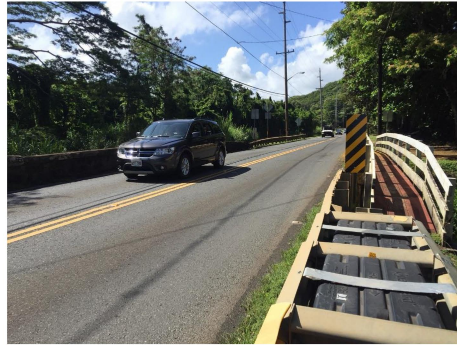
Photo 2: Bridge deck looking eastbound, pedestrian walkway
