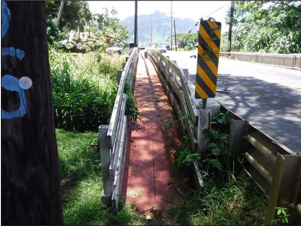
Photograph 2. Bridge and pedestrian deck.
