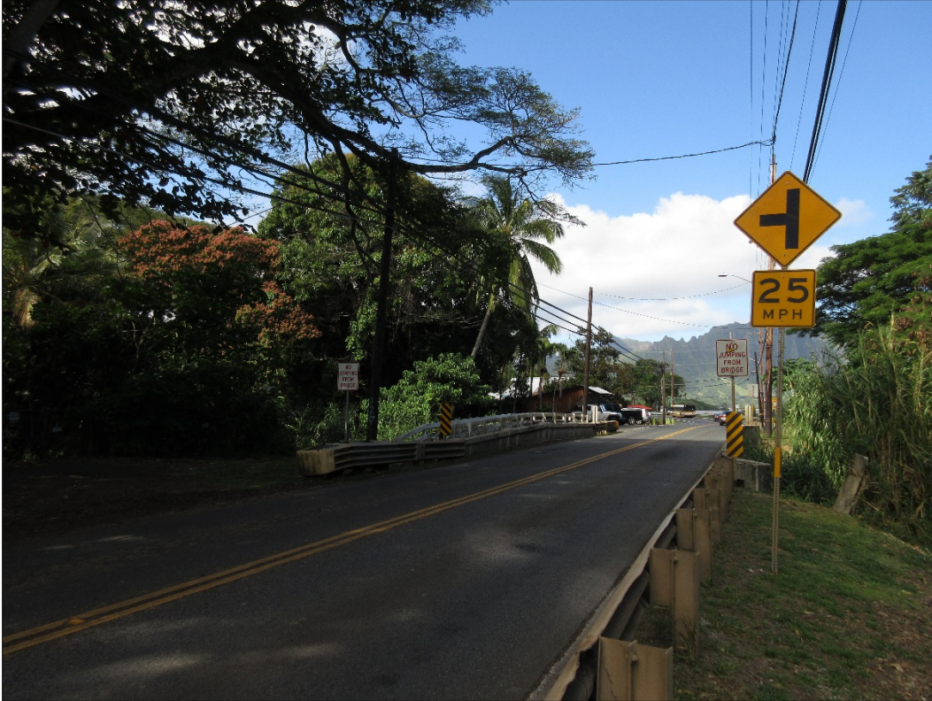
Figure 5. Kamehameha Highway and Waiāhole Bridge (view to the northwest).
