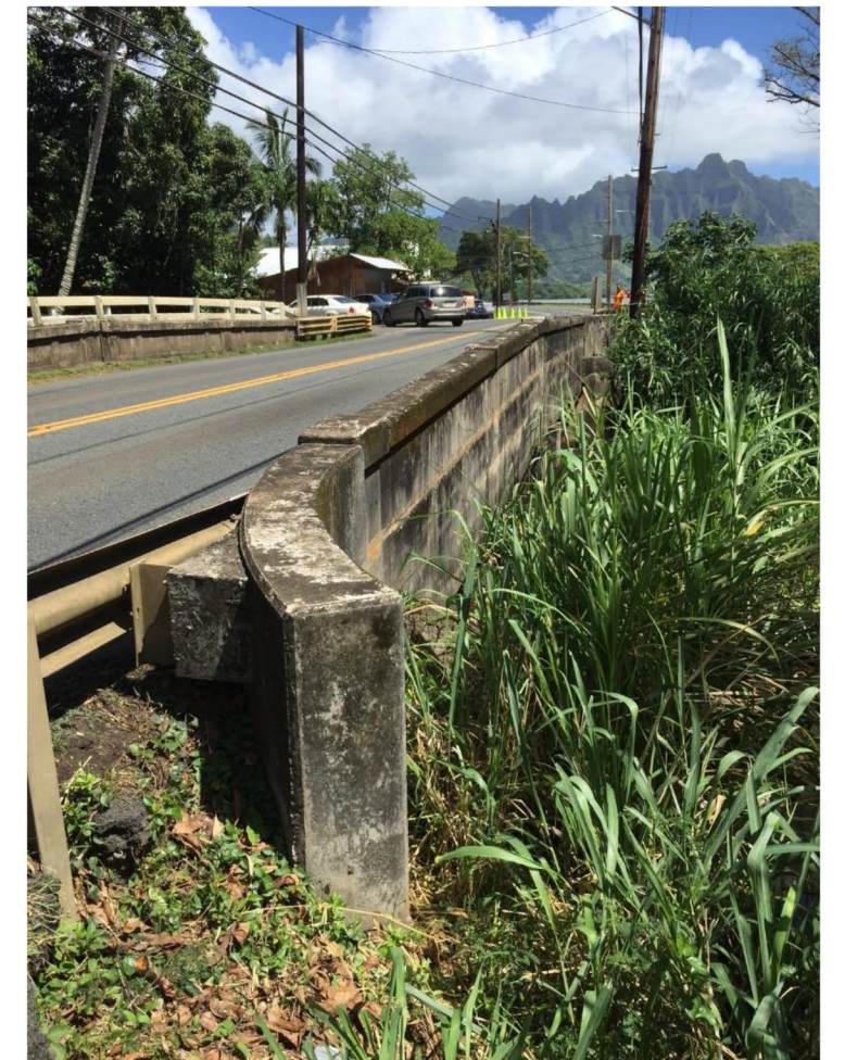
Photo 6: Makai bridge railing, looking westbound
