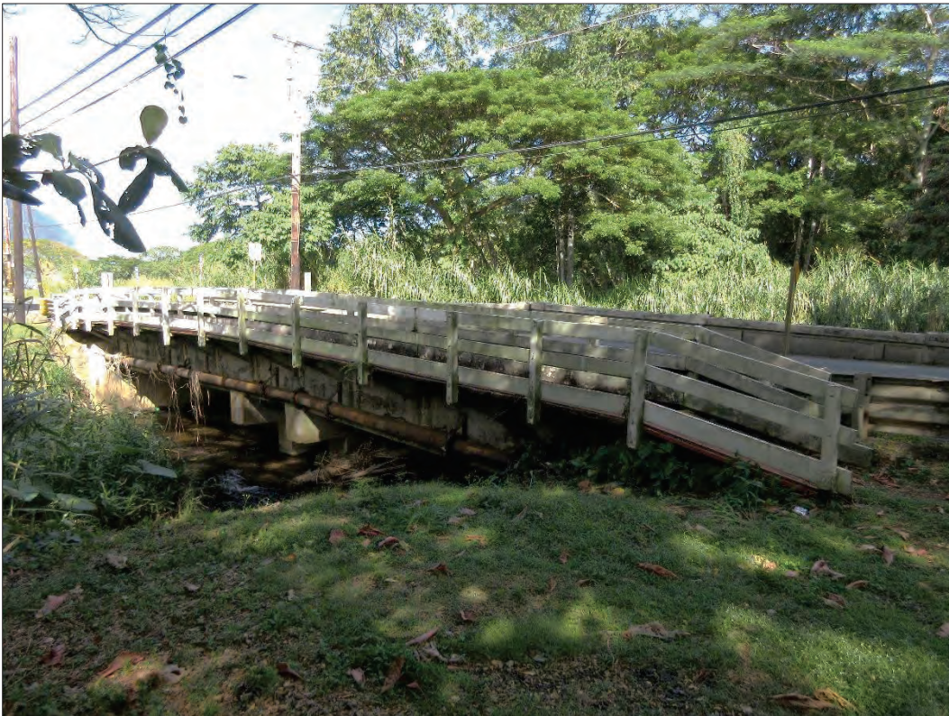
Figure 15. Mauka side of Waiāhole Bridge, view to the northeast.
