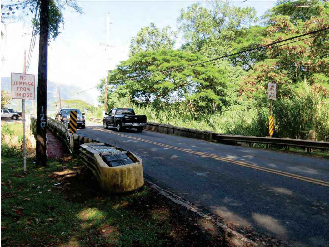
Figure 12. Waiāhole Bridge, view to the northeast.
