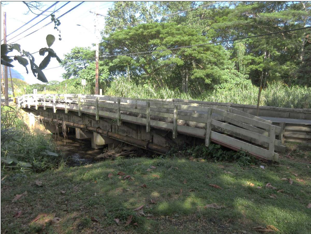
Figure 8. Mauka side of Waiāhole Bridge (view to the northeast).
