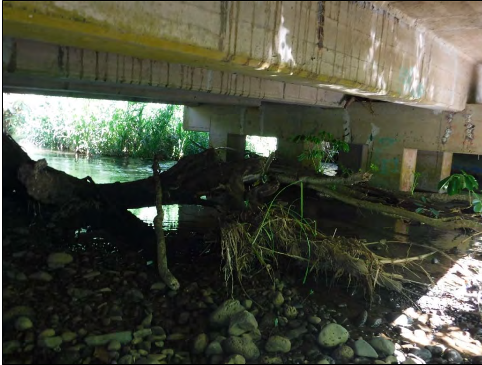
Photograph 3. Waiāhole Stream under the bridge.
