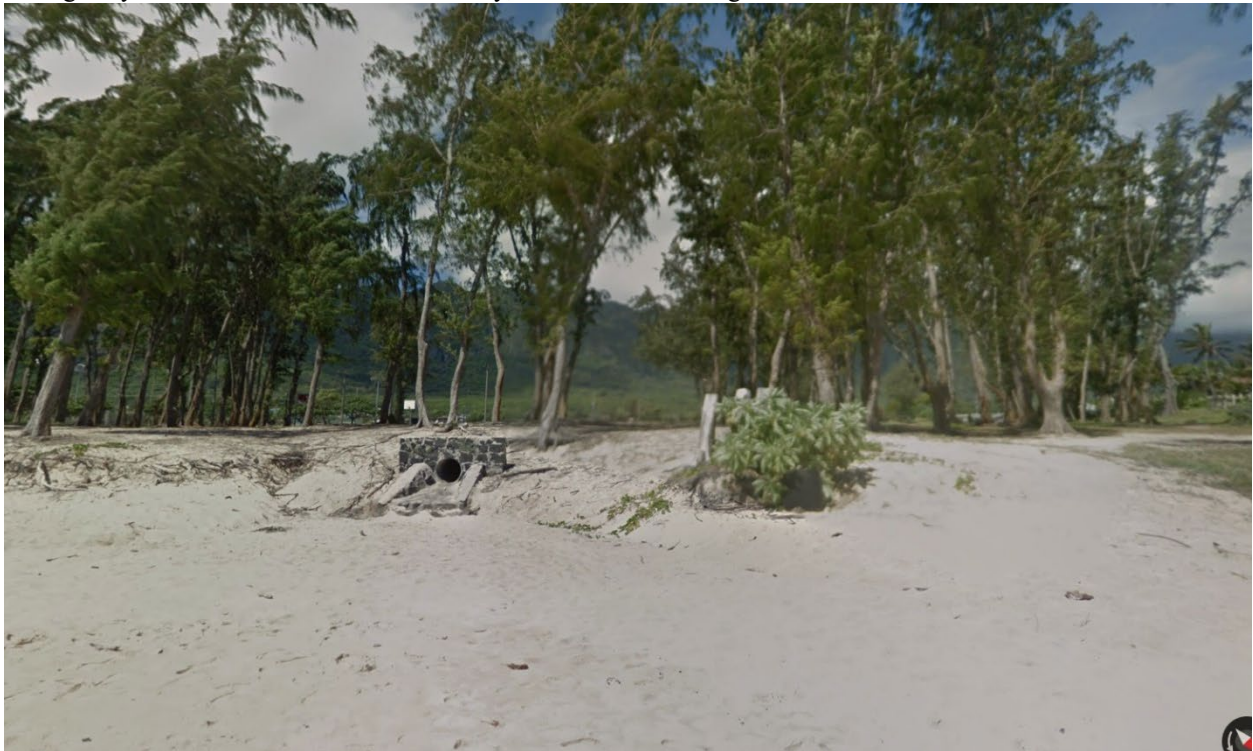
B. Highway storm drain outfall area in May, 2017. Source: Google Street View.
