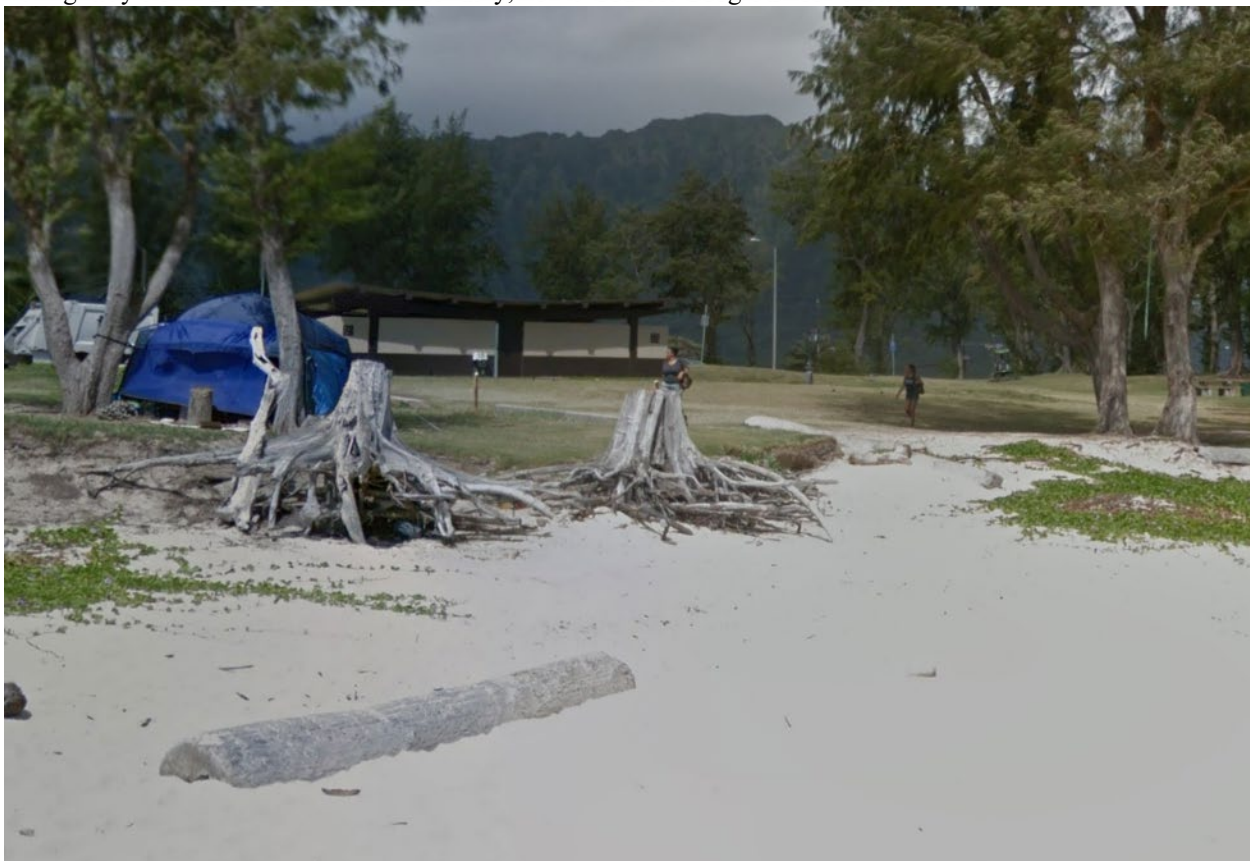
B. Highway storm drain outfall area in May, 2017. Source: Google Street View.
