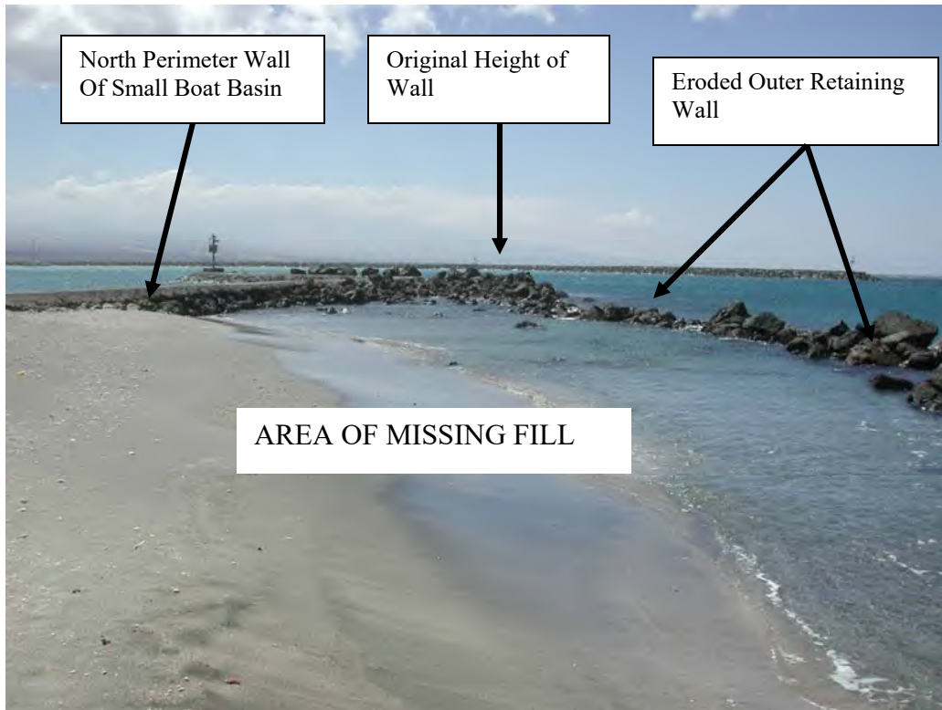
Fig. 1-Kawaihae Small Boat Basin – Photo Of Eroded Retaining Wall & Missing Fill
