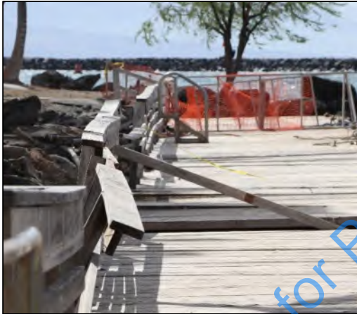
(c) January 2020. Incoming waves hit underside of marginal wooden wharf and damaged structure. Wharf was condemned.
