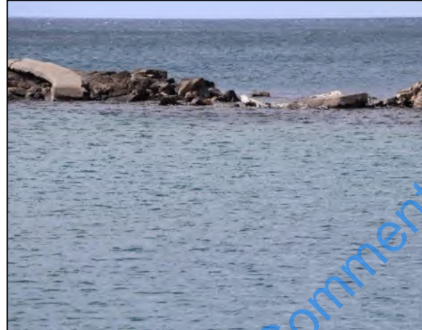
(b) January 2020. Breached section of main breakwater
