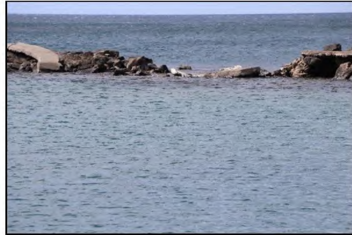
(b) January 2020. Breached section of Main Breakwater.
