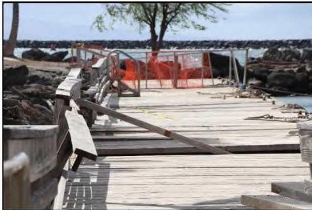
(c) January 2020. Incoming waves hit underside of marginal wooden wharf and damaged structure. Wharf was condemned.
