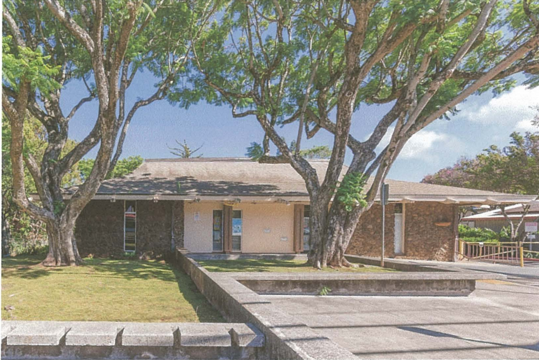
Entry to Makawao Public Library from Makawao Avenue
