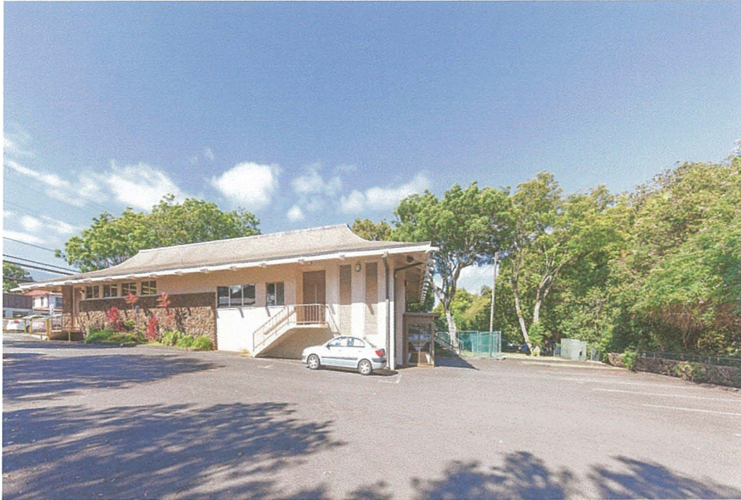
Photograph 1. South View of Building Corner Proposed for the 2-Story Addition.
