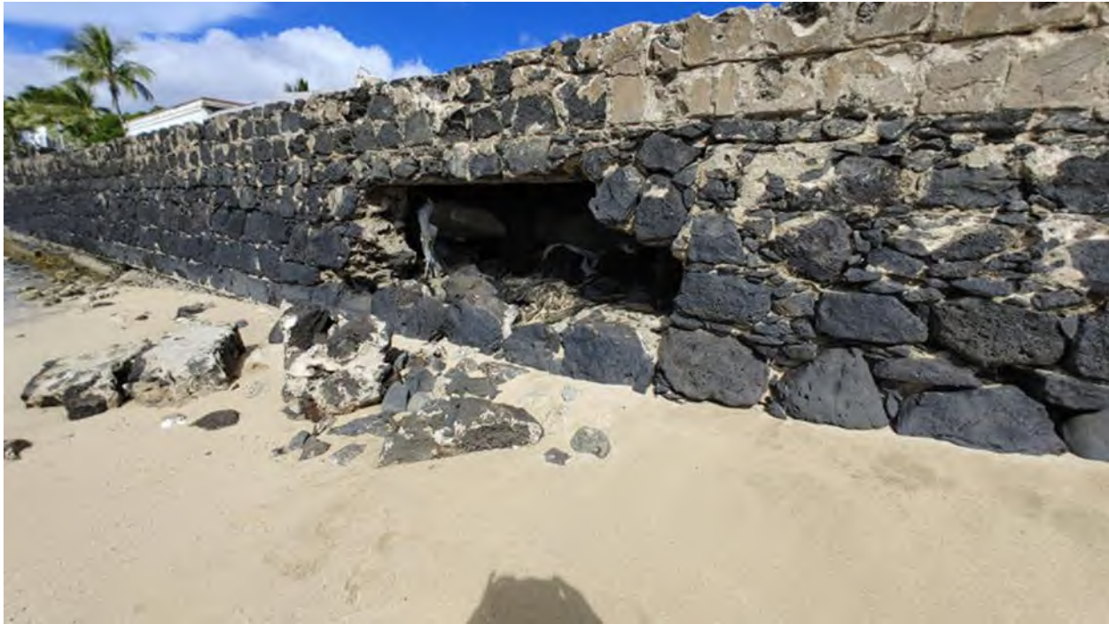
Figure 2-9: Seawall Repair
