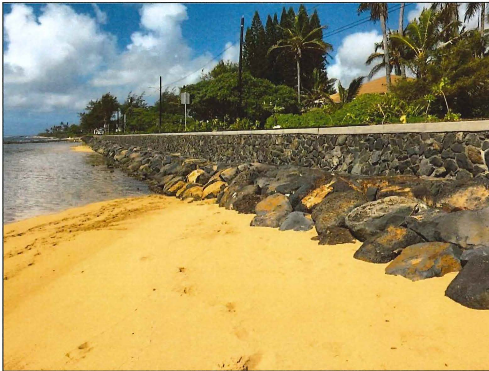
Figure 5-17 Hybrid seawall-revetment(Kapa'a, Kaua'i)
