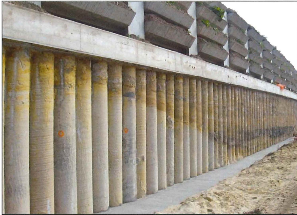
Figure 5-18 Example of a concrete secant pile wall
