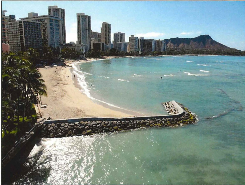
Figure 5-8 Beach stabilization with L-head groin (Waikīkī, O‘ahu)
