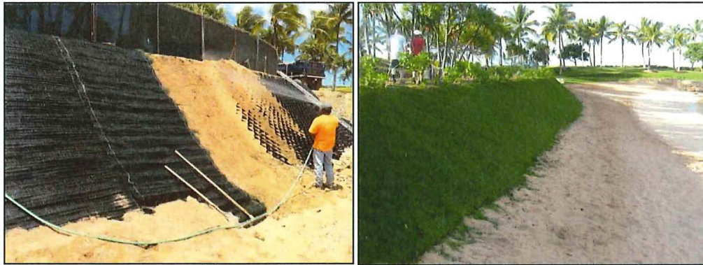
Figure 5-3 Slope stabilization with GEOCELLS and vegetation providing soft shoreline protection (Ko'olina, O'ahu)
