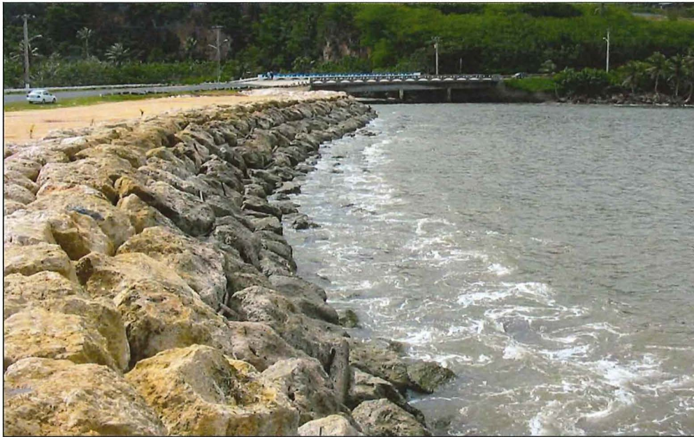
Figure 5-16 Typical rock revetment providing hard shoreline protection
