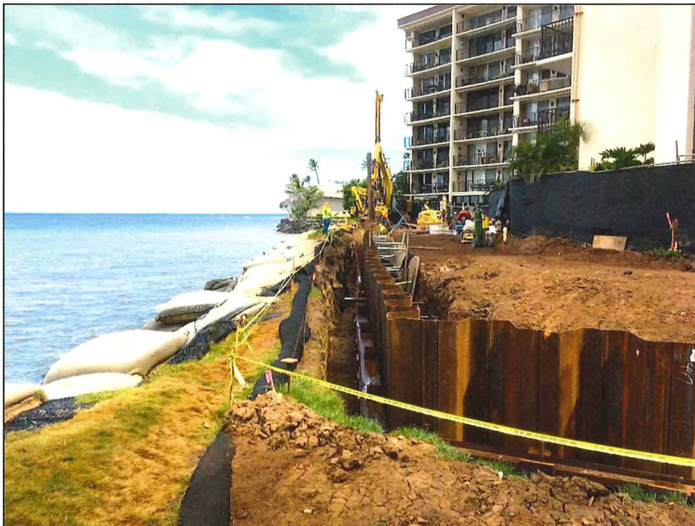
Figure 5-19 Example of a steel sheet pile wall with earth anchors (Kahana, Maui)
