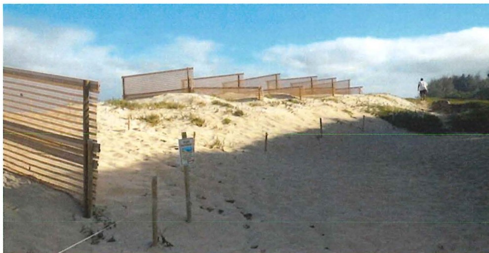
Figure 5-2 Sand fencing at Kanaha Beach, Maui
