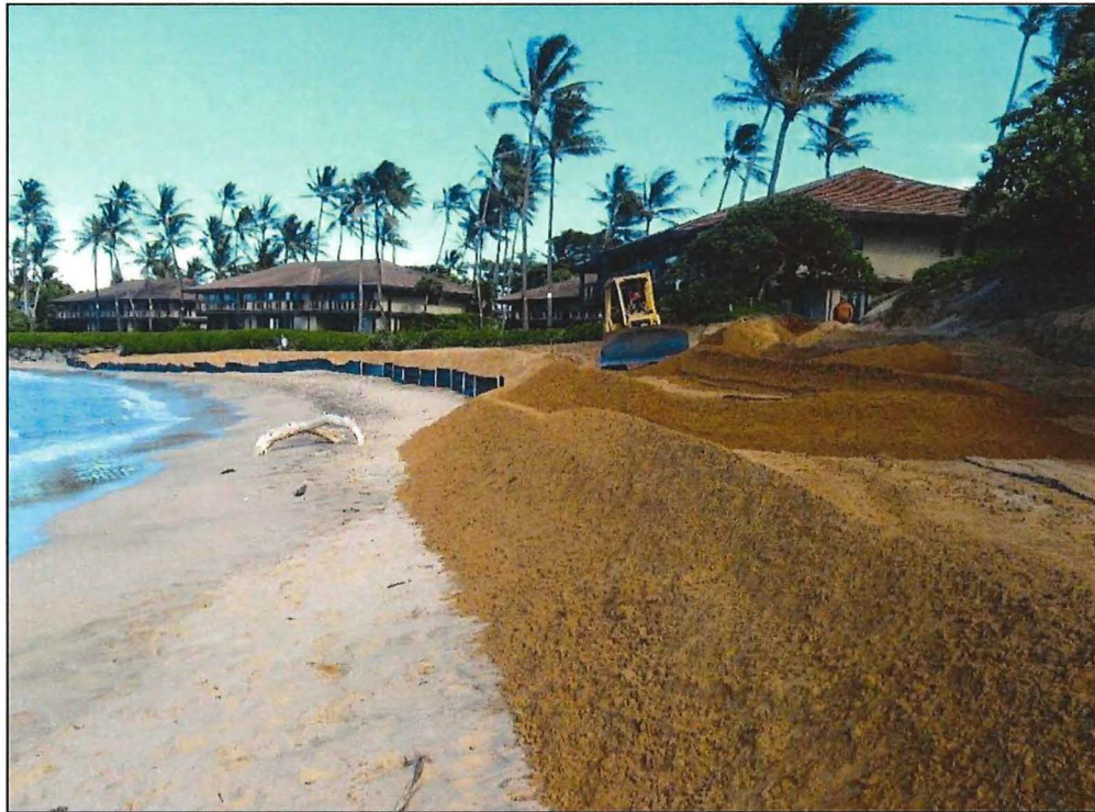
Figure 5-6 Small-scale beach nourishment at Paia, Maui (2016)
