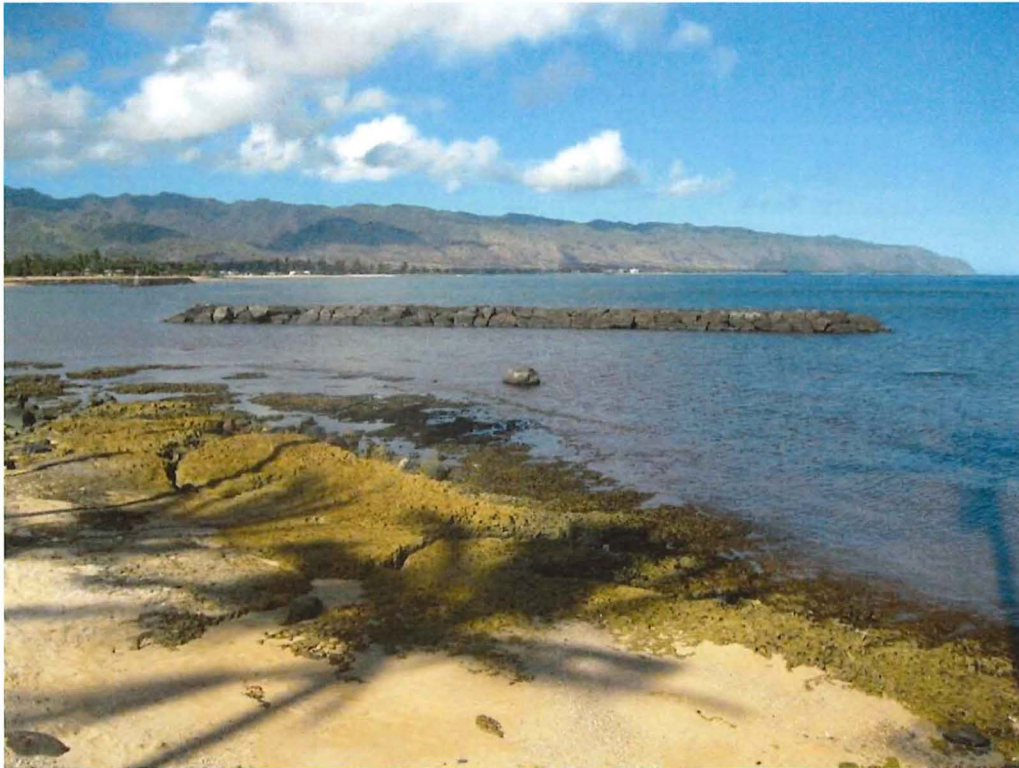
Figure 5-20. Offshore breakwater at Haleiwa Beach Park
