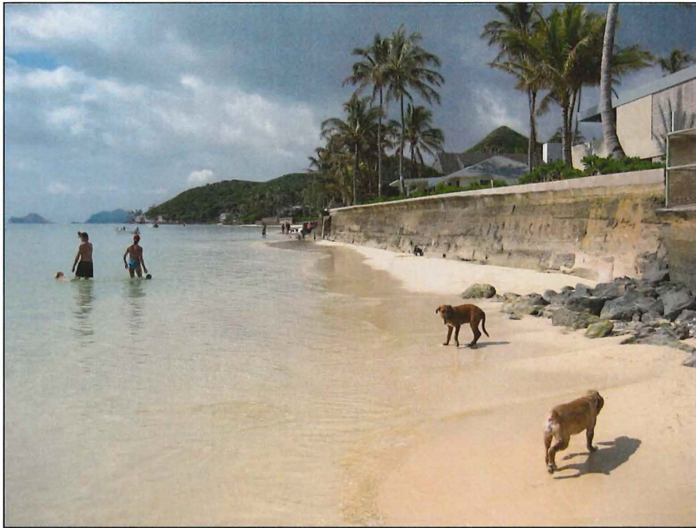
Figure 5-15 Typical concrete seawall providing hard shoreline protection
