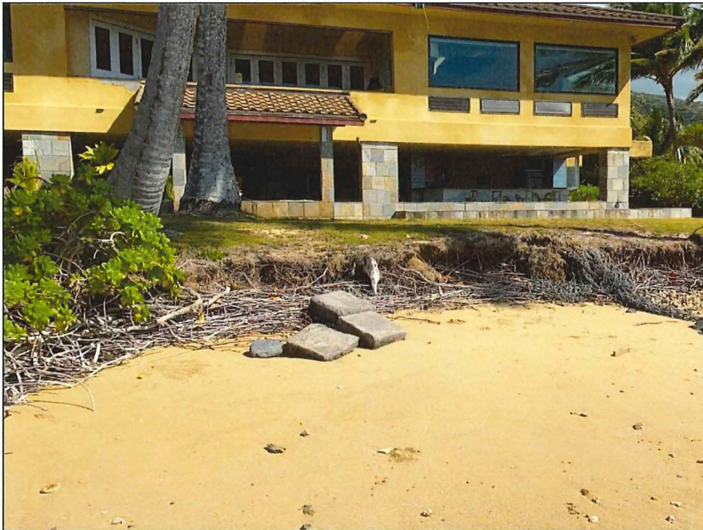
Figure 5-10 Example of vertical accommodation (freeboard) on Moloka'i
