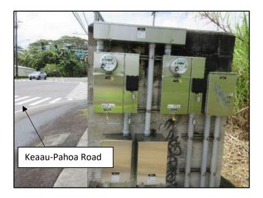
Photograph 13. A view of the back side of a concrete wall with street light and traffic sign meters as well as the HELCO gutter box and communication cabinet east of the subject property at parcel 007 (31 May 2023).
