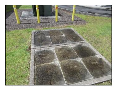
**Photograph 9.** A view of the cable manholes west of the pad-mounted transformer on the adjoining property, parcel 069. The concrete cap is stained due to rain/water and potential mildew (31 May 2023).
