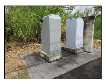
Photograph 12. A view of the Hawaii Electric Light Company (HELCO) street light and traffic signs closets east to parcel 007. The concrete pad is stained due to potential mildew (31 May 2023).
