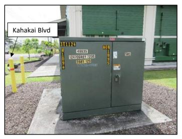
Photograph 8. A view of the padmounted transformer on the adjoining property (parcel 069) to the south of parcel 007. Stain on the concrete pad appears to be mildew (31 May 2023).
