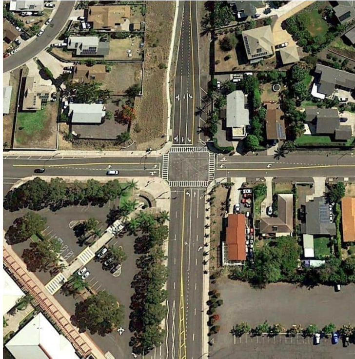
Figure 7 Aerial View of Paniolo Avenue and Ho'oko Street Intersection
