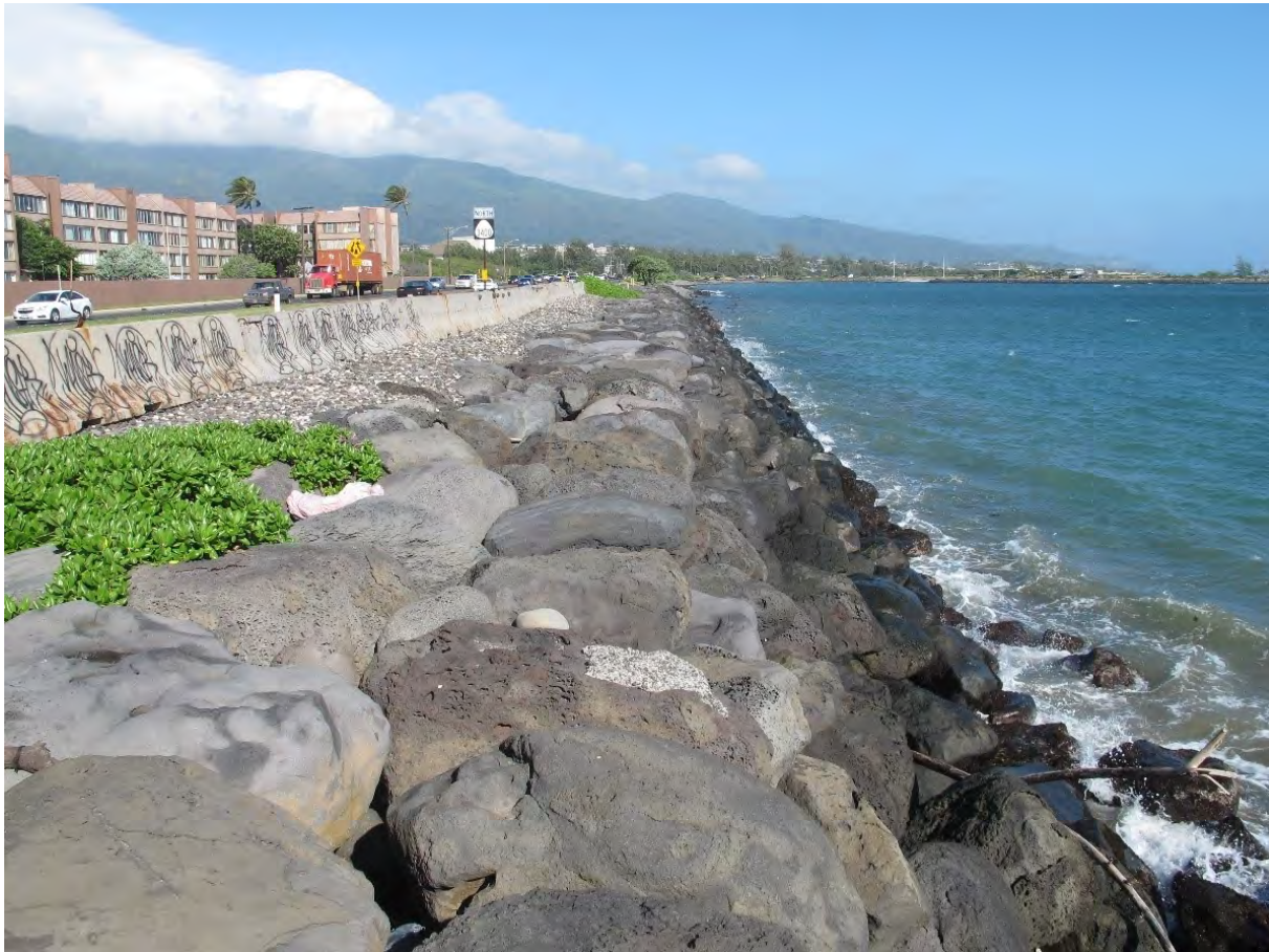
Figure 6-1. Example of rock (rubble mound) revetment, Kahului Harbor, Maui
