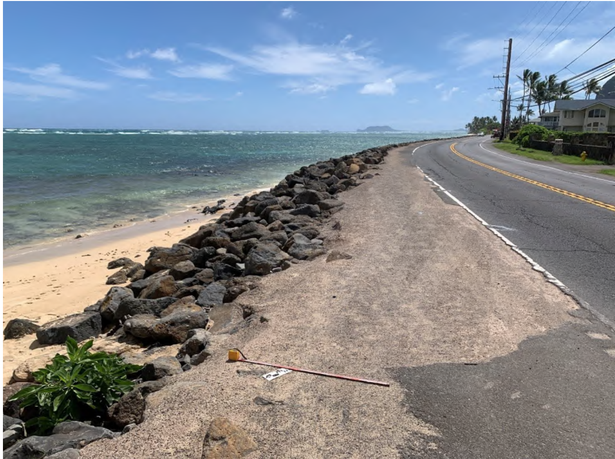
Figure 27. Northern end of section 5, Ka‘a‘awa Ahupua‘a, at the southern end of several residential structures just south of Swanzy Beach Park; view southeast
