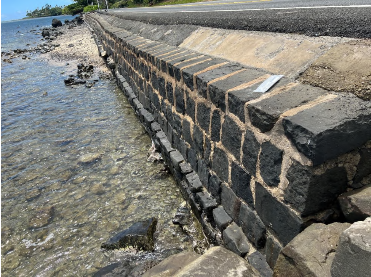
Figure 44. View of mortared rock wall (SIHP # 50-80-06-7922) dating from the original construction of the Kamehameha Highway in the late 1920s along the makai shoulder of the highway in section 4; facing south
