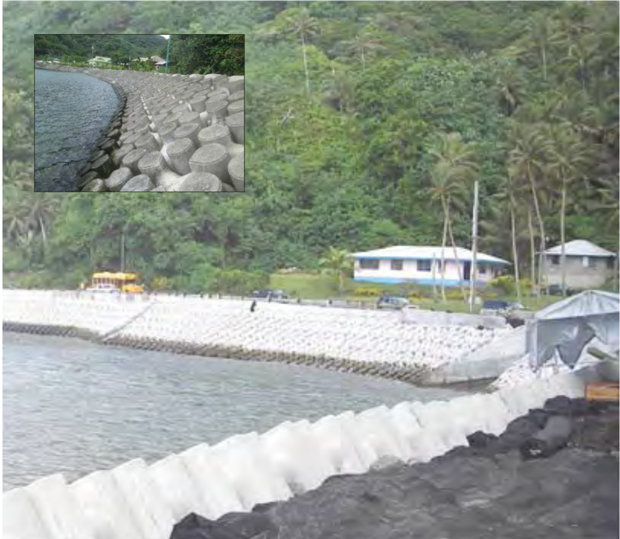
Figure 7-15. Example tribar installation, American Samoa
