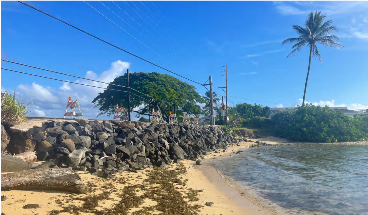
Figure 2-3. Kualoa Park (North) project site and riprap emergency protection, shoreline receding from right to left
