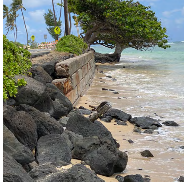
Figure 2-14. Scattered and displaced riprap and concrete piles, looking south ( left ) and pile seawall ( right )
