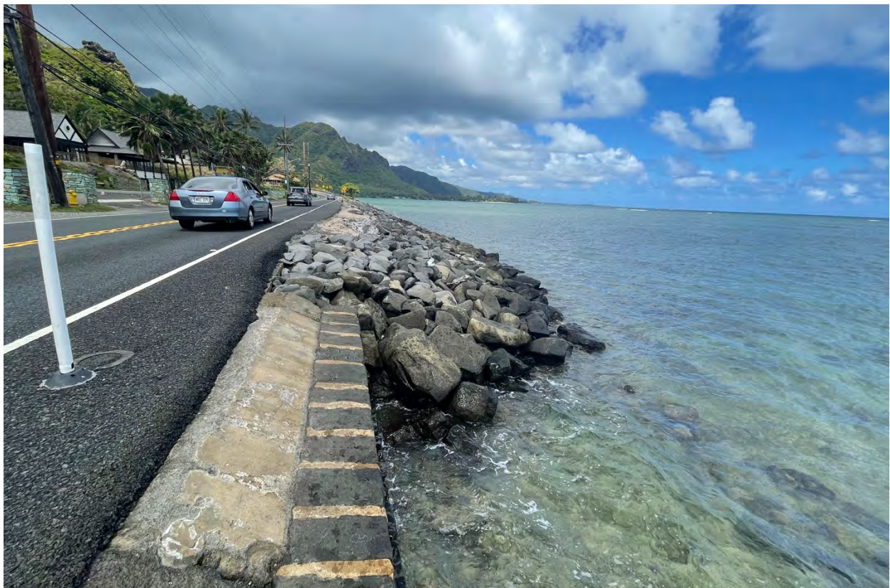
Figure 2-23. North end of Crouching Lion project site, Kahana Bay in background
