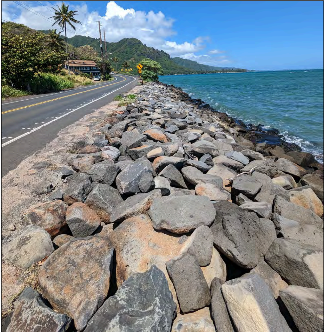
Figure 2-1. Example of an engineered, uncemented revetment near Crouching Lion.
