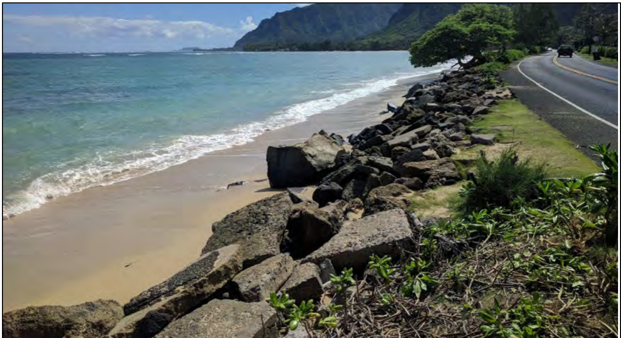
Figure 1-15. Stone and concrete riprap along the Punalu'u South Project Site.
