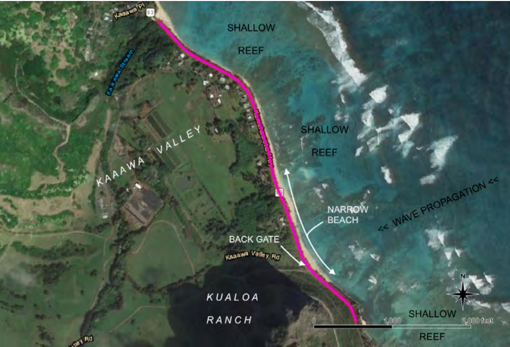
Figure 2-7. Kaaawa Stream to Kaaawa Beach Park repair site (credit: background map Google Earth)
