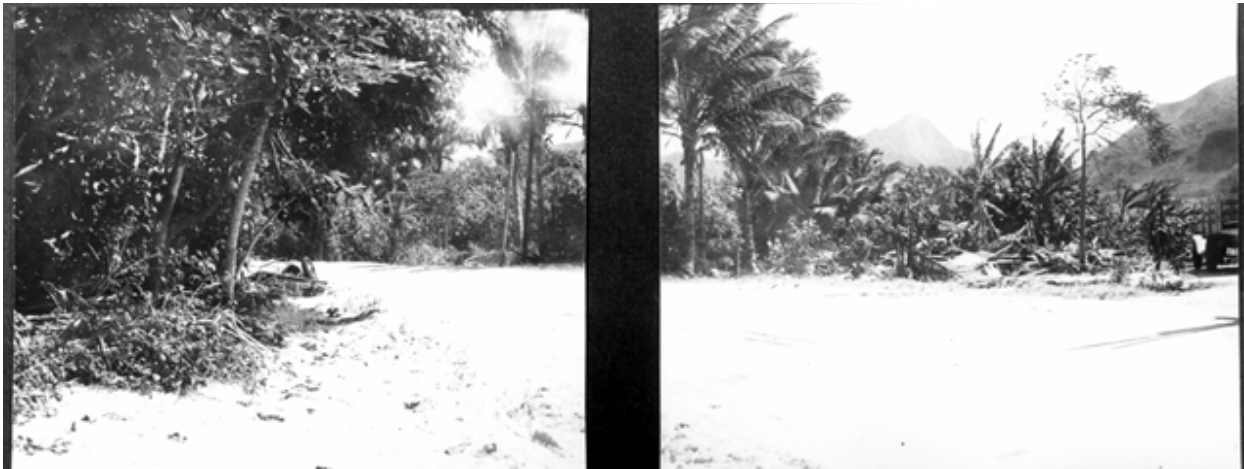
Figure 1-8. Kamehameha Hwy in Punaluu, following 1946 tsunami.
