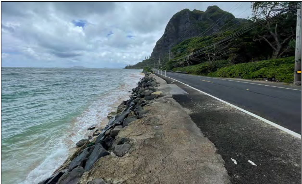
Figure 1-9. Central stretch of the Ka'a'awa Valley Project Site.
