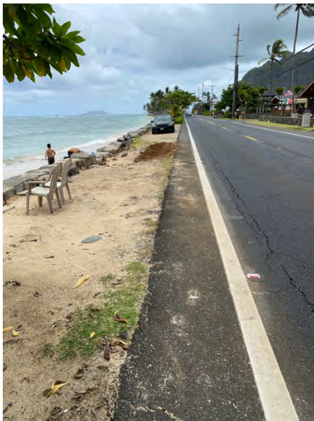
Figure 2-18. Stacked concrete block seawall, looking south ( left ) and northern pocket beach ( right )
