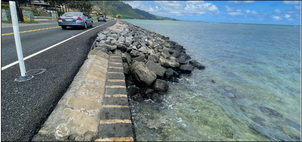
Figure 1-14. Absence of beach material, seawall, and non-engineered riprap along the northern section of the Crouching Lion Project Site followed by discontinuous non-engineered riprap.
