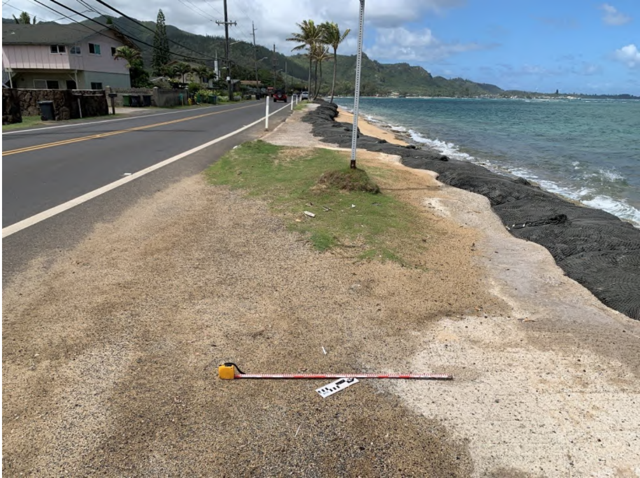
Figure 19. Middle of section 1, near the boundary of Mākao and Kapaka ahupua‘a, just south of Makao Road; view northwest
