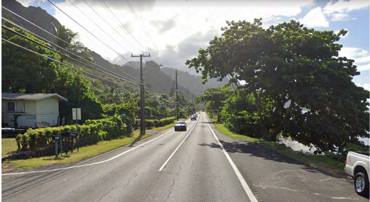
Figure 2-21. Highway shoulder condition in vicinity of photographs shown in Figure 2-20
