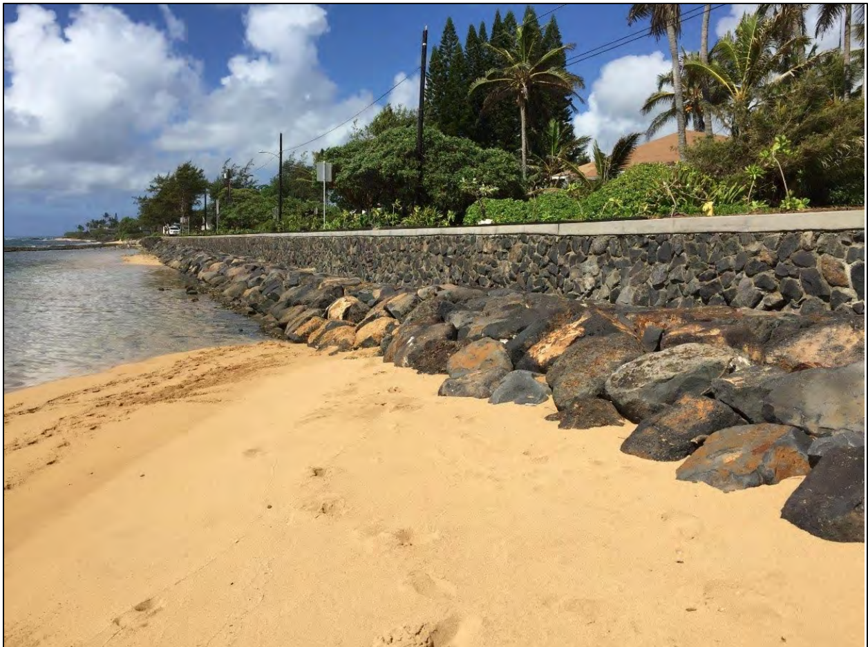
Figure 2-3. Example hybrid seawall with rock apron in Kapa'a, Kauai.
